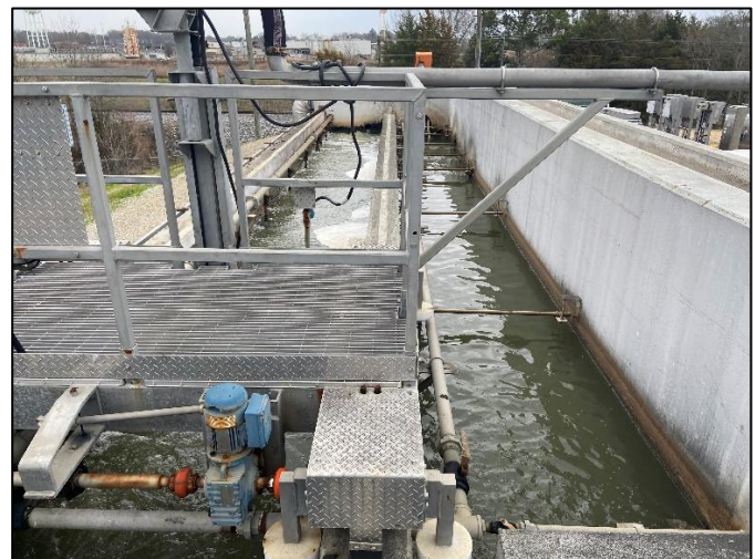
Photo 6: Headworks (grit chamber on left).
