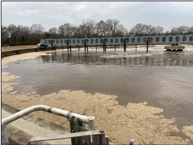
Photo 1: Circular traveling bridge aeration basin.
