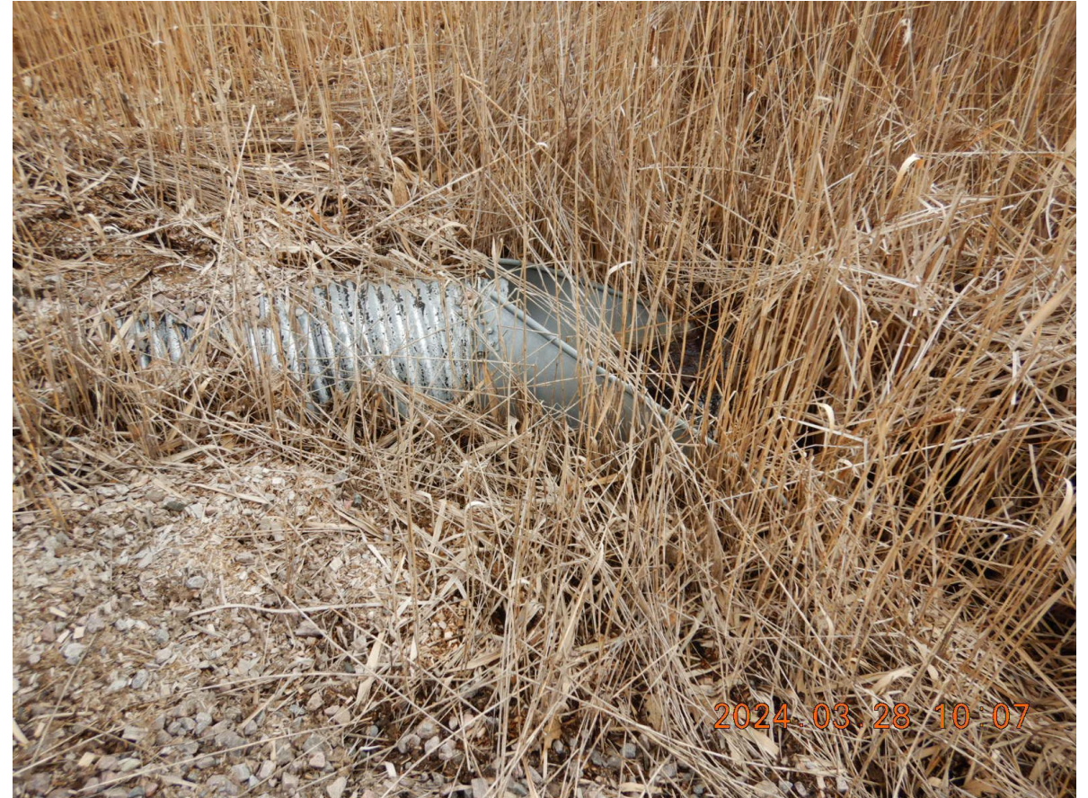
DSCN2691 - Outlet pipe of W corner and continues under gravel road to railroad property
