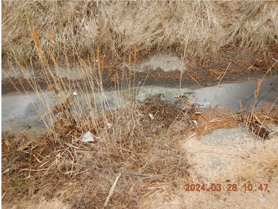
DSCN2755 - Channel with water from outlet near Catch Basin #3
