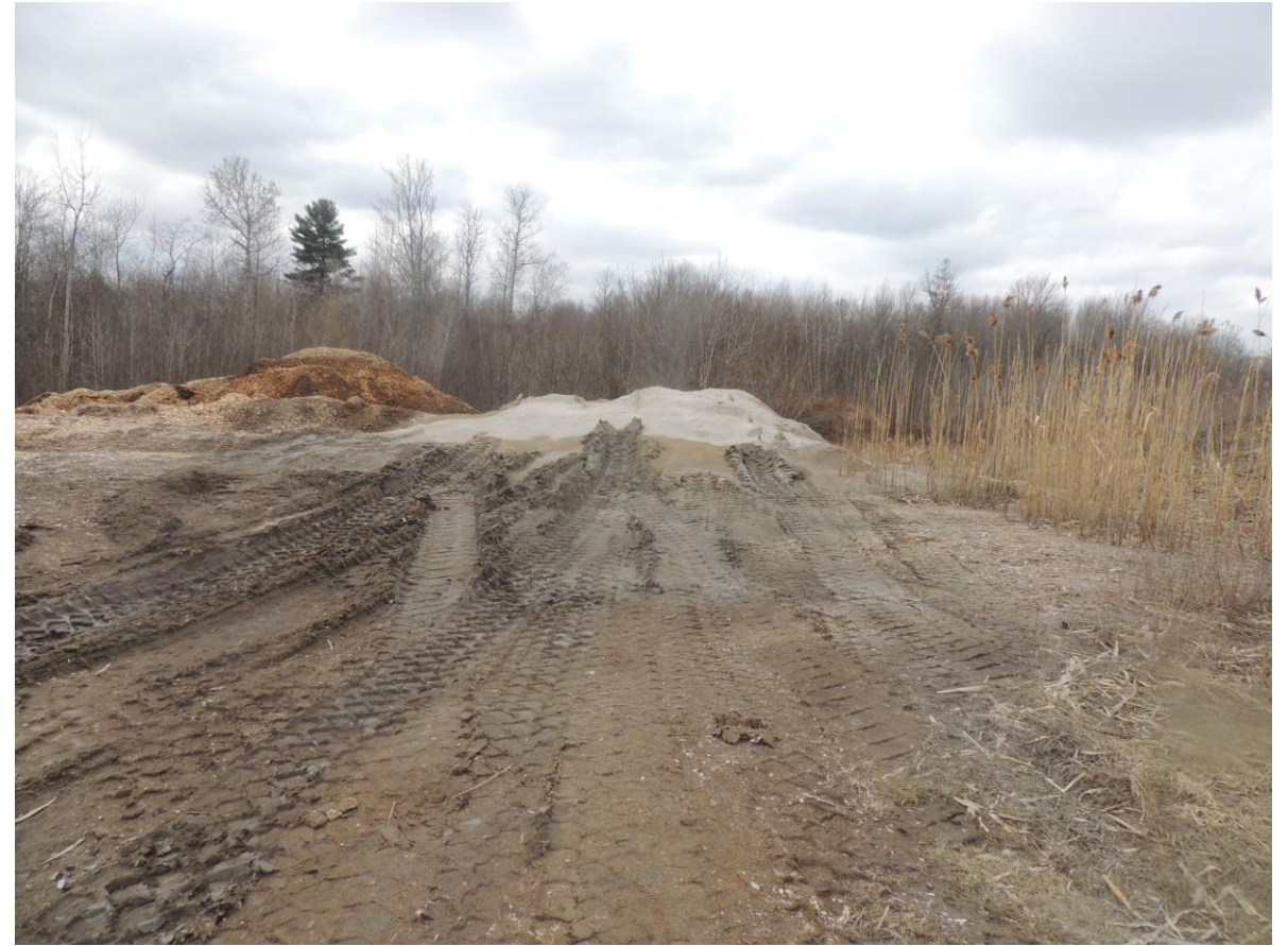
DSCN4046 – Boiler ash storage pile (uncovered), no BMPs in place
