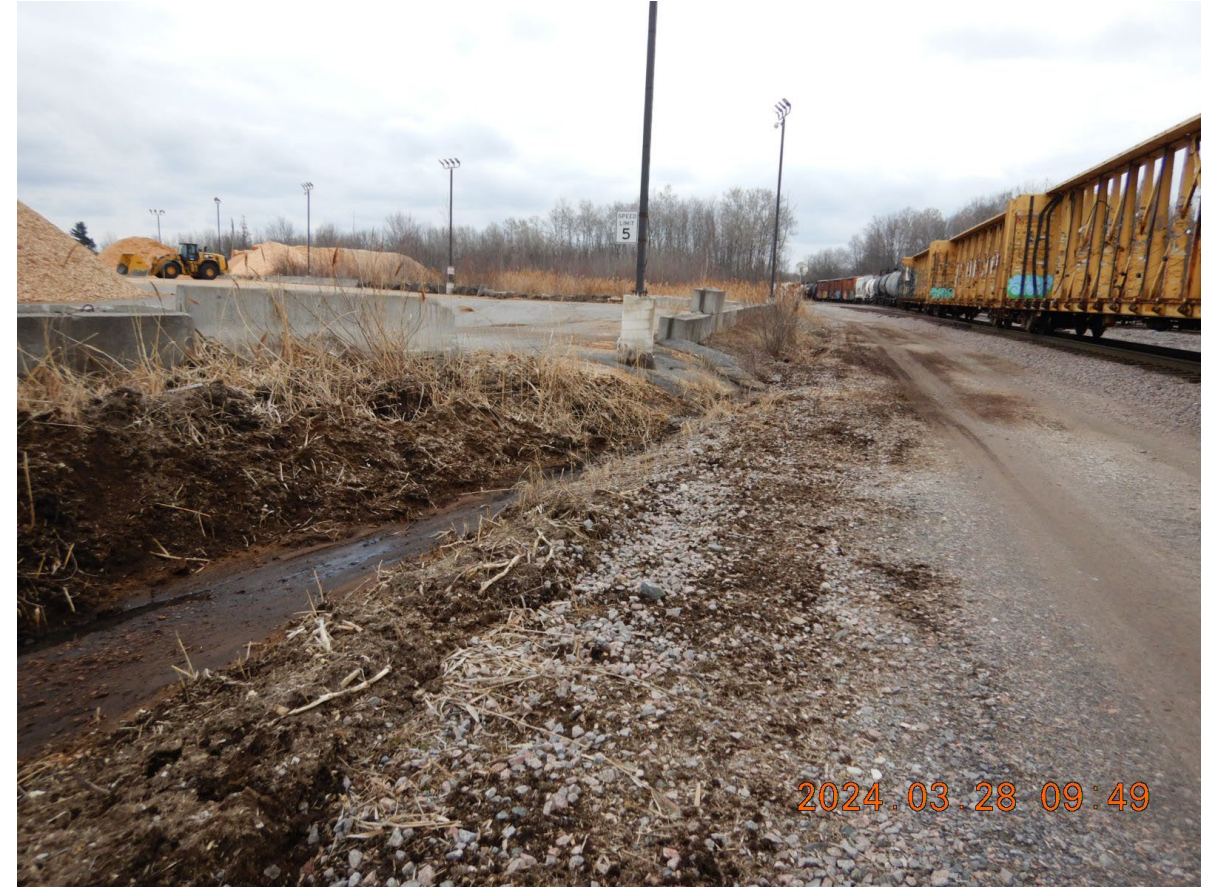
DSCN2672 - SW view of stormwater runoff from W edge of Site along CSX Rail Line
