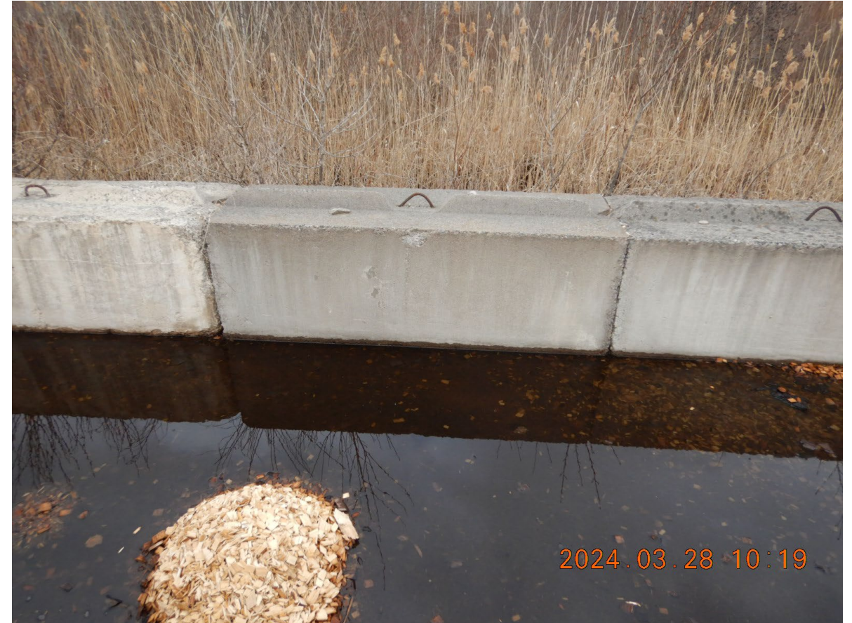
DSCN2716 - Stormwater runoff on S lot of Site
