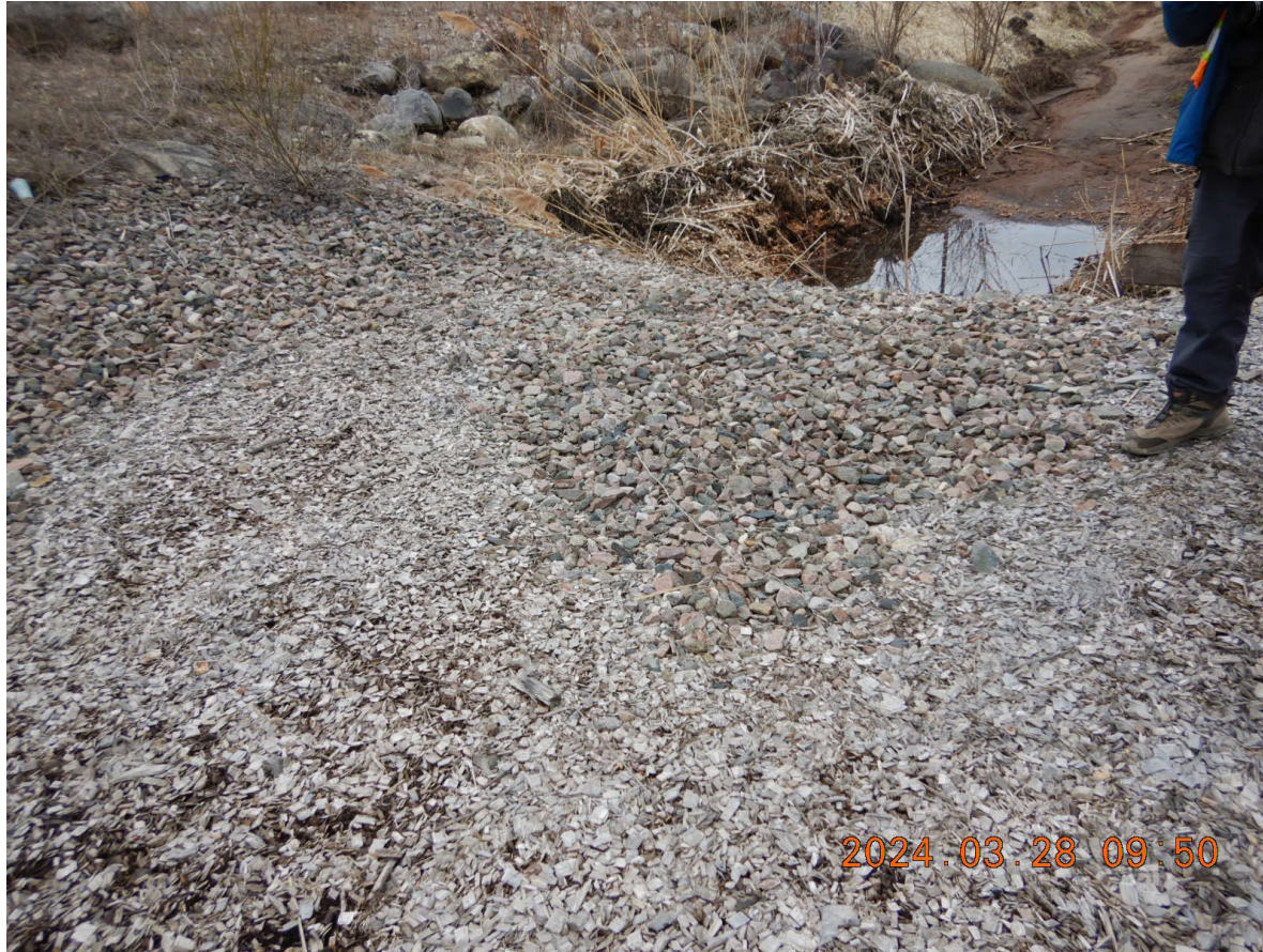
DSCN2675 - Gravel drive over stormwater runoff area connecting railroad area to loading parking lot on W side of Site
