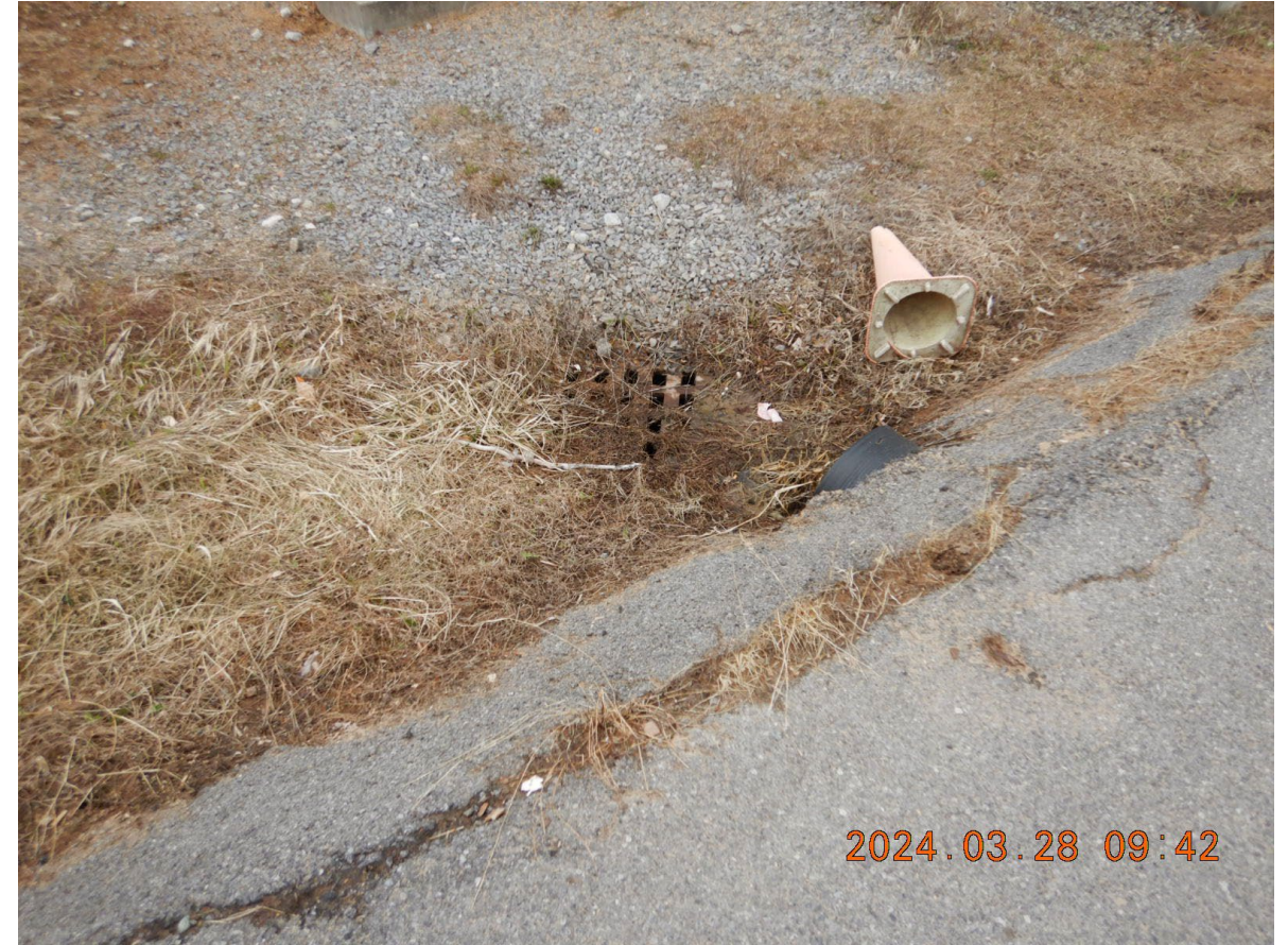
DSCN2662 - Stormwater Catch Basin #1 near the S corner of the packaging warehouse building that leads to W edge of Site
