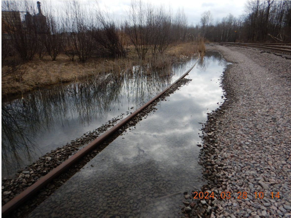
DSCN2699 - Stormwater runoff on SW side of Site
