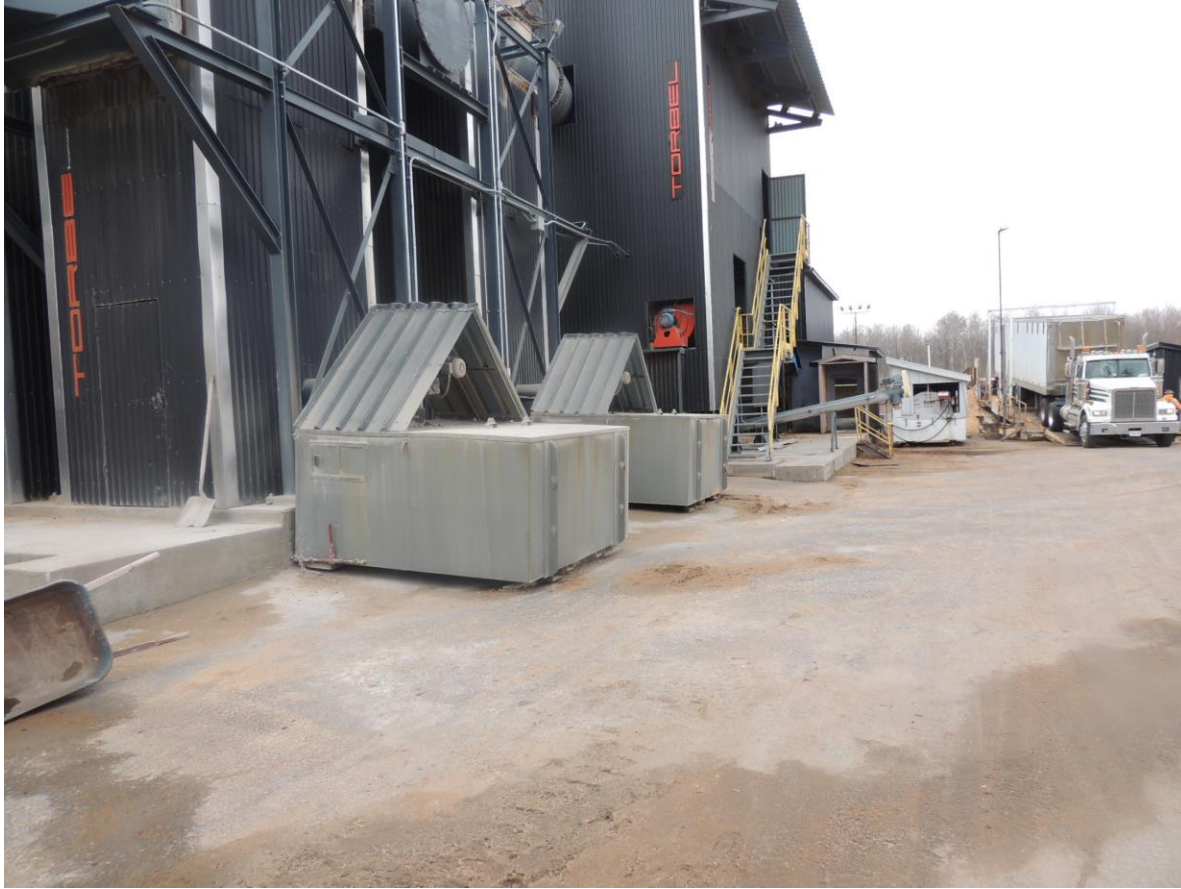
DSCN4043 – Waste ash dumpsters
