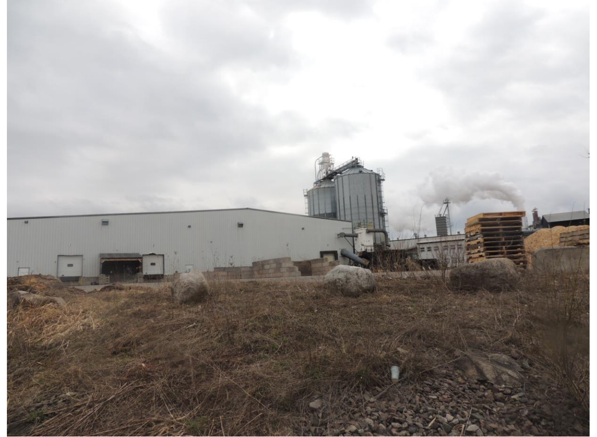
DSCN4001 – Western portion of Site, with slope down to stormwater channel/retention pond along railway
