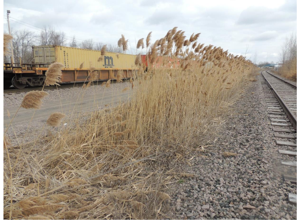
DSCN4009 swale along railway (west of northern portion of Curran Site)
