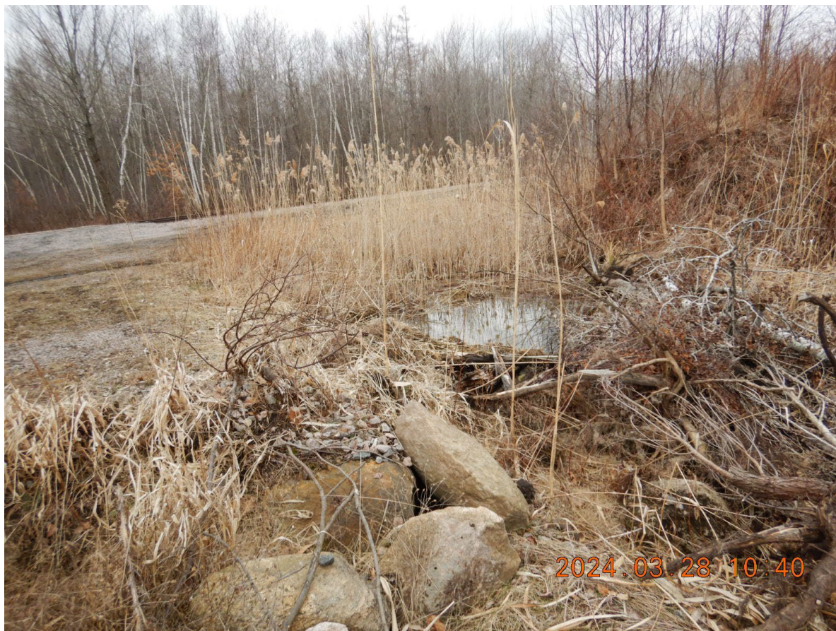
DSCN2745 - Stormwater drainage downhill of pellet ash stockpile area
