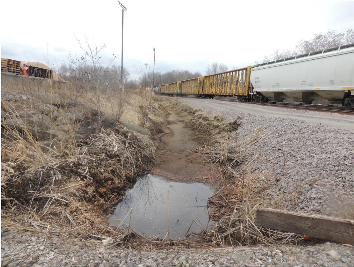
DSCN4002 – Stormwater channel, with water in it that is said to flow under the gravel roadway
