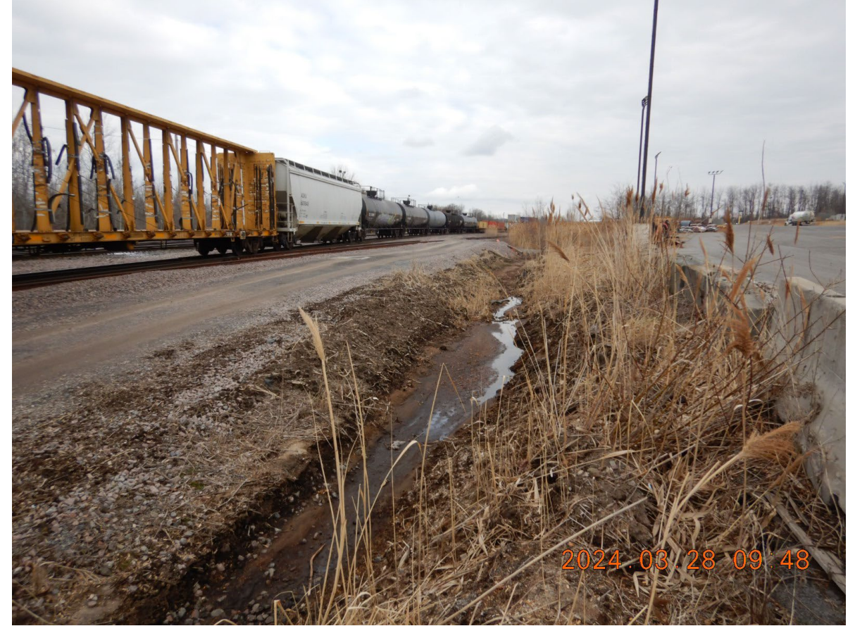
DSCN2669 - Stormwater channel with water in it along CSX rail line on western side of Site
