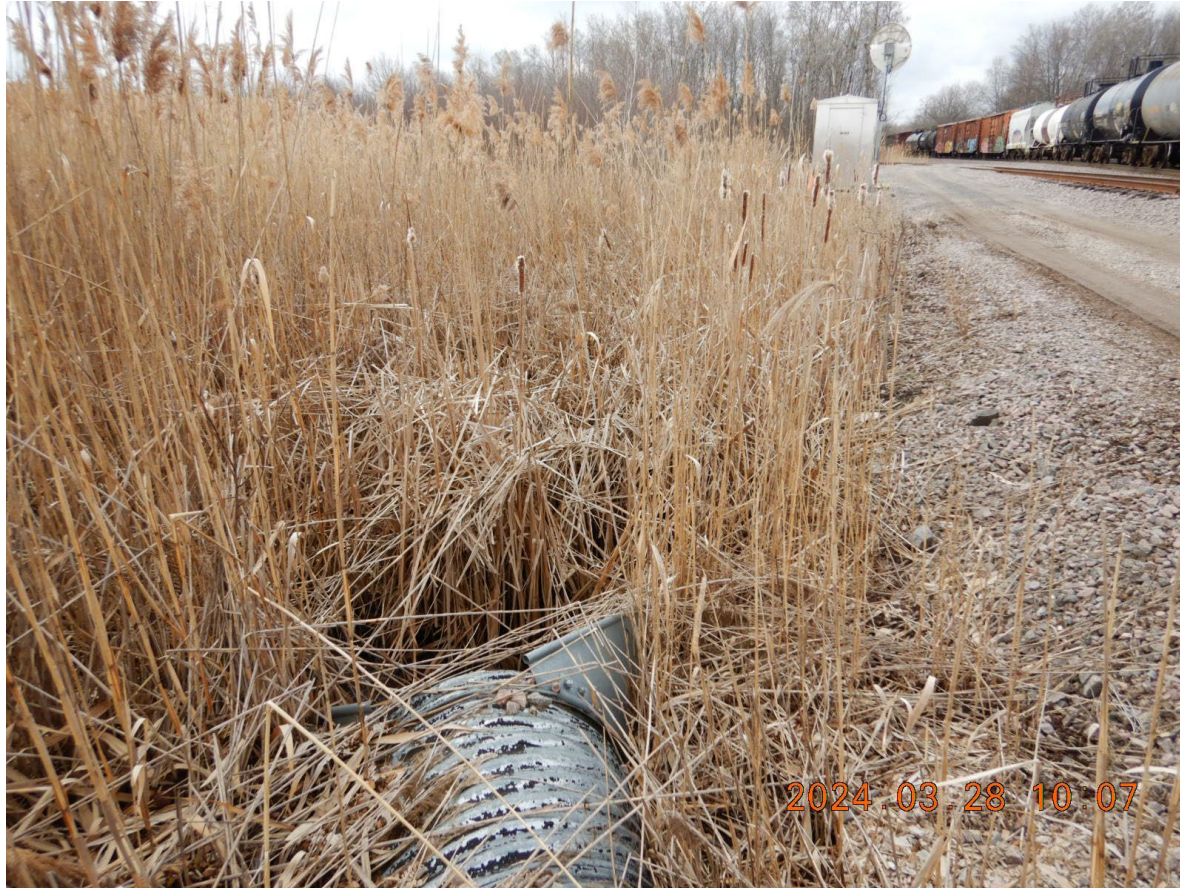
DSCN2693 - Outlet pipe of W corner and continues under gravel road to railroad property
