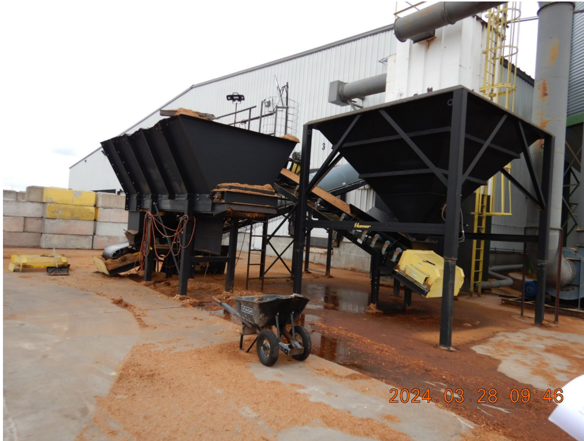
DSCN2666 - Mulch loading area located on the SW corner of the packaging warehouse
