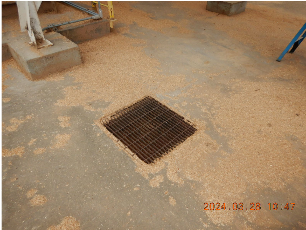
DSCN2753 - Catch basin #3 on S corner pellet manufacturing building
