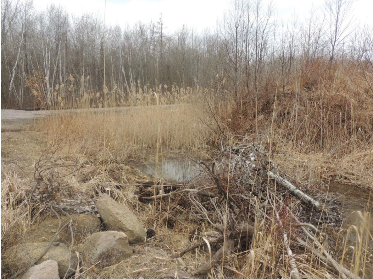
DSCN4056 - Drainage between rail line and southern portion of Facility
