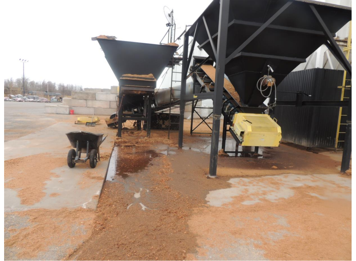
DSCN3991 – Puddles of water in and around material from mulch loading area/package warehouse and exposed mulch material
