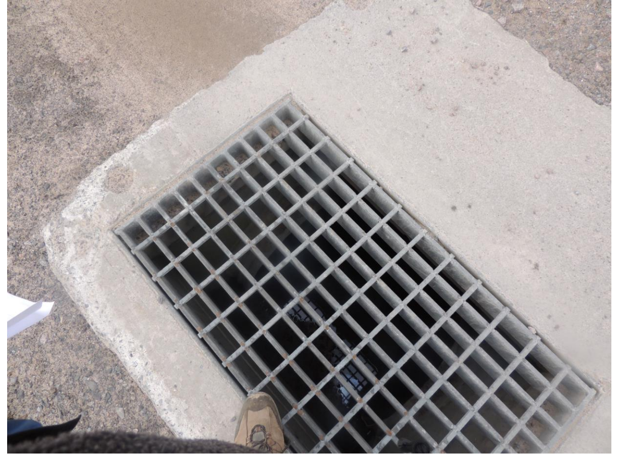
DSCN4013 – Stormwater catch basin along railroad tracks on western portion of the Site
