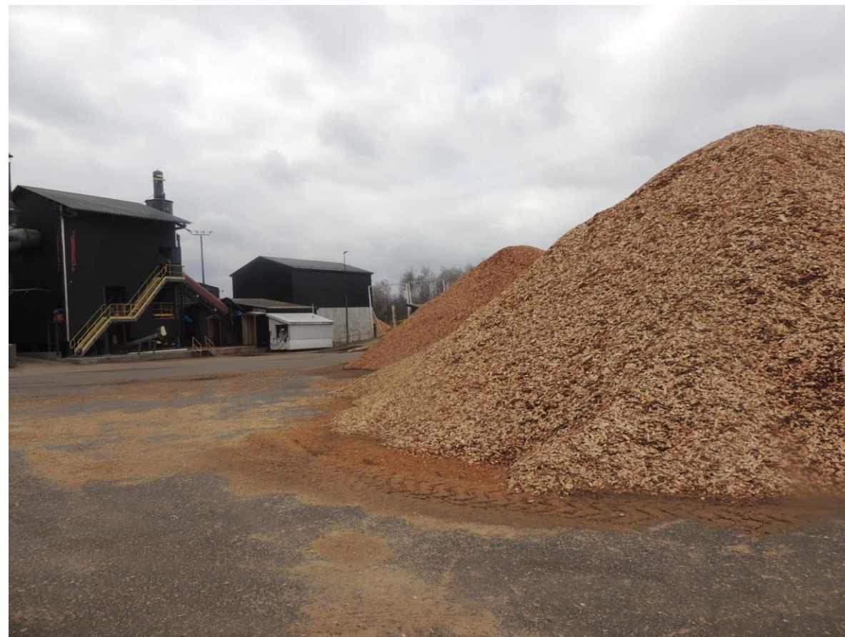
DSCN3993 – Exposed woodchip storage piles
