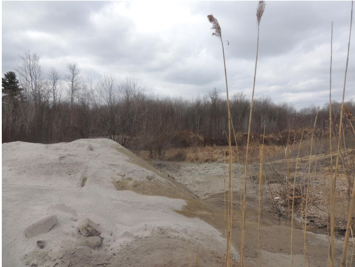
DSCN4047 – Boiler ash storage pile (uncovered), no BMPs in place
