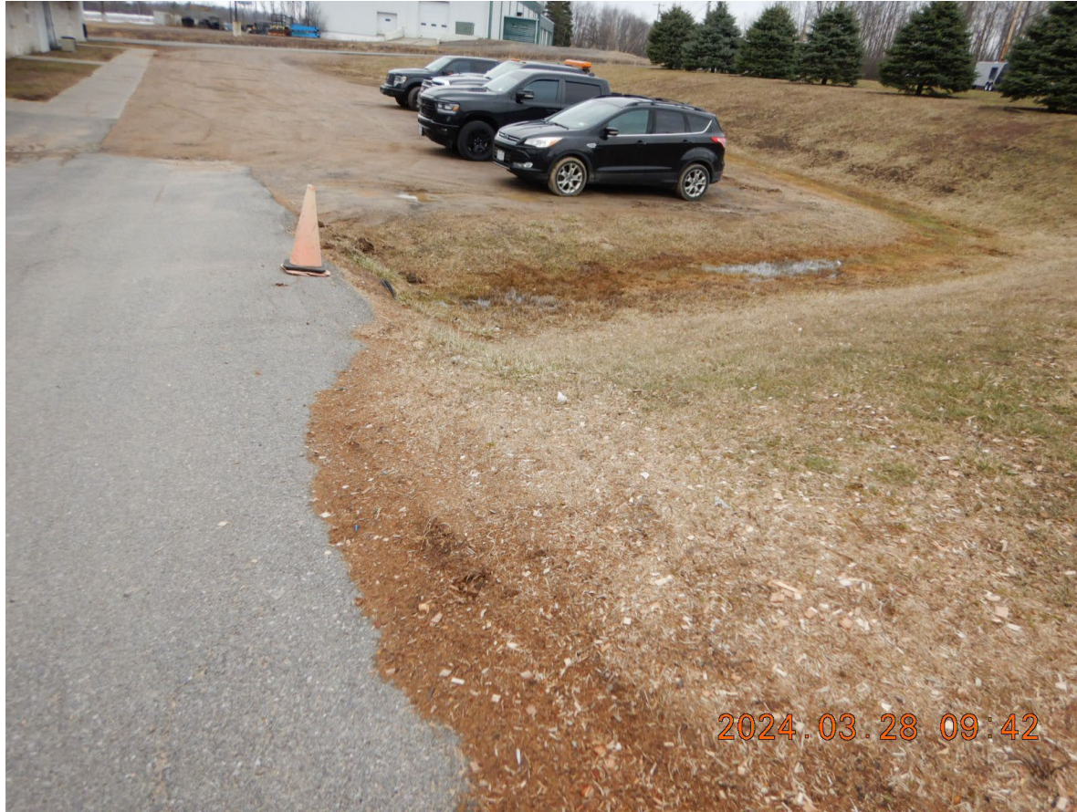
DSCN2661 - Stormwater channel that enters a pipe and flows downslope W towards storm drainage along rail line
