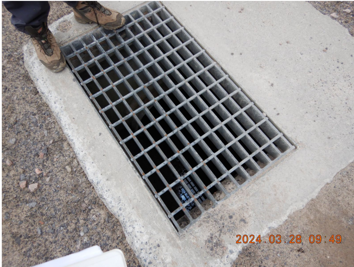
DSCN2673 - Catch Basin #2 located on what appears to be railroad property on W edge of Site, stormwater piping seen in the storm sewer
