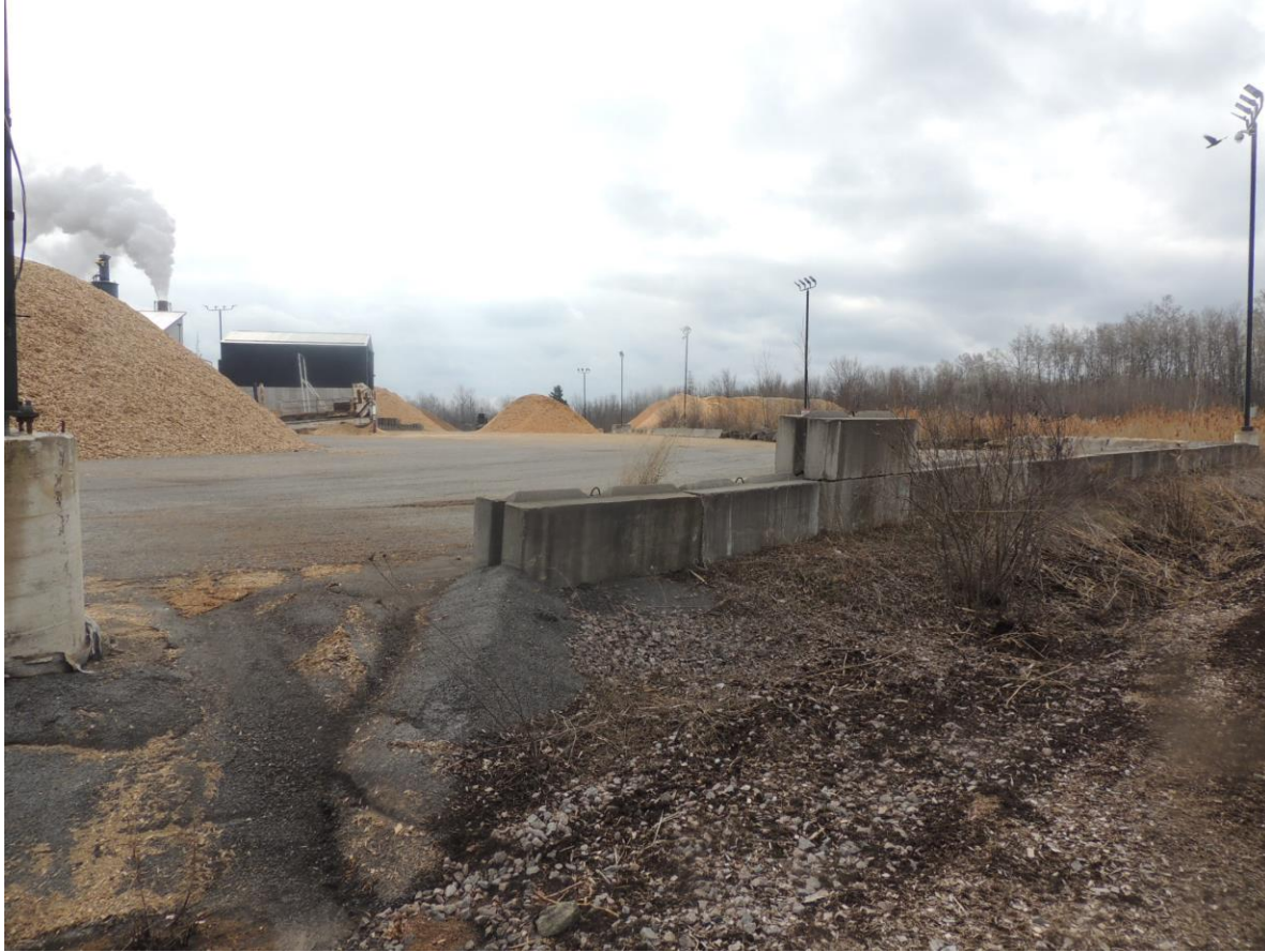
DSCN4014 – Area along western portion of the Site where stormwater can flow into channel between the Site and the CSX rail
