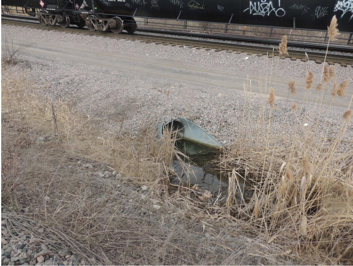
DSCN4008 – Pipe and channel with water adjacent to northwestern portion Curran Site next to CSX rail line
