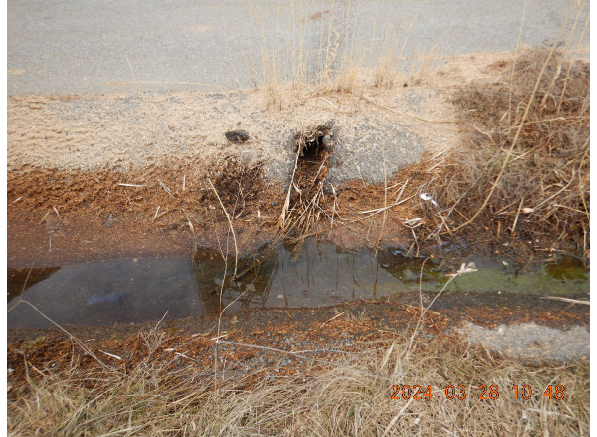
DSCN2756 - Stormwater outfall into channel near Catch Basin #3
