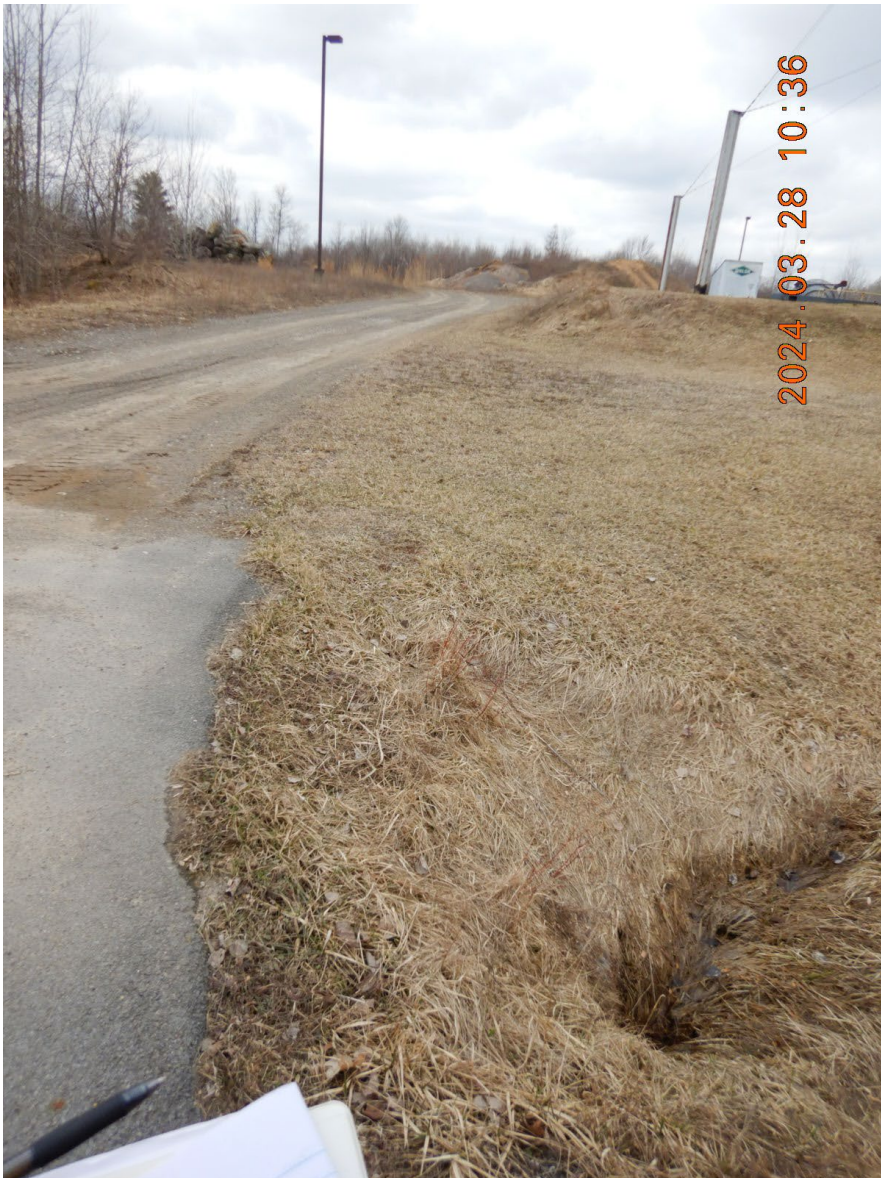
DSCN2728 - Stormwater drainage along Trade Drive
