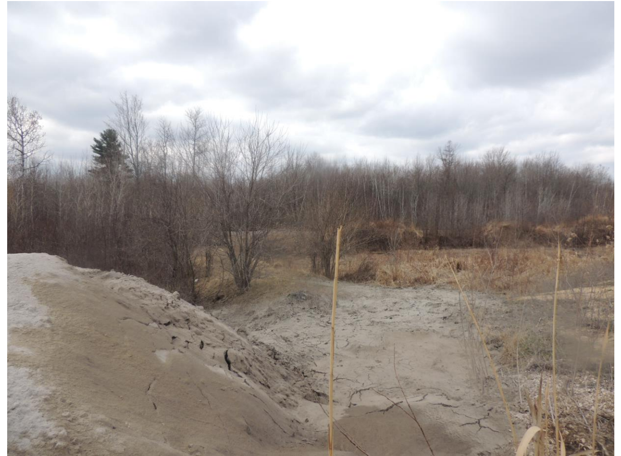
DSCN4048 – Boiler ash storage pile (uncovered), no BMPs in place
