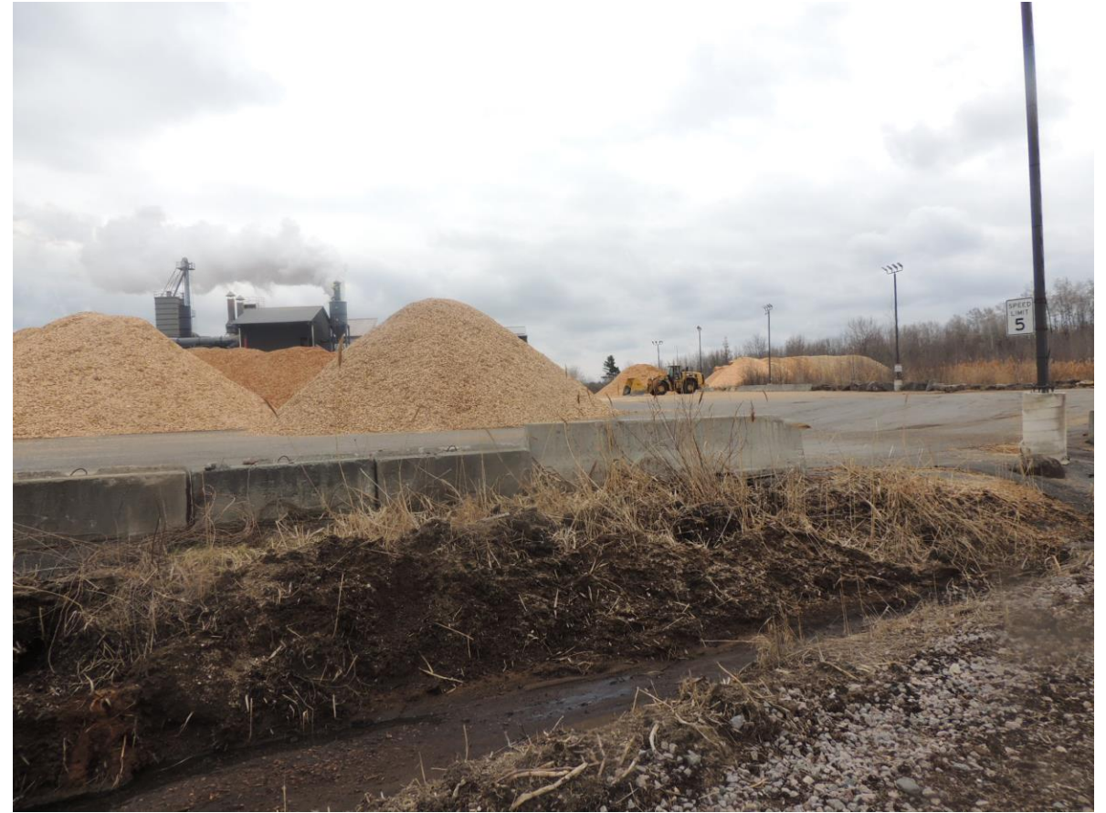
DSCN3997 – Exposed woodchip piles seen in the western portion of Site and the storm drainage channel seen in the foreground along the CSX rail. There is a gap in the concrete block wall on the right that allows stormwater to flow swales near CSX tracks.
