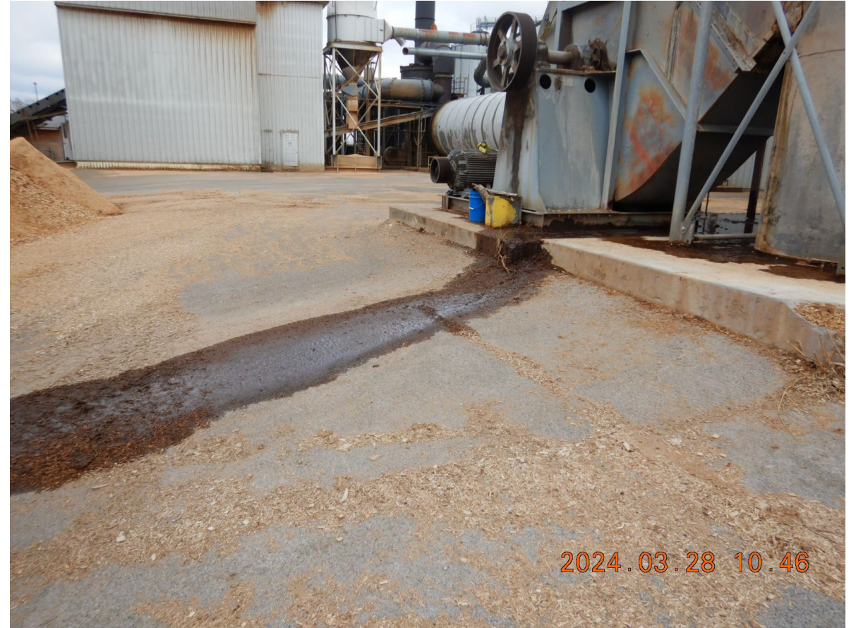
DSCN2748 - Condensate from manufacturing process
