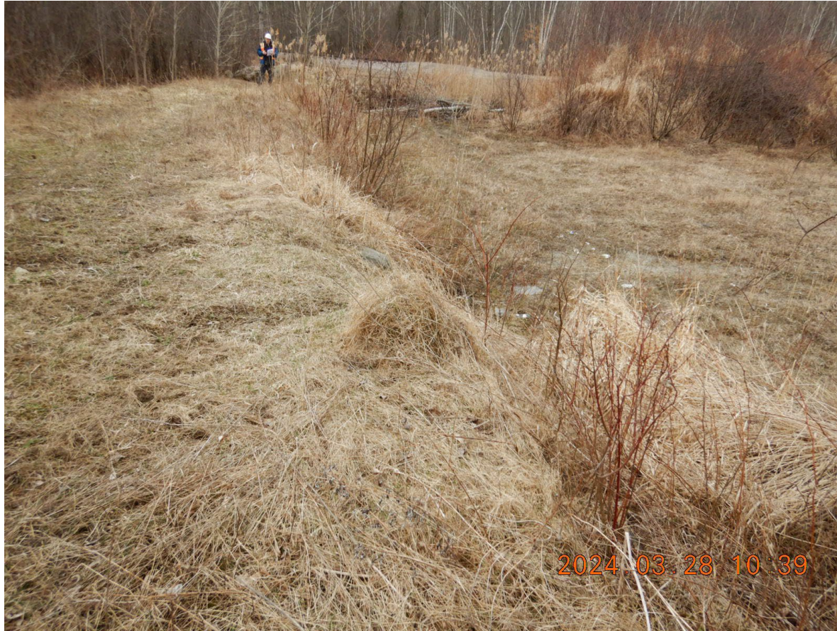
DSCN2741 - Stormwater drainage near pellet ash collection area
