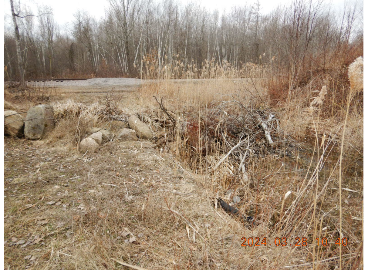
DSCN2744 - Stormwater drainage near pellet ash collection area
