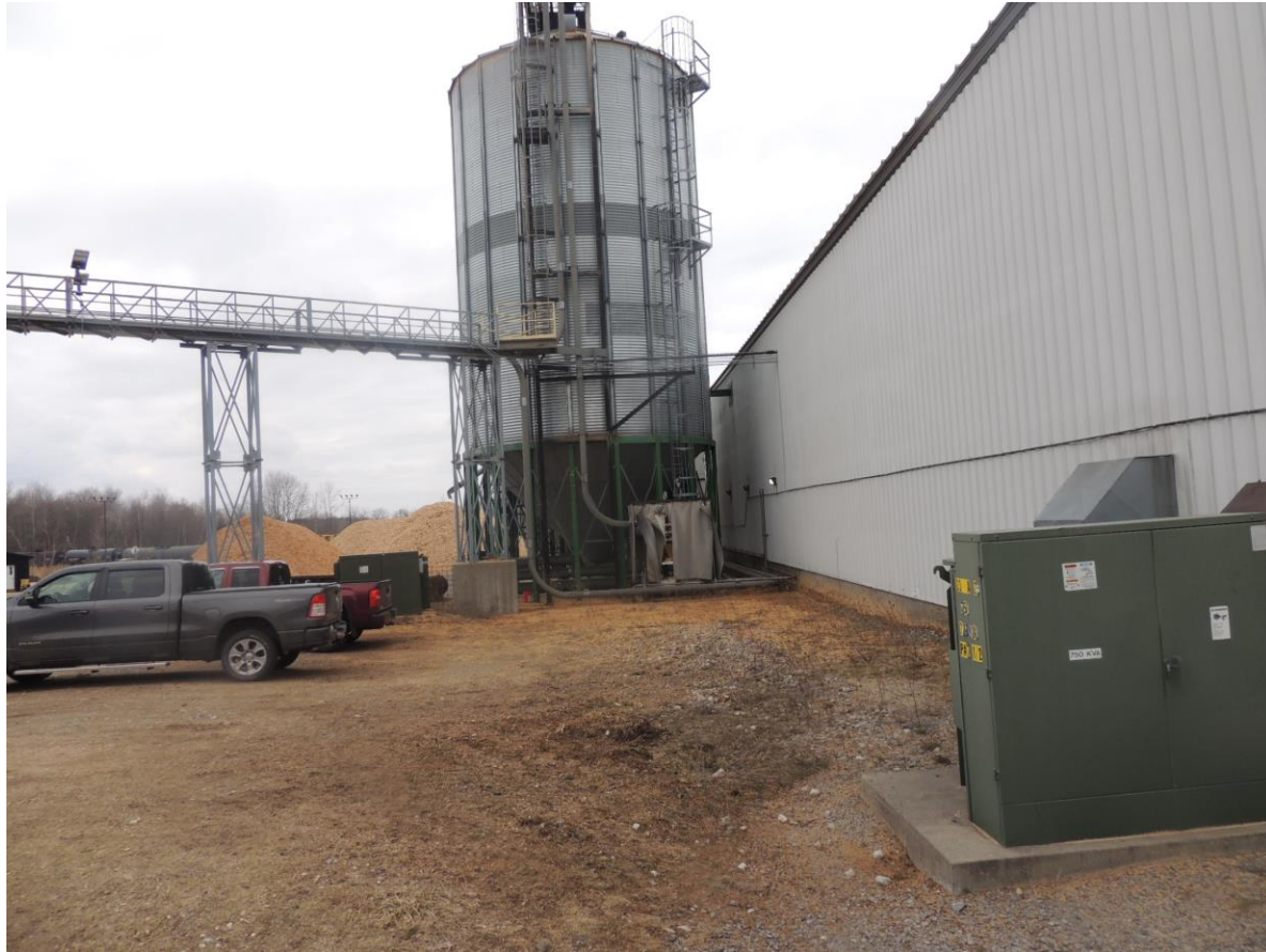
DSCN3988 – Pellet Silo – filled via vacuum system
