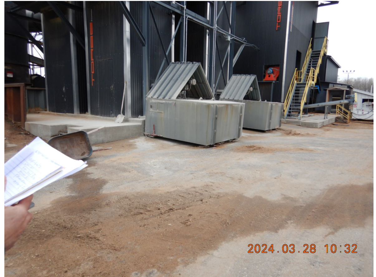
DSCN2724 - Two containers that collect waste ash during pellet manufacturing with loose material seen on the ground near them
