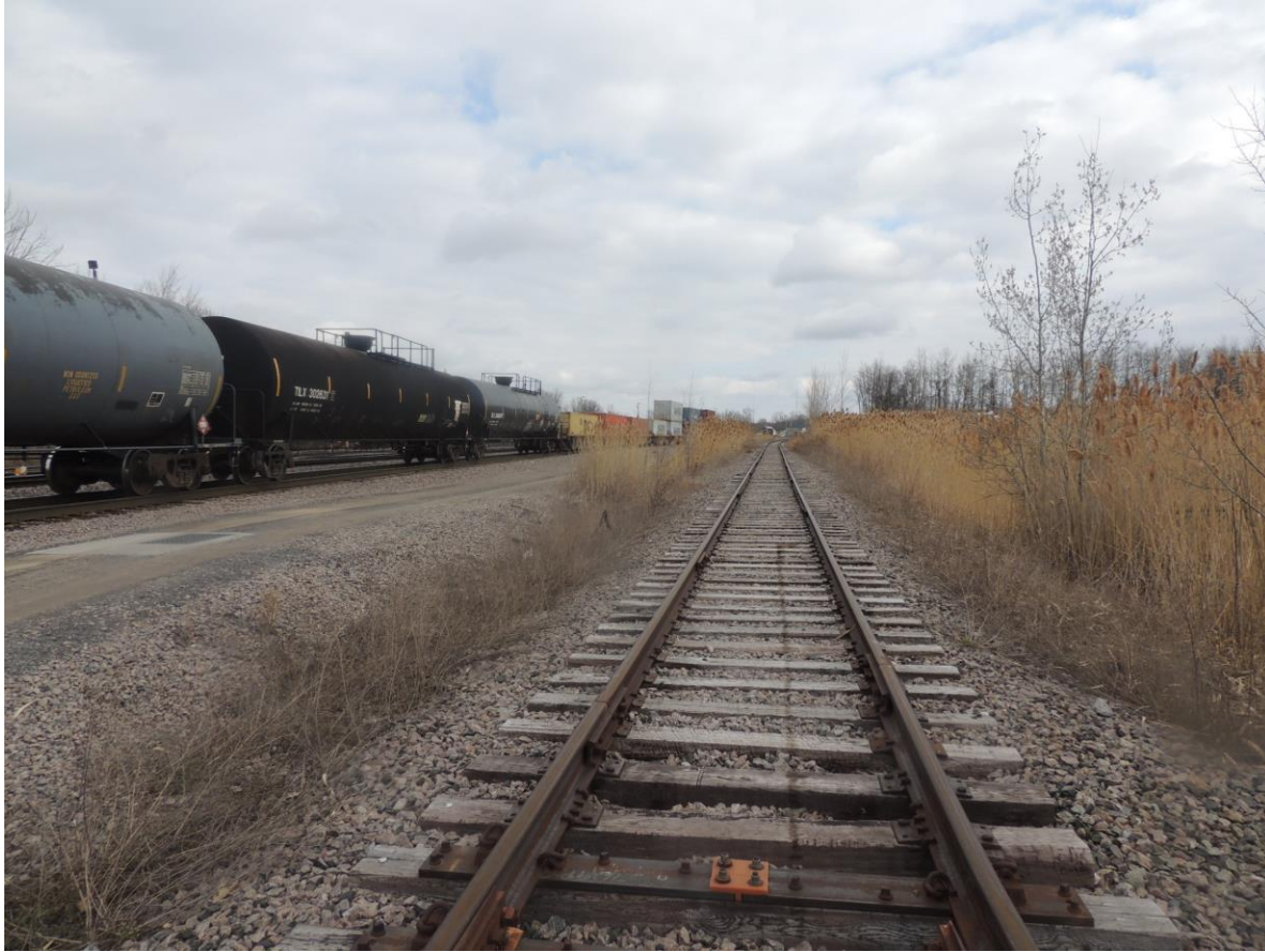
DSCN4012 - CSX tracks on the west side of the Curran property, stormwater inlet seen in left side of the photo near tank car
