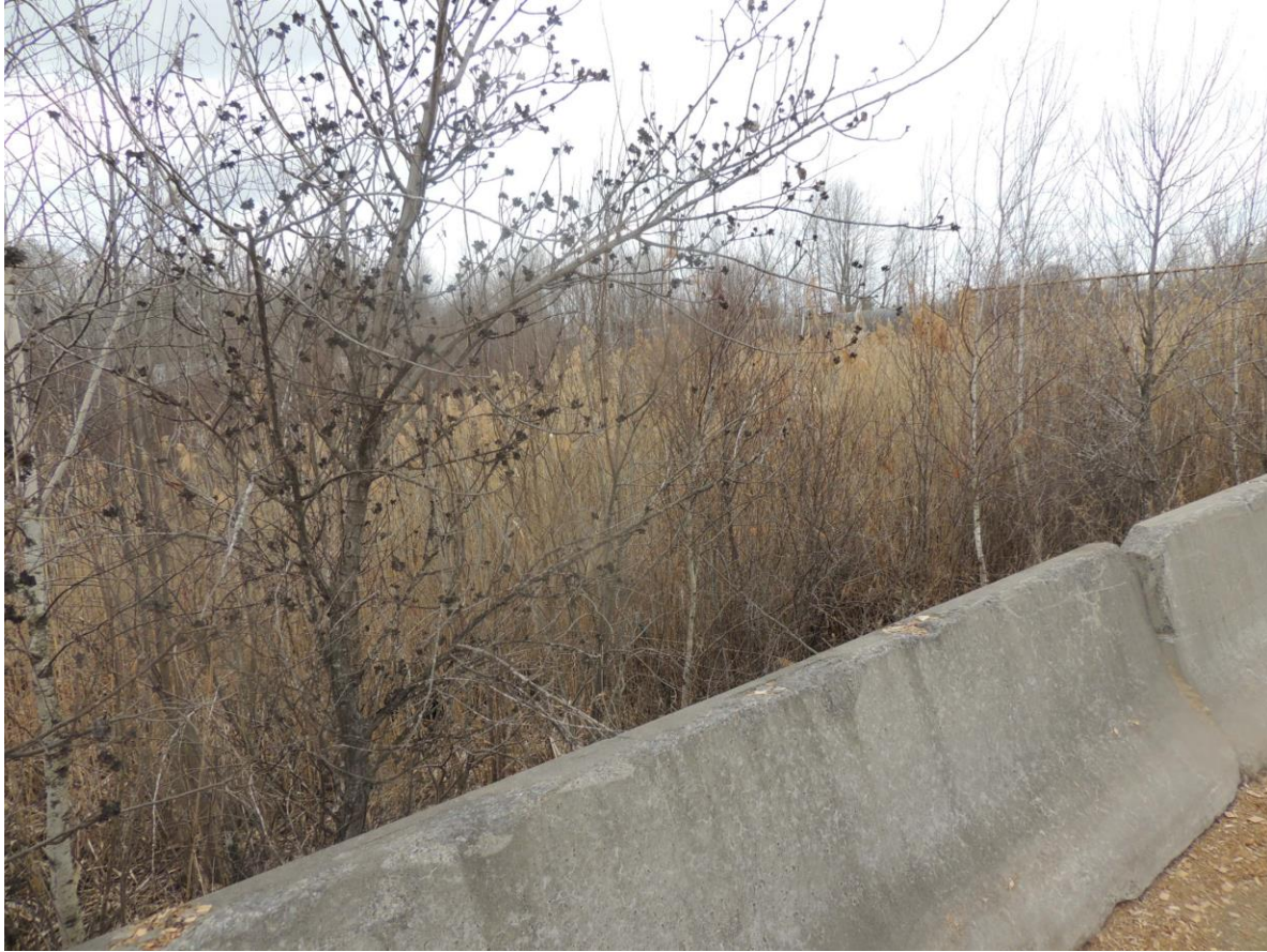
DSCN4034 - Exposed woodchips in the southwest portion of the Site with drainage downslope from it
