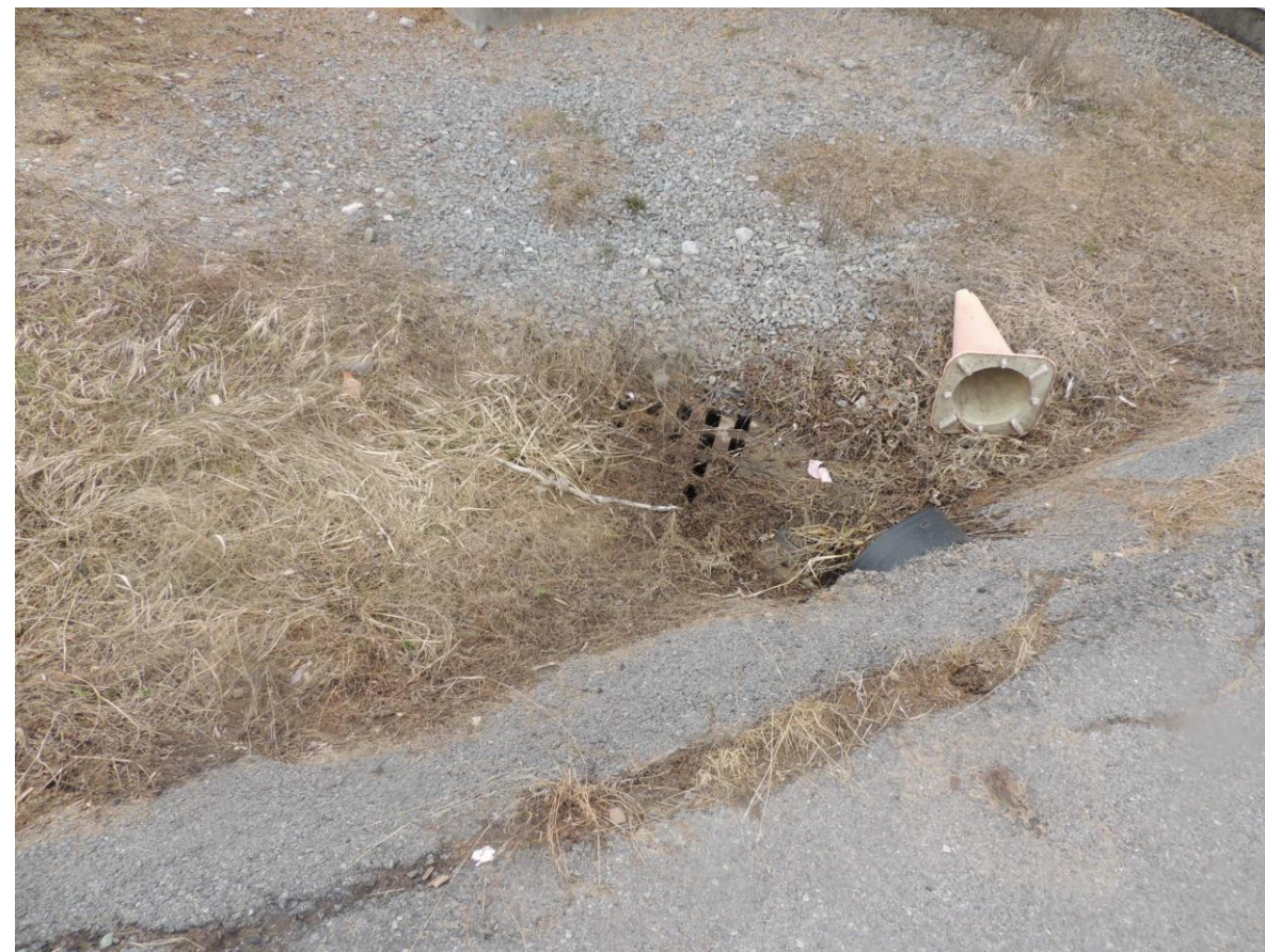
DSCN3987 – Storm inlet near southeast corner of packaging warehouse, that flows via pipe to the western edge of the Site
