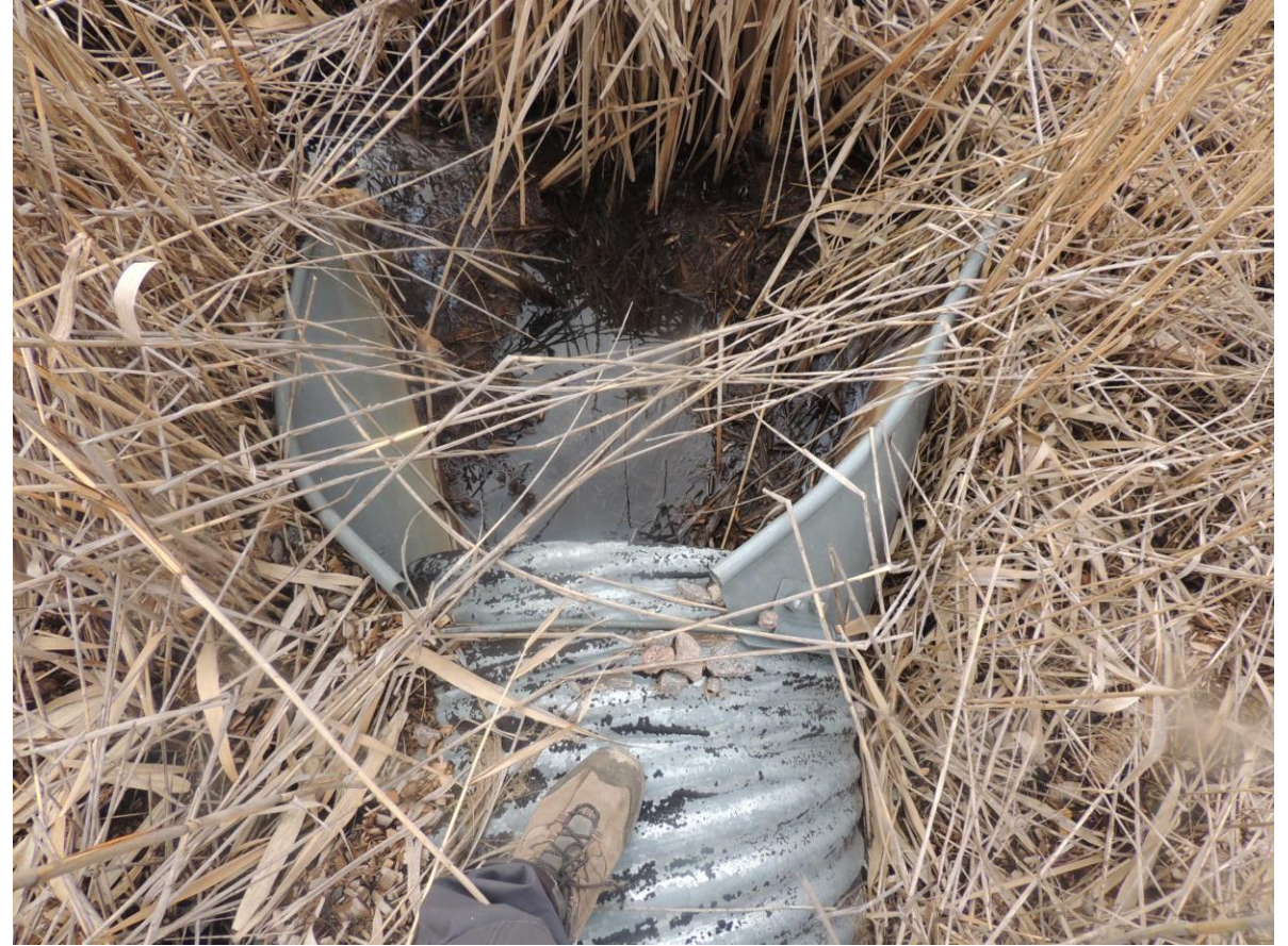
DSCN4015 – Stormwater culvert/channel western portion of Site at or around CSX rail line
