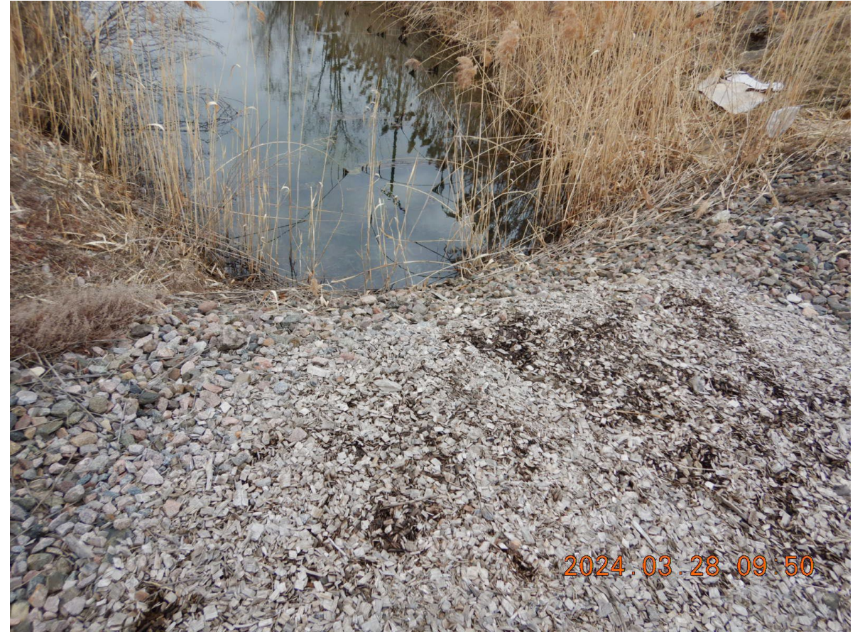
DSCN2676 - Gravel drive over stormwater runoff area connecting railroad area to loading parking lot on W side of Site
