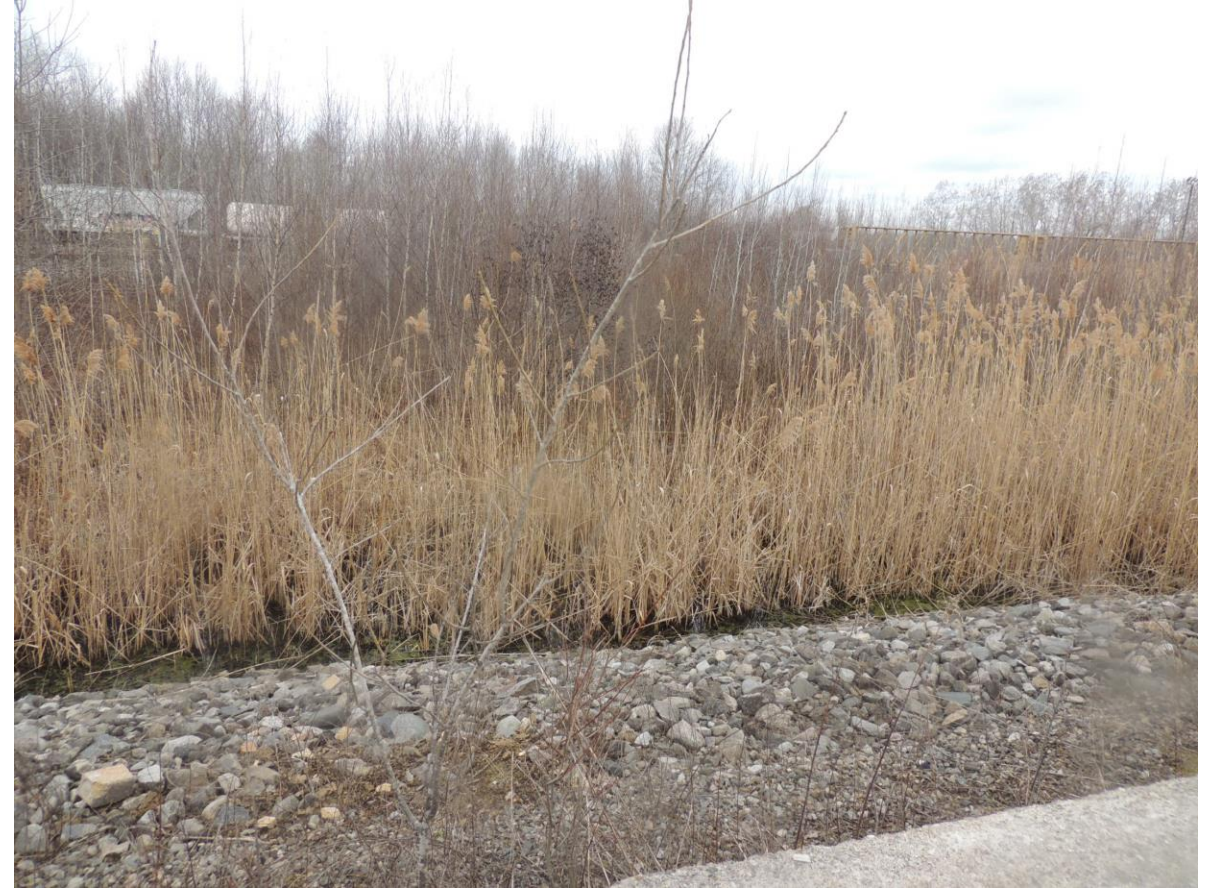
DSCN4031 - Block walls southwest portion of the Site – wet area with phragmites downgradient from the wall
