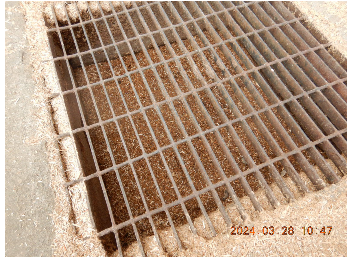
DSCN2754 - Catch basin #3 on S corner pellet manufacturing building – material seen in the catch basin
