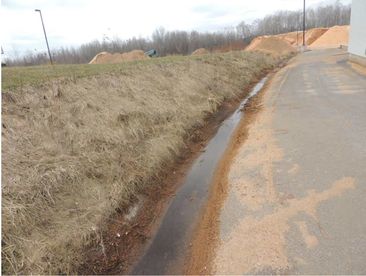
DSCN4063 - Swale with flow south of main building
