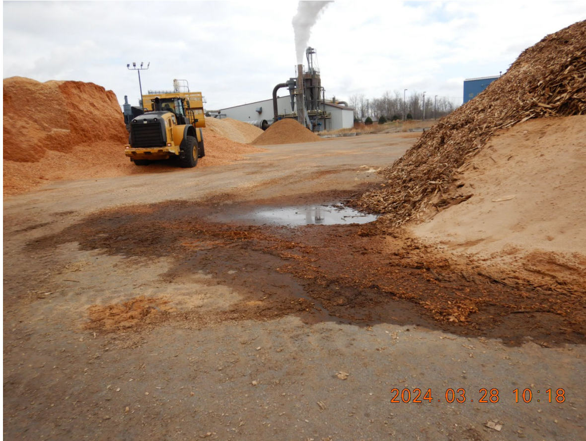
DSCN2710 - Stormwater runoff on S lot of Site
