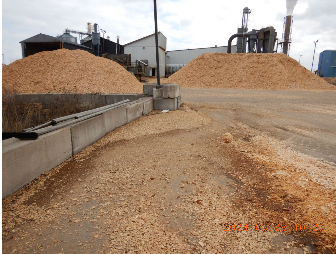
DSCN2717 - Stormwater runoff on S lot of Site
