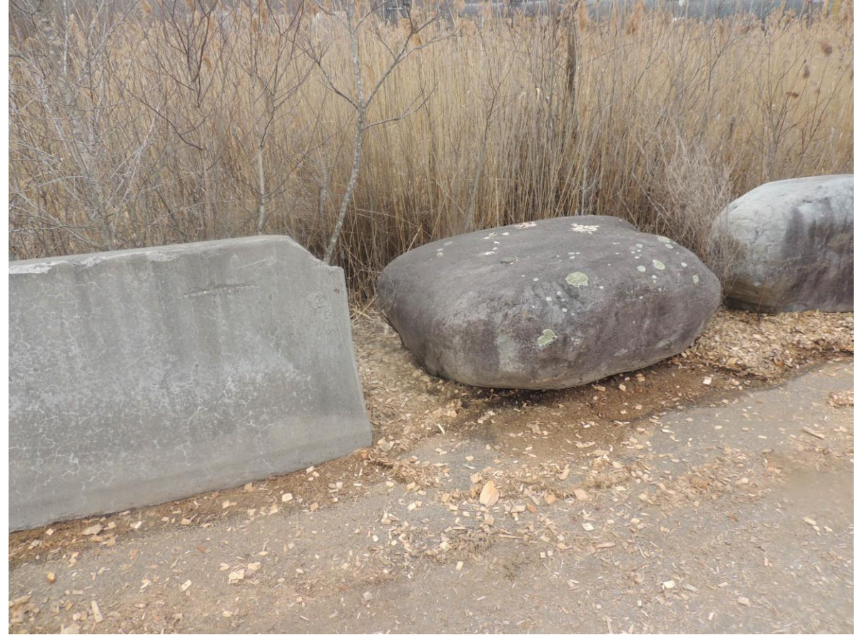
DSCN4035 – Gap in block wall. Southwest portion of the Site
