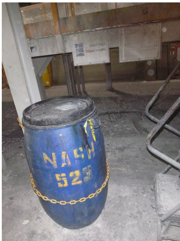
Photograph 23: Lump Breaker Deck Area.
