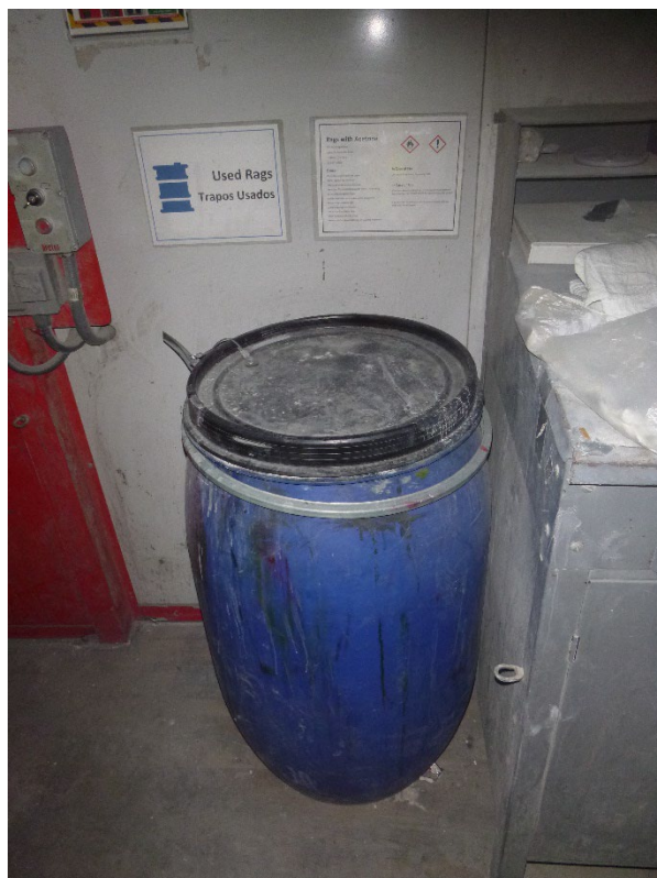
Photograph 20: Distributer Area ESCW container.
