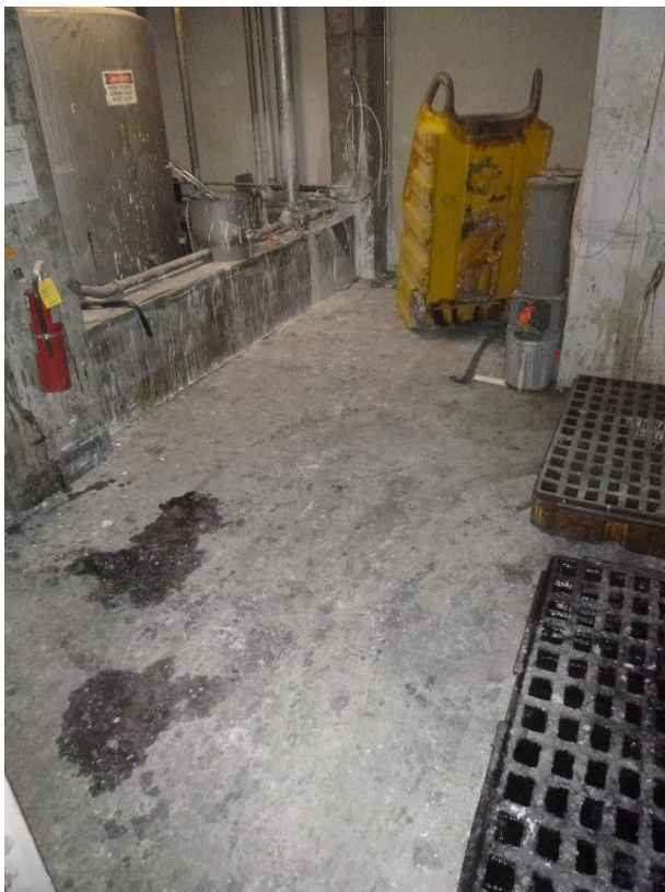
Photograph 11: Daily Tank Area.
