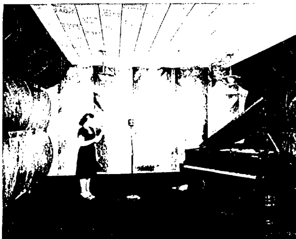
NOW The cylindrically constructed walls diffuse sound so loudness is evenly distributed. All studios with natural walls are the Paul A. Schmitt Music Co., Minneapolis.
