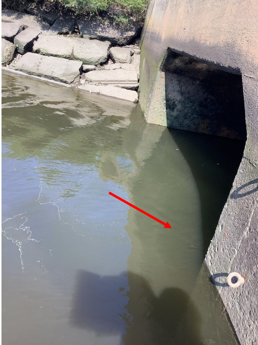
19. Strawb: Box culvert outfall for Strawberry Brook, located along Summer Street, flowing into the Saugus River. Sample point is indicated by a red arrow.
