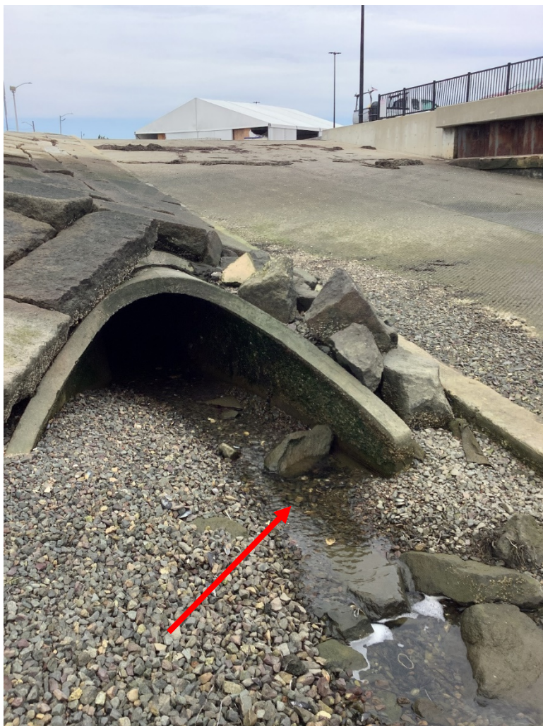
13. Blossom: Outfall located on the west side of the Blossom Street boat ramp. Sample point indicated by a red arrow.
