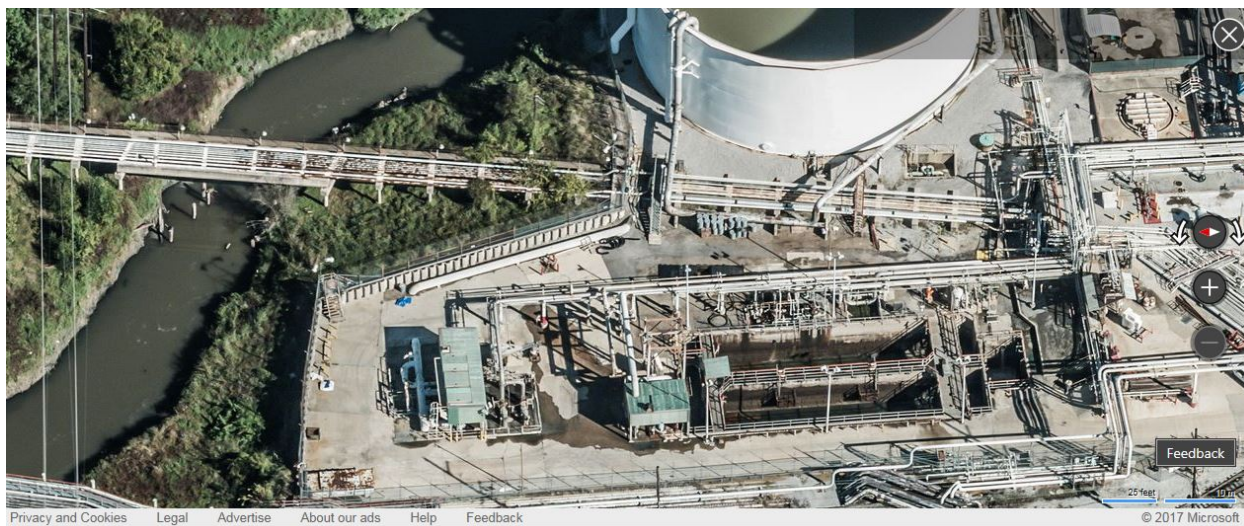
Aerial Photo 2 – View of separator unit, sump and gate valve for outfall 009 at end of unit, outfall 009 location, and partial view of one surge tank, using Bing Maps.
