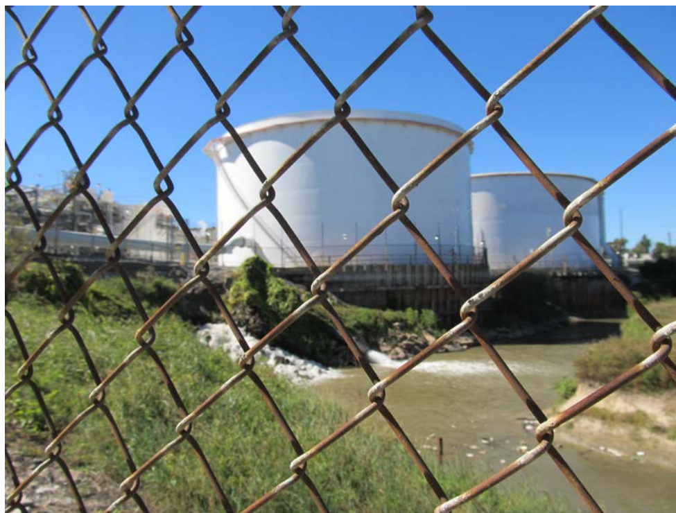
Photo 5 – Outfalls 001 and 004 discharge between the 2 surge tank areas, with view of the 2 western most tanks.
