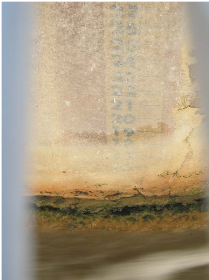
Photo 7 – Flow gauge at Parshall Flume
