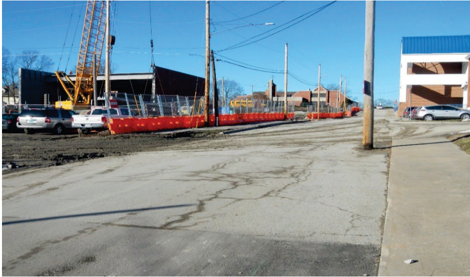
Photo 3, Sediment trackout onto 61 st Street from the construction site
