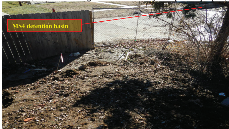
Photo 24, Sediment leaving the site into the adjacent private property.
