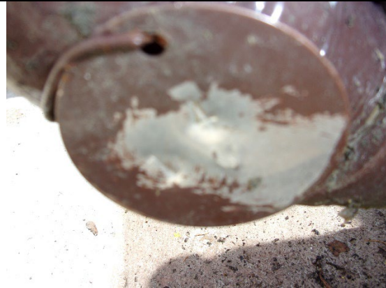
Figure 13: 10:04 AM Tank Farm Tag #4 partially illegible.
