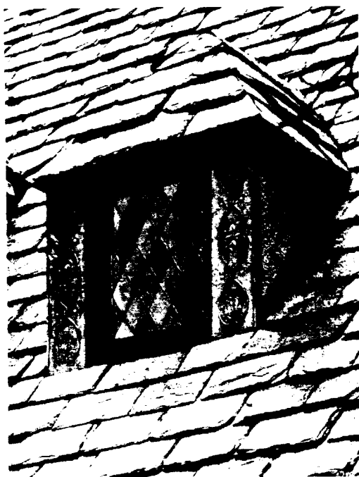
Detail of the dormer window showing the lead-covered face, cheeks, and lead comes in window
