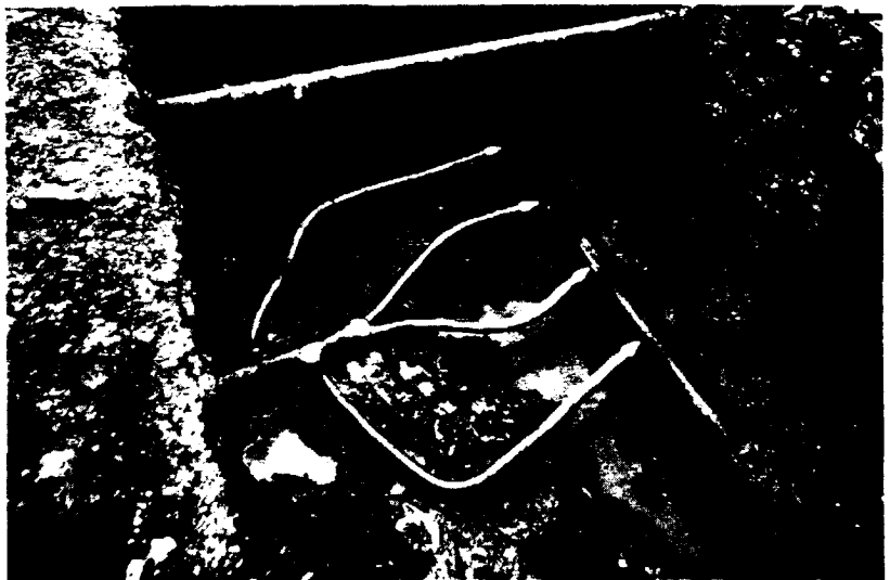
View showing four 1 in. taps serving a 2 in. water service from a 6 in. main in New Orleans
