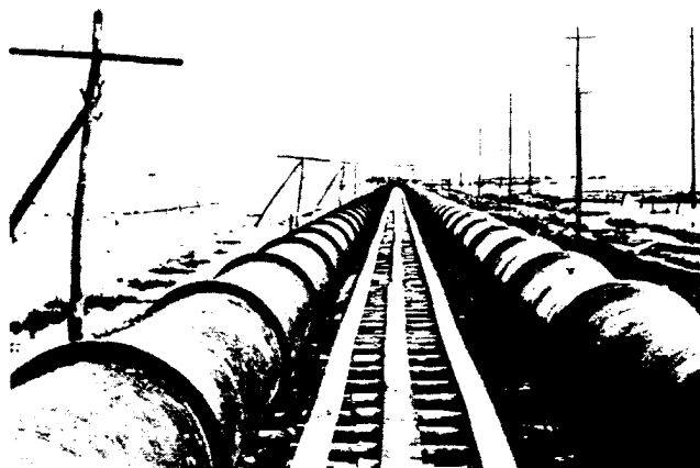
Old and new Atlantic City pipe lines. That on the left was laid in 1914, that on the right in 1937
