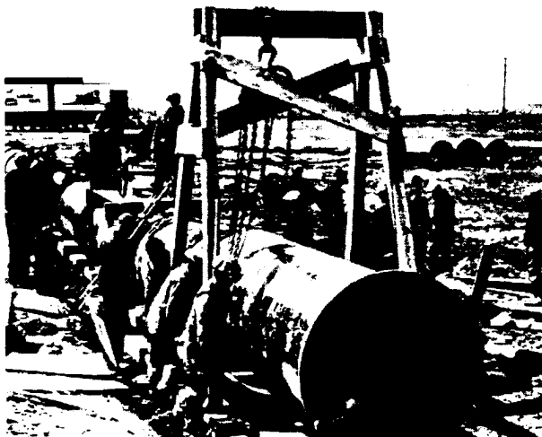
Setting the pipe on the cradles, using the portable derrick
