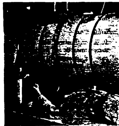
Use of dropcloth to contain wastes and facilitate clean-up.
