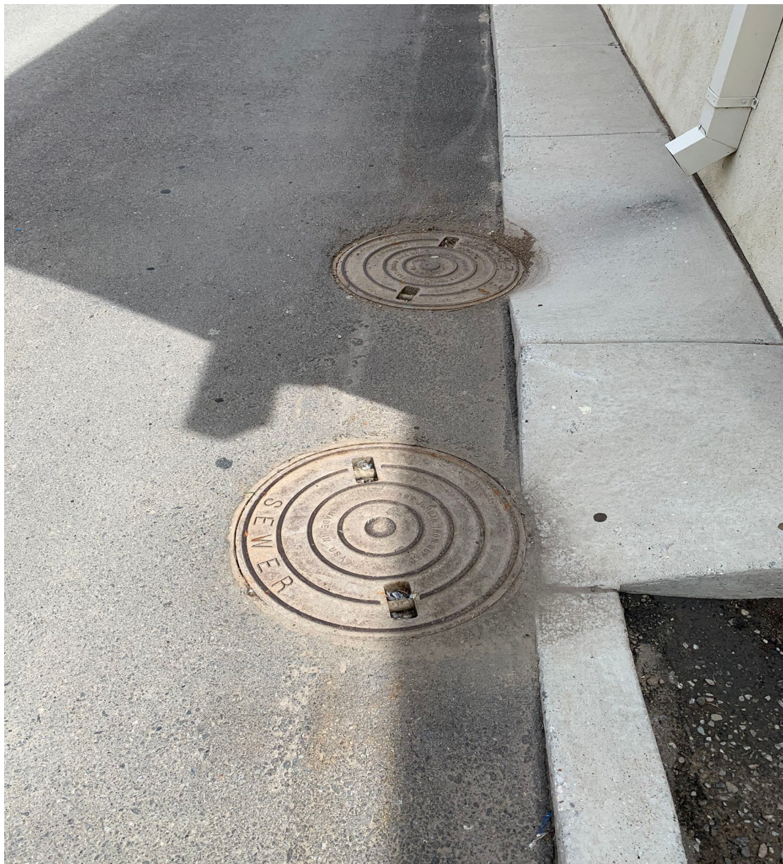
View of the Burger King Lift station vaults located within the drive-thru next to the building. (IMG0142). September 13, 2022. Photographed by D. Esparza West side of drive-thru next to building
