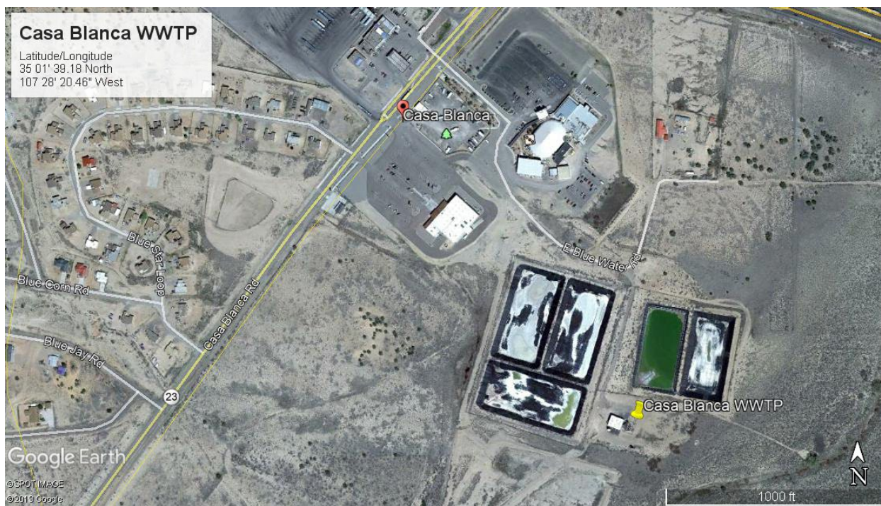
Aerial Image #1: Overall view of the Laguna Development Corporation- Casa Blanca Wastewater Treatment Plant location. Note: the evaporative lagoon cells. Aerial from Google Earth Maps.
