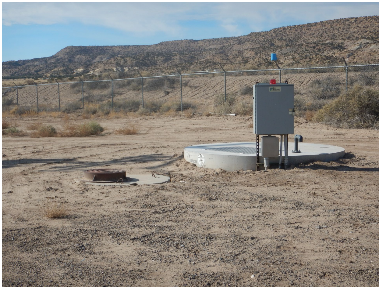
View of Lift Station (LS) WWTP#1 located at the approximate Northwest corner inside WWTP fenced perimeter. (DSCN1653). September 13, 2022. Photographed by D. Esparza
