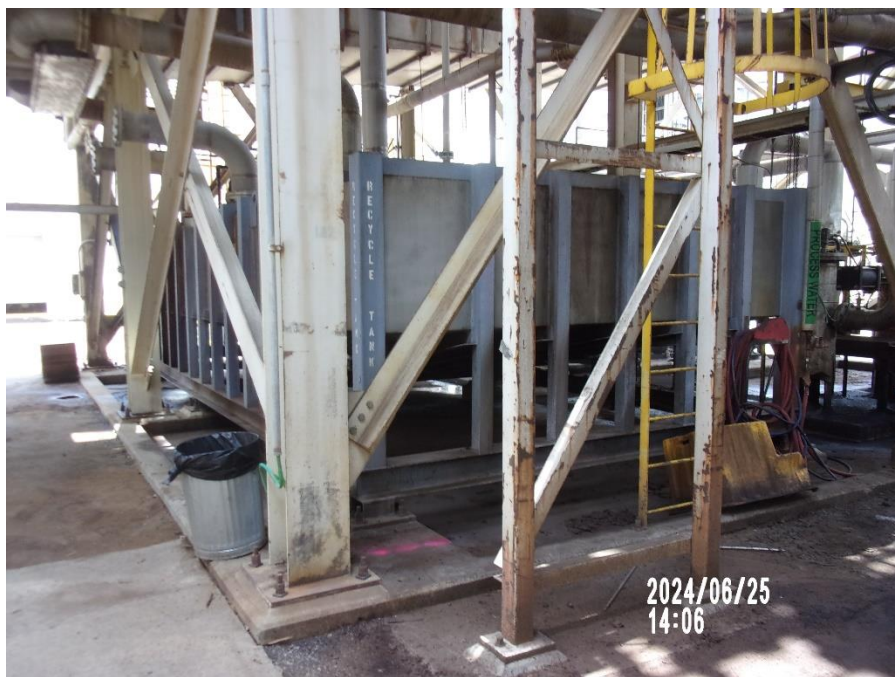
Photograph 7: Second view of tank where recycled RTO water is inputted into the Air Pollution Control System.
