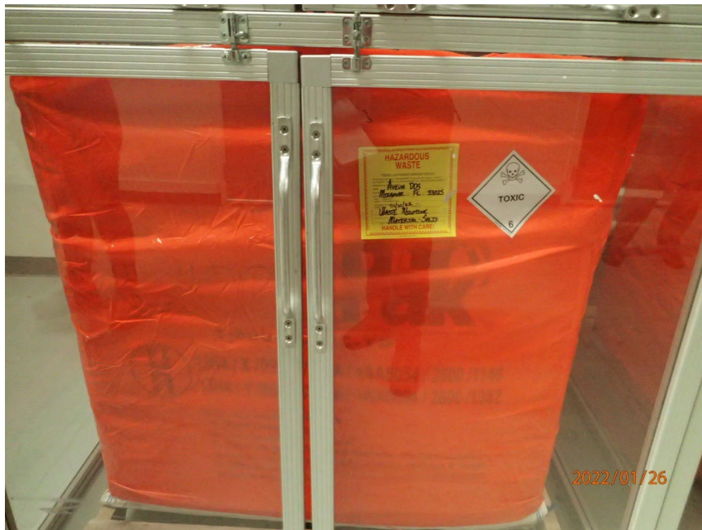
Photo 7: One (1) cubic yard box (CYB) with a liner, enclosed in a glass case with a latch that contained closed bags of waste nicotine material from the process packaging lines. The CYB was labeled "Hazardous Waste—Waste Nicotine Material Solid" and dated 1/21/2022. The CYB also had a DOT Toxic placard displayed as an indication of hazard.
