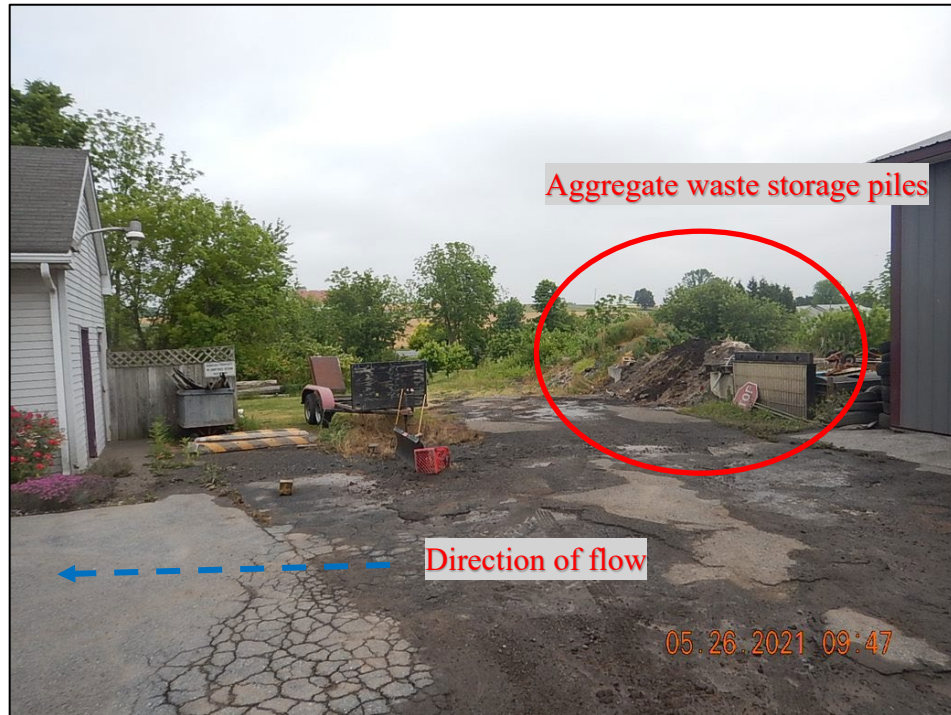
Photograph 5. Municipal Garage: (DSCN5091) View, facing north, of more storage buildings and aggregate waste storage in the northern portion of the property.
