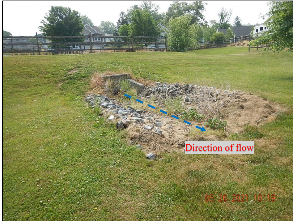
Photograph 17. Randall Drive Detention Basin: (DSCN5110) View, facing east, of the outlet structure for the detention basin.
