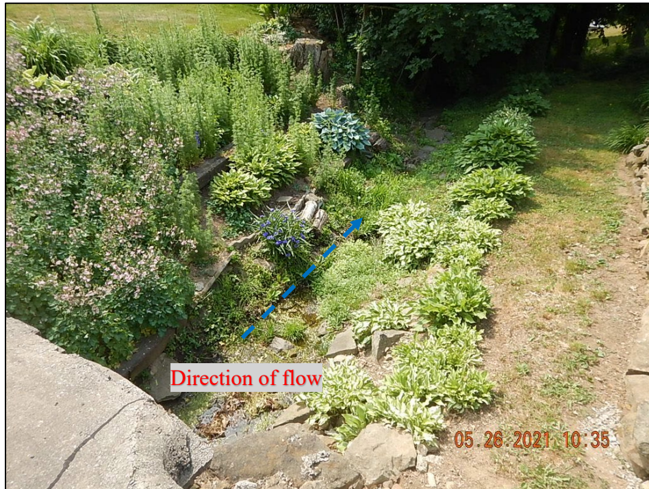
Photograph 23. Outfall #4: (DSCN5122) View, facing south, of the top of the headwall for Outfall #4 along Fairview Street.
