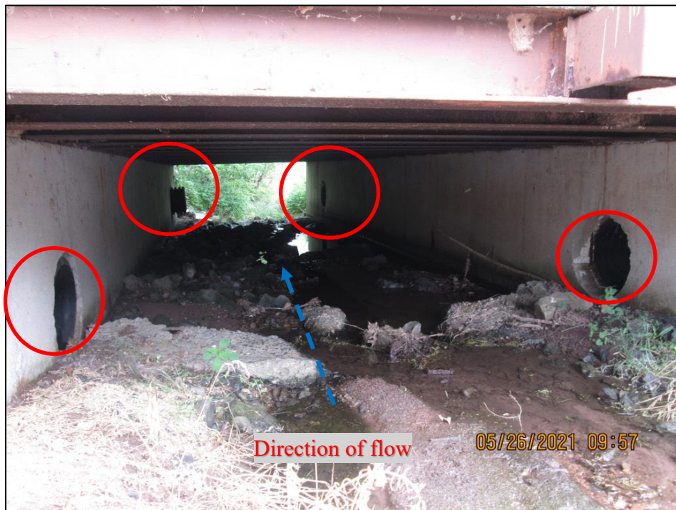
Photograph 14. Outfall #12: (IMG_1795) View inside outlet structure for Outfall #12. Note the four separate pipes leading into the structure that convey stormwater from both directions of Willow Street.
