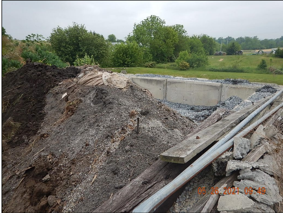
Photograph 7. Municipal Garage: (DSCN5093) Closer view of Photograph 6, facing east, of the wasted aggregates (primarily comprising dirt and crushed stone).
