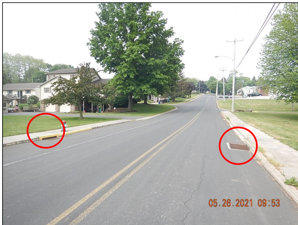
Photograph 10. Outfall #12: (DSCN5100) View, facing east along Willow Street, of the catch basins that collect roadway stormwater and convey it to Outfall #12.
