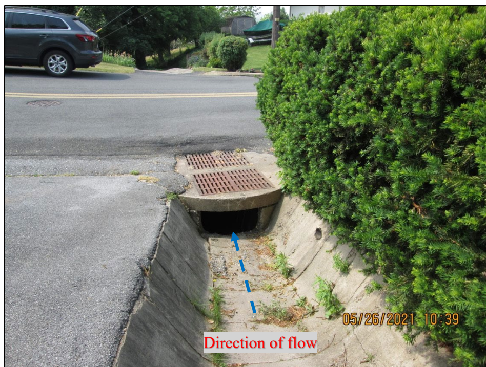
Photograph 26. Outfall #4: (IMG_1819) View, facing north, of culvert in Photograph 25 that flows to Outfall #4.
