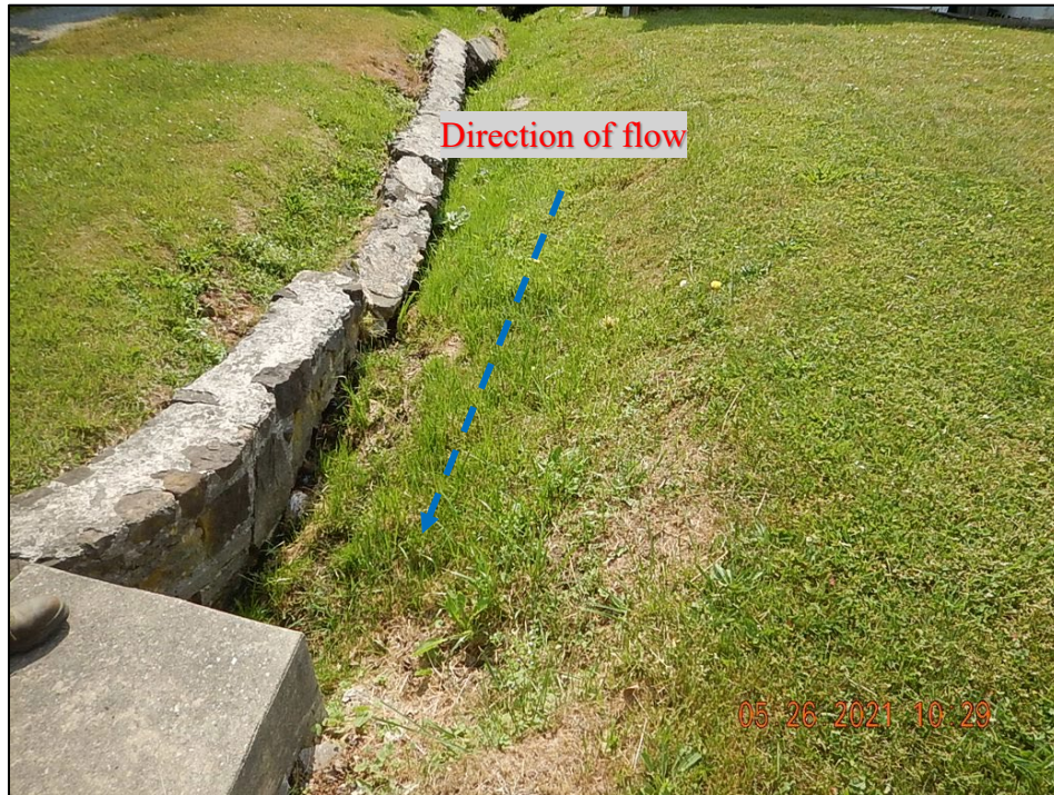
Photograph 21. Outfall #7: (DSCN5120) View of the channel from the private basin located on the southern side of Center Avenue that channels flow into Outfall #7.
