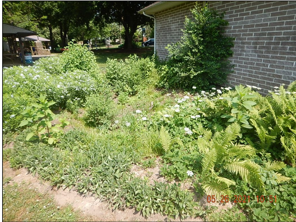
Photograph 31. Memorial Park Rain Garden #2: (DSCN5137) An additional view of Rain Garden #2. Note the excessive weeds and vegetation within the rain garden.
