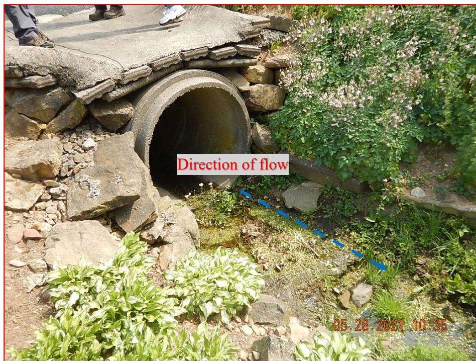
Photograph 24. Outfall #4: (DSCN5123) View, facing north, of the outlet pipe for Outfall #4. The structure appeared to be a 36-inch concrete pipe.
