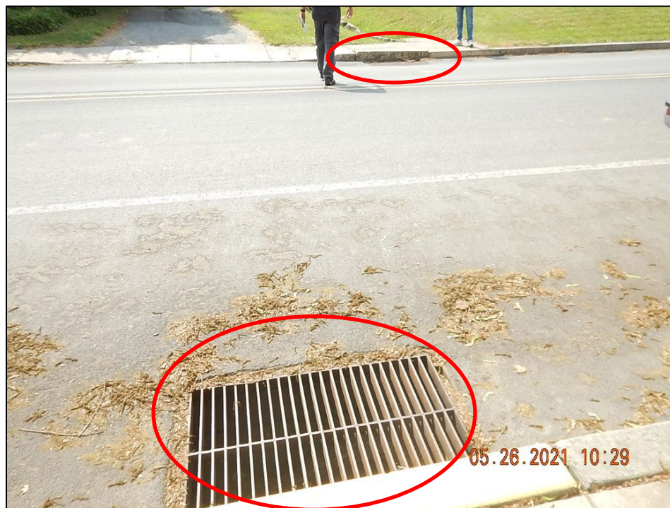
Photograph 20. Outfall #7: (DSCN5118) View, facing southeast, of the two catch basins on Center Avenue that drain into Outfall #7.
