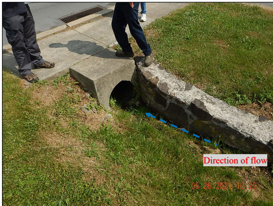
Photograph 22. Outfall #7: (DSCN5121) View, facing north, of the headwall at the end of the private basin channel that flows into Outfall #7.
