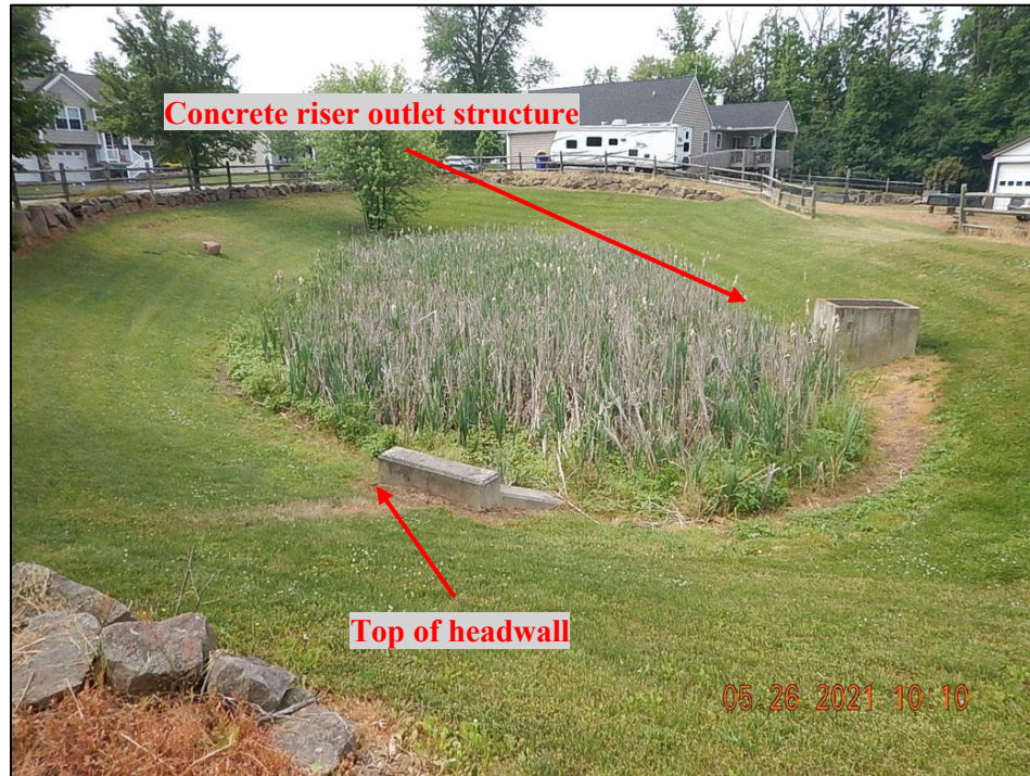
Photograph 15. Randall Drive Detention Basin: (DSCN5108) View, facing west, of the privately-owned and operated detention basin. This basin collects stormwater from the adjacent Randall Drive.
