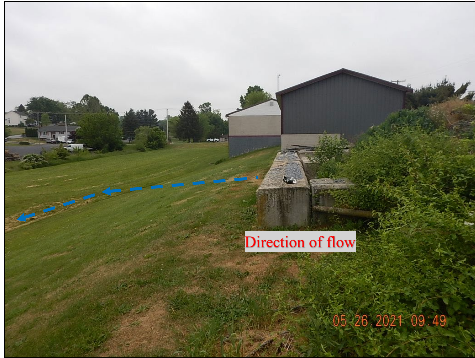
Photograph 9. Municipal Garage: (DSCN5095) View, facing south, of an infiltration swale located on private land to the east of the entire property. This swale collects stormwater from the eastern portion of the property.
