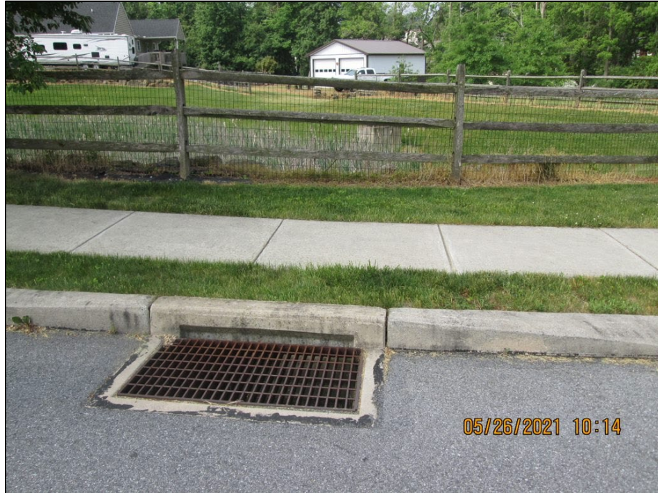
Photograph 16. Randall Drive Detention Basin: (IMG_1801) View of the primary catch basin along Randall Drive that conveys stormwater to the detention basin. Note the basin visible in the background.
