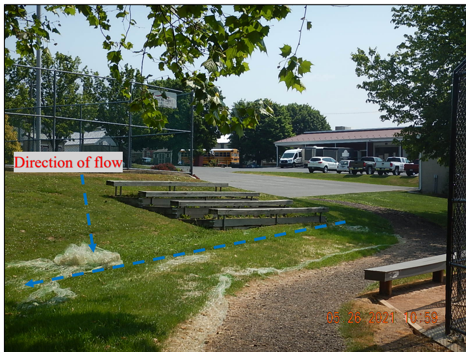
Photograph 34. Memorial Park Rain Garden #3: (DSCN5143) View, facing northeast, of the parking lot and tennis court that runoff and drain into the rain garden.
