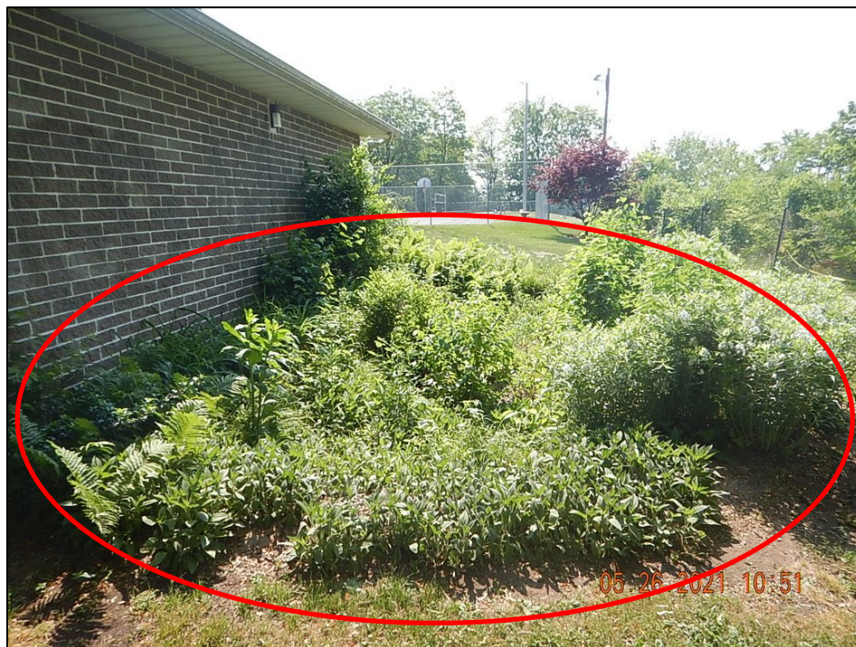
Photograph 30. Memorial Park Rain Garden #2: (DSCN5135) View of Rain Garden #2 at the Terre Hill Community Memorial Park which collects stormwater from the nearby grassy areas and adjacent building. Note the excessive weeds and vegetation within the rain garden.
