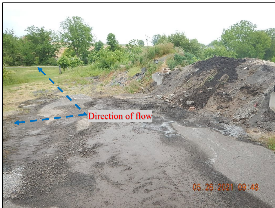
Photograph 6. Municipal Garage: (DSCN5092) Closer view of Photograph 5, facing north, of aggregate waste storage piles in the northern portion of the property. Note the migration of materials from the containment area. Stormwater from this area flows north offsite to a grass field.
