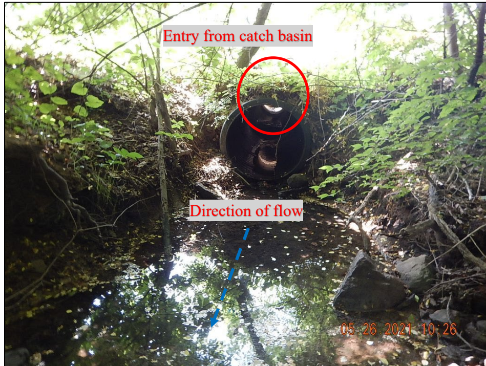
Photograph 19. Outfall #7: (DSCN5115) View, facing southeast, of the culvert under Center Avenue where Outfall #7 is located. Dry weather flow was visible at the time of the inspection. Borough representatives stated that the location is part of a spring-fed stream and flow is normal.
