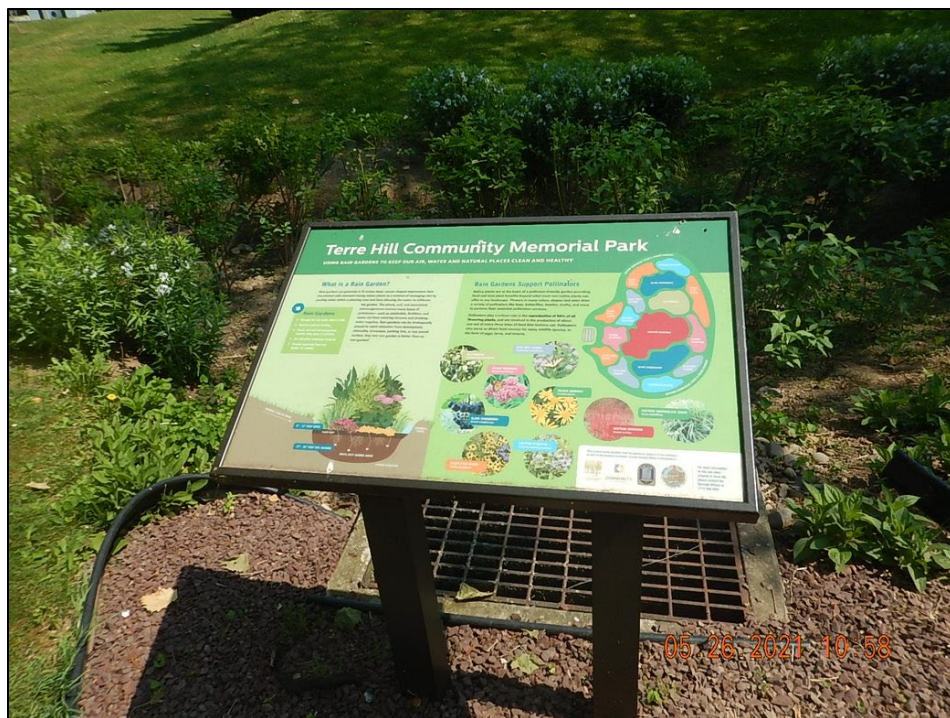
Photograph 32. Memorial Park Rain Garden #3: (DSCN5140) View, facing north, of Rain Garden #3 and attached inlet at the Terre Hill Community Memorial Park. This rain garden collects stormwater from an adjacent parking lot and tennis court.
