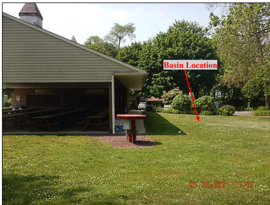
Photograph 36. Memorial Park Underground Storage Tank: (DSCN5145) View of Pavilion #1 at Terre Hill Community Memorial Park. Rainwater from the roof of the pavilion is stored in an underground 2,000-gallon storage tank. Some stormwater is also able to collect through the inlet drain to the tank.
