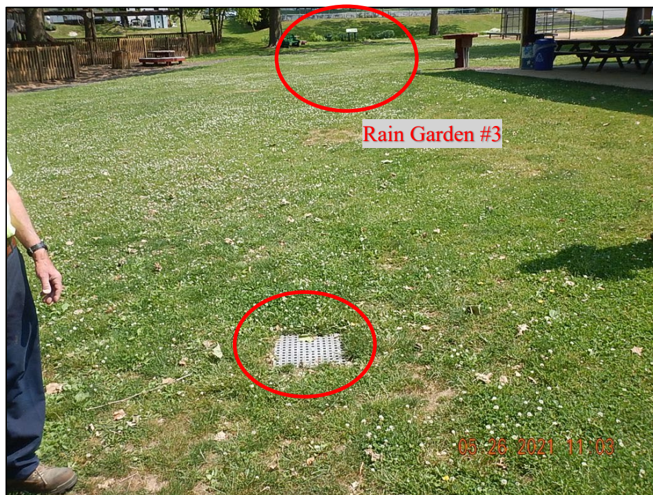
Photograph 37. Memorial Park Underground Storage Tank: (DSCN5147) View, facing north, of the drain into the underground storage tank that collects rainwater from park pavilion and surrounding area.
