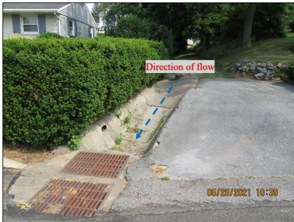
Photograph 25. Outfall #4: (IMG_1817) View, facing north, of culvert that flows into Outfall #4.
