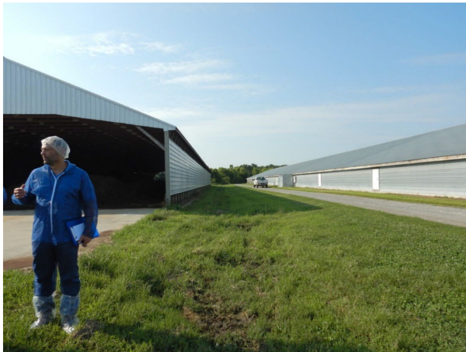
Photograph 14. Downgradient view of the stormwater drainage on the west side of the southern manure storage facility that conveys flows from the manure storage buildings to the stormwater basin.
