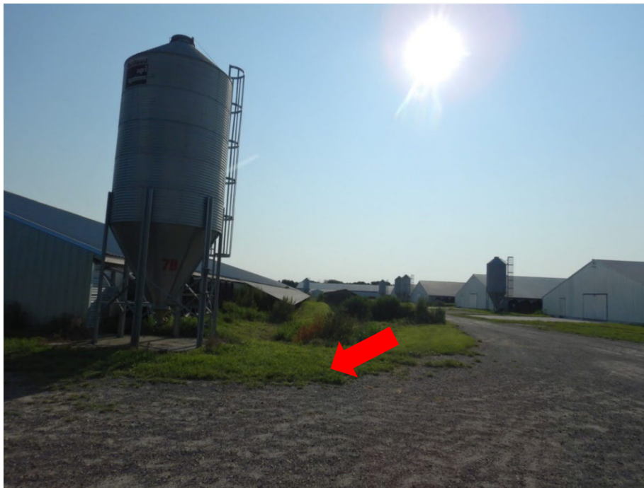
Photograph 8. View of the southern wall of Poultry House 7. A drainage and a culvert (red arrow) convey runoff from the roof and the areas surrounding the house to the western edge of the facility.
