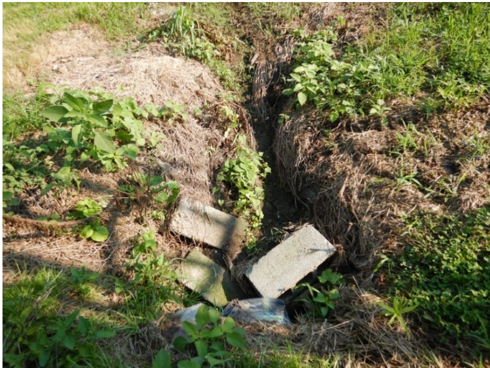
Photograph 24. Close up view of the culvert in the drainage between Poultry Houses 1 and 2.
