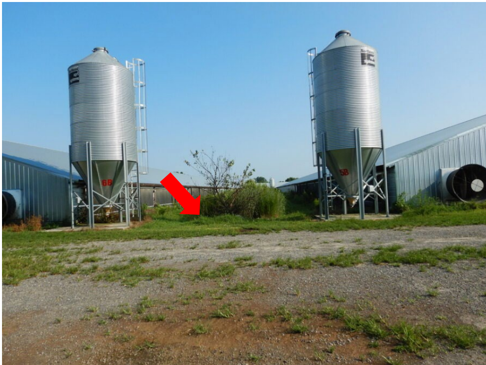
Photograph 28. View, looking north, of the area between Poultry Houses 5 and 6.
