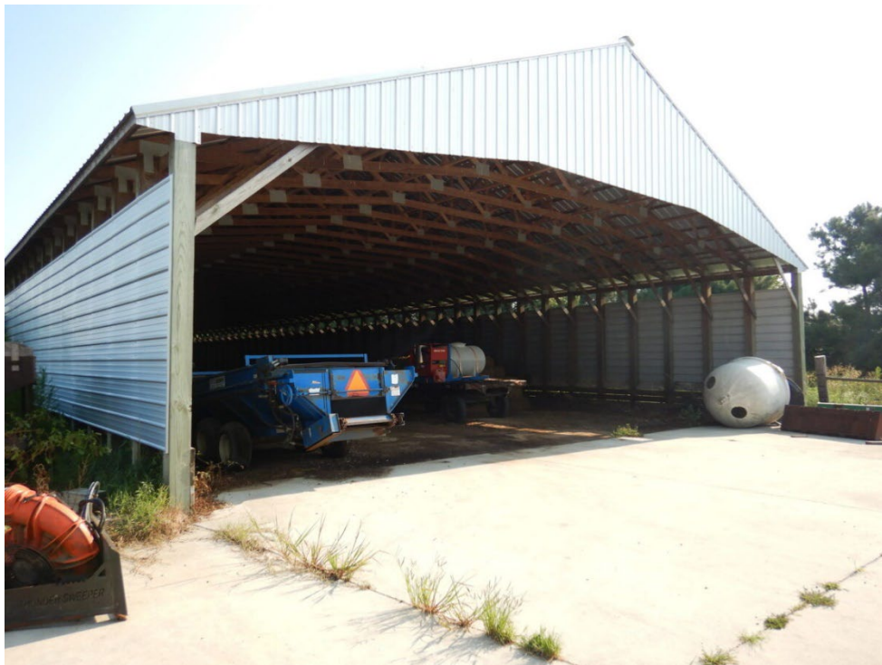
Photograph 12. View of the northern manure storage building and the concrete pad on the southern end of the building.
