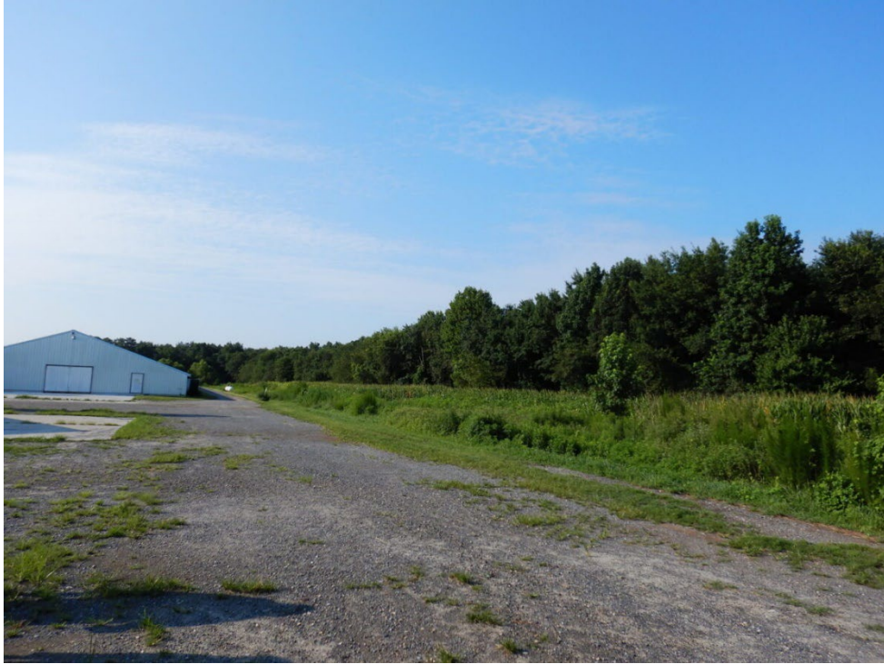
Photograph 5. View of the western edge of the facility, taken from the north.
