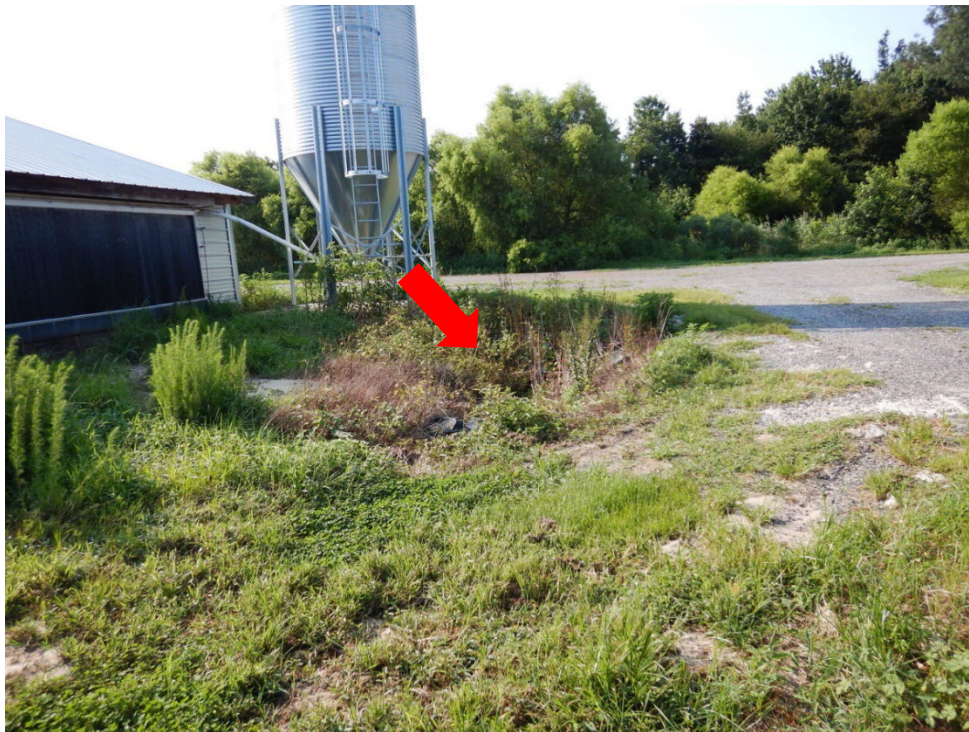
Photograph 30. View of the drainage culvert (indicated by the red arrow) between Poultry Houses 3 and 4. Stormwater runoff flows south through the culvert to the stormwater basin.
