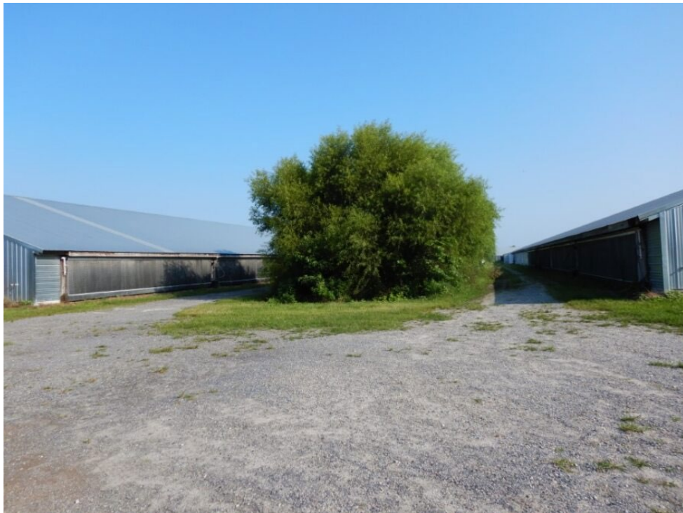
Photograph 26. View of the area between Houses 3 and 4 from the south.
