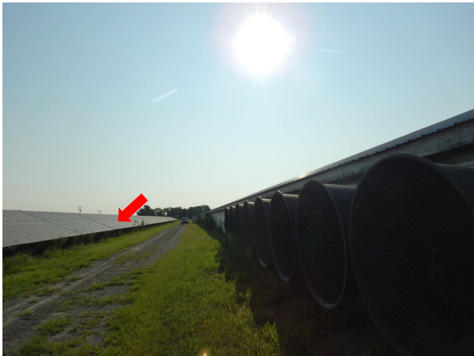
Photograph 4. View of the northern wall of the Poultry House 8 from the west. The solar panels (red arrow) run along the northern edge of the facility and have a drainage ditch underneath them.
