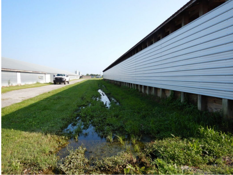
Photograph 15. Upgradient view of the stormwater drainage located west of the southern manure storage facility that conveys flows from the manure storage facilities to the stormwater basin.
