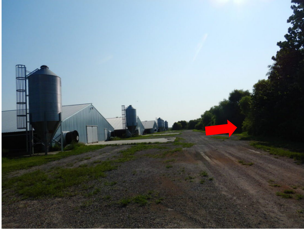
Photograph 29. View, looking east, of the area south of Poultry Houses 1 through 6. The red arrow shows the location of the stormwater basin on the south side of the facility.
