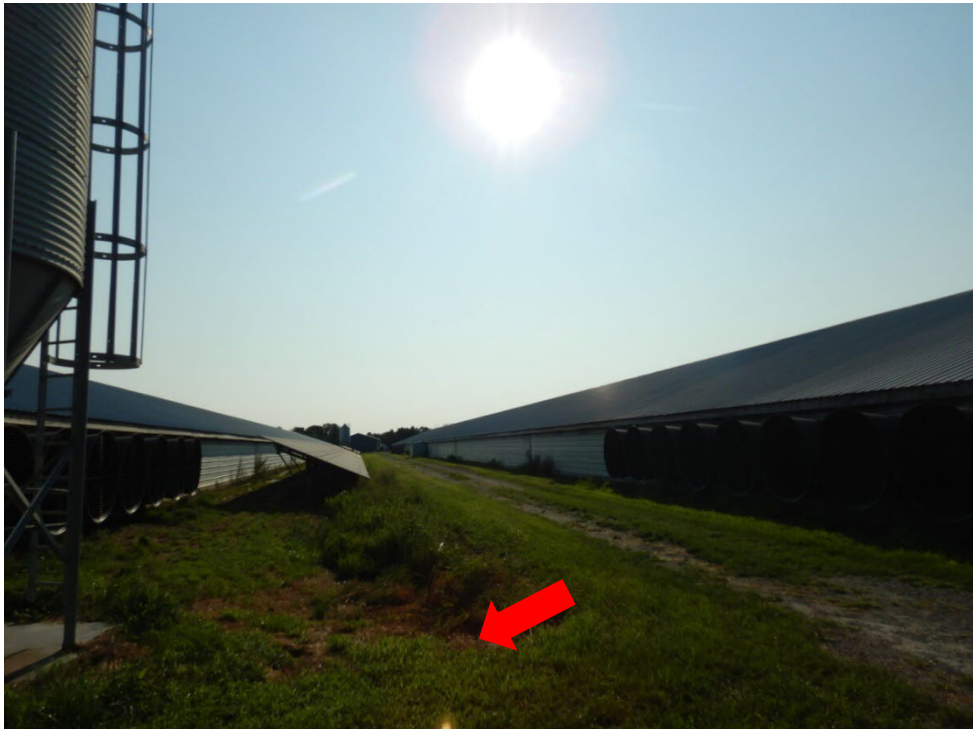
Photograph 6. View of the area between Poultry Houses 7 and 8. A drainage and a culvert (red arrow) convey runoff from the roof and the areas surrounding the houses to the western edge of the facility.
