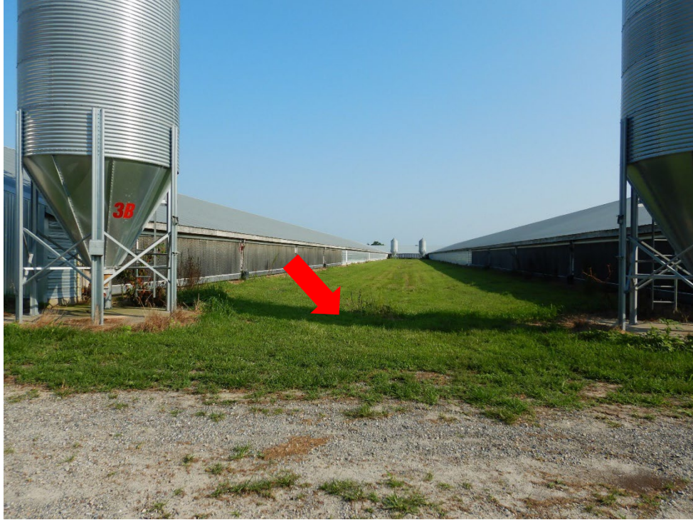
Photograph 25. View, looking north, of the area between Poultry Houses 3 and 4. Stormwater runoff flows south through the drainage to a culvert (red arrow) that conveys it to the stormwater basin.
