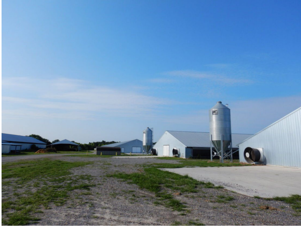
Photograph 1. Overview of the facility, view from the northeastern corner, near the facility entrance.
