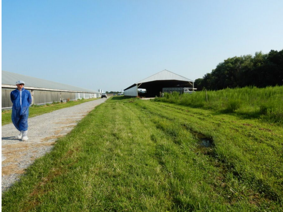
Photograph 17. Upgradient view of the stormwater drainage shown in Photographs 14-16. The southern manure storage facility is visible in the background. The stormwater drainage conveys flows from the manure storage facilities to the stormwater basin.
