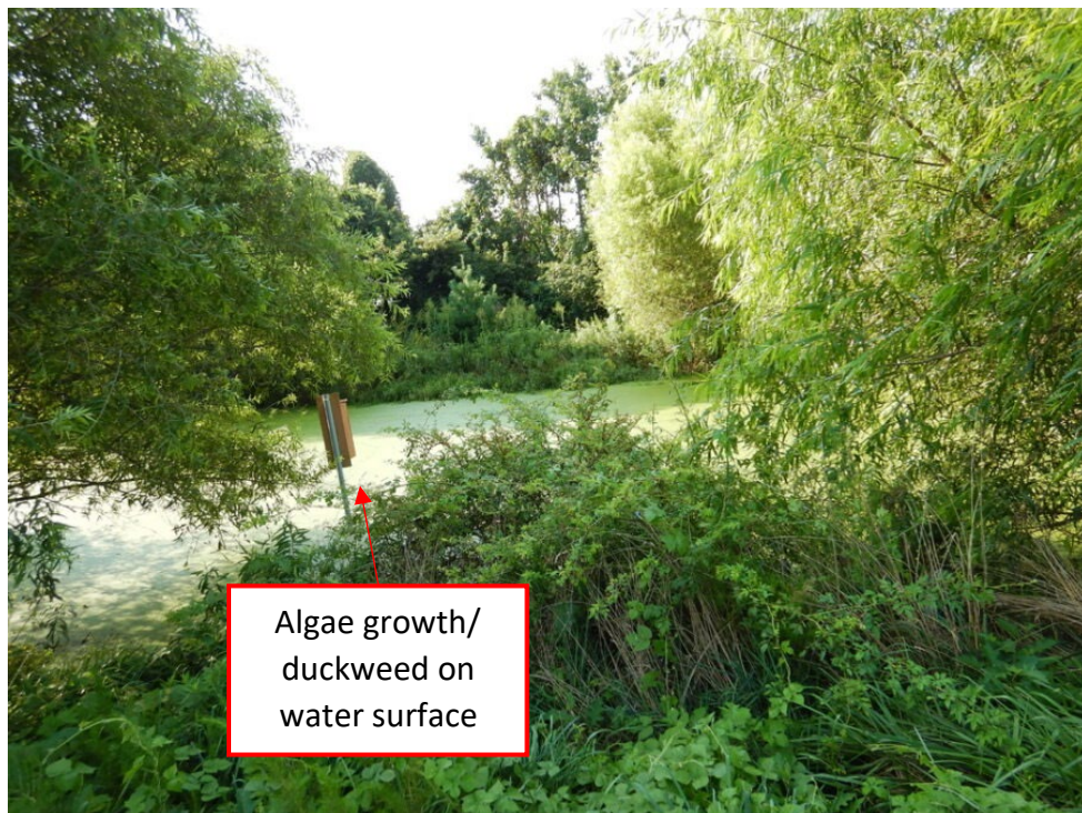
Photograph 22. Second view of the stormwater basin on the south side of the facility. The surface of the water is covered by a layer of algae and/or duckweed.
