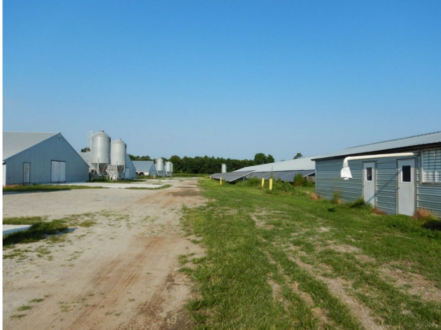
Photograph 9. View, looking west, of the area between the southern wall of Poultry House 7 and the northern walls of Poultry Houses 1-6.
