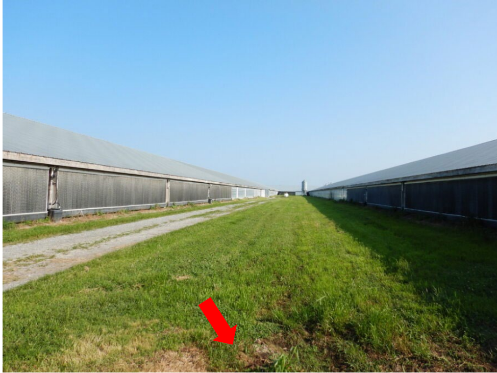
Photograph 23. View of the area between Poultry Houses 1 through 2 from the south. Stormwater runoff flows south through the drainage to a culvert (red arrow) that conveys it to the stormwater basin.
