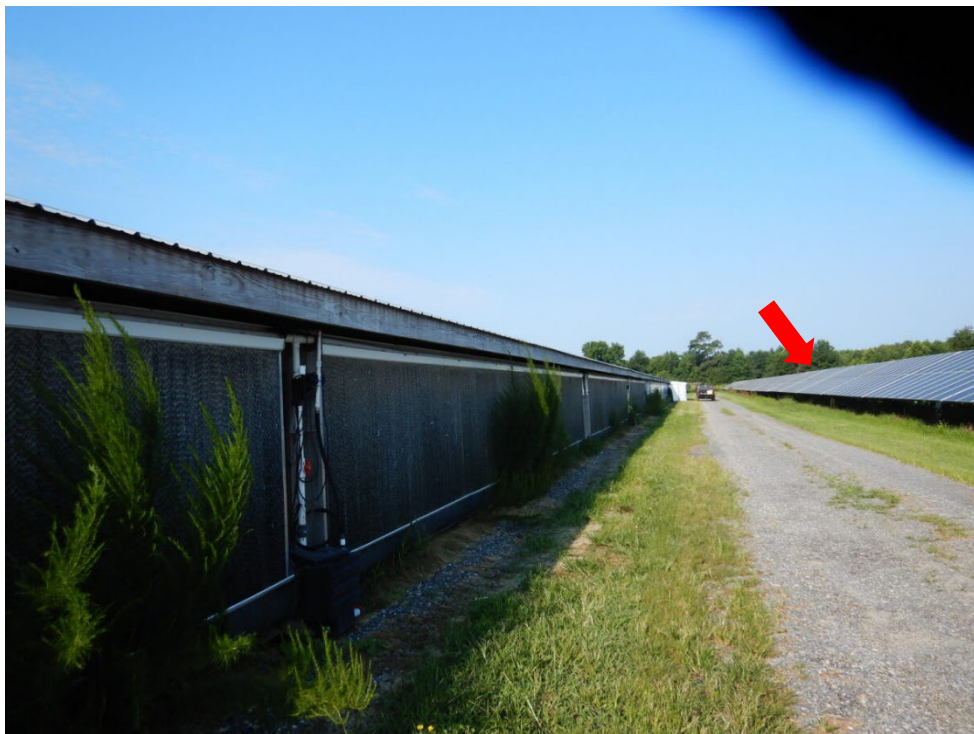
Photograph 2. View of the northern wall of Poultry House 8 from the east. The solar panels (red arrow) run along the northern edge of the facility and have a drainage ditch underneath them.
