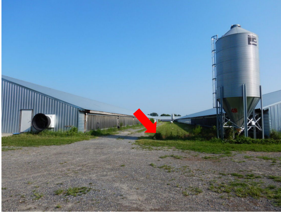
Photograph 27. View, looking north, of the area between Poultry Houses 4 and 5. Stormwater runoff flows south through the drainage to a culvert (red arrow) that conveys it to the stormwater basin.
