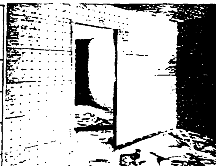
Ready for Plastering
