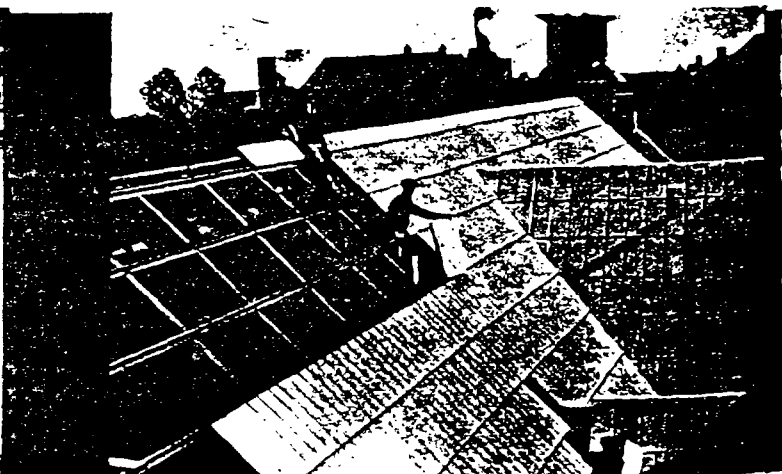
Pyrobar Roof Tile are adapted to construction involving steep slopes.
