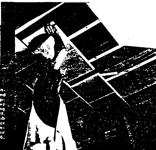
Cross scored tile applied without regard to joist spacing.
