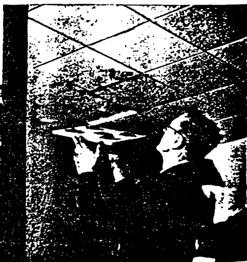
Weatherwood Tile applied with adhesives to flat surfaces.
