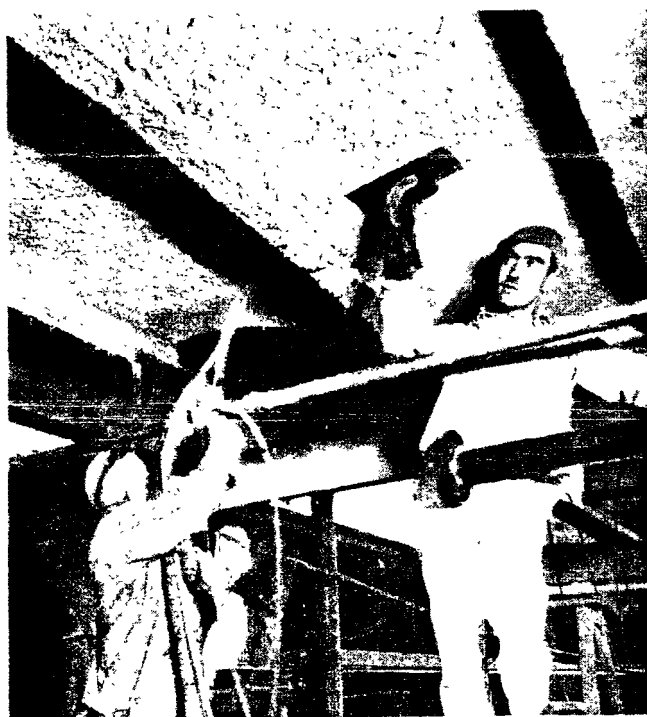
Spraying K & M Limpet as a deck insulation
