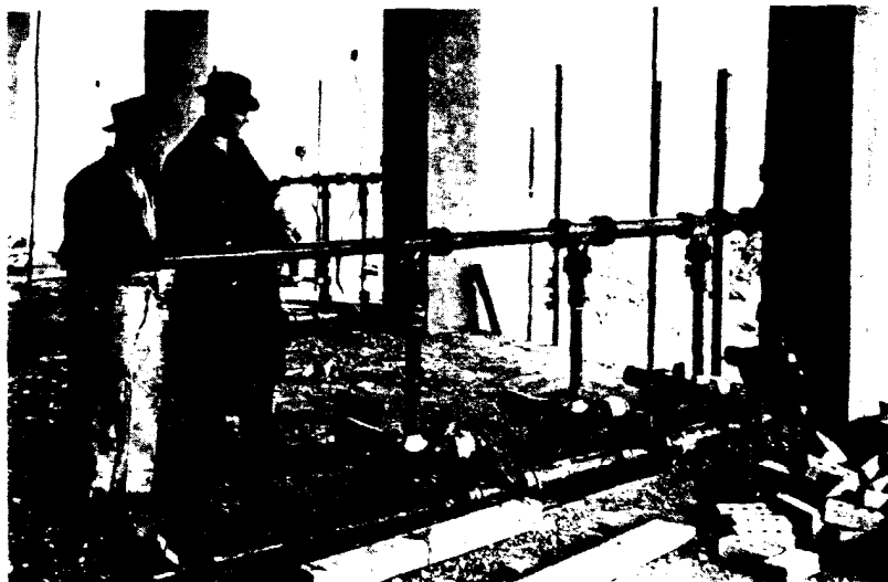
Roughing-in with cast iron and lead for the new Central Office Building of the Southwestern Bell Telephone Company, as required under Port Arthur's plumbing code. I. R. Timlin, St. Louis, Mo. and W. J. Knight & Co., of the same city, were architect and engineers respectively. The photograph shows William R. Tooley, City Plumbing Inspector, at right, and V. D. Houston, Local 617, journeyman plumber, at left. H. B. Paggi, Port Arthur, Texas, was the plumbing contractor
