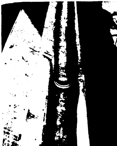
Left, loose-locked joint in lead-lined gutter. The lock is filled with non-hardening compound
