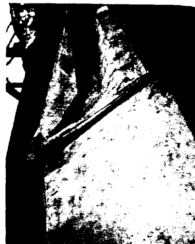
Left, side-wall and valley flashings for dormer window. flashings interwoven with the shingle courses
