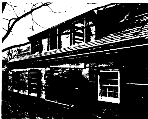
Left, lead side-wall flashings and window-sill flashings for the large dormer. The end-wall flashings between the dormer windows are not yet installed
