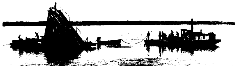
HERBERT R. FITCH An 1886 photograph showing the laying of the San Diego water main, made of cast iron with lead-calked joints
