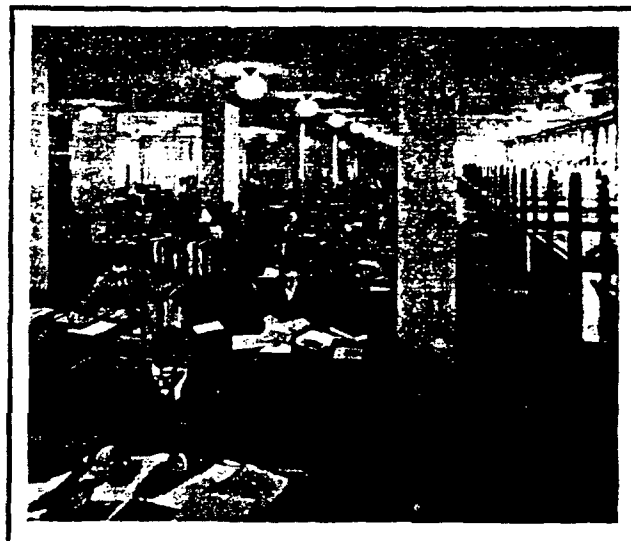
300 WEST ADAMS ST. BUILDING, CHICAGO J. J. JENSEN, ARCHITECT
