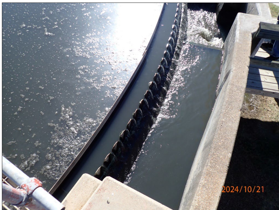
Photograph 17. Weir of the east primary clarifier. Note the air bubbles on the surface of the clarifier.
