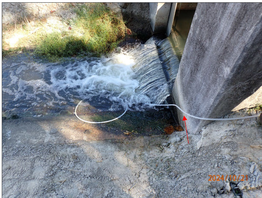
Photograph 37. Effluent weir and Outfall 001. Note the red arrow indicating the auto sampler intake tubing.
