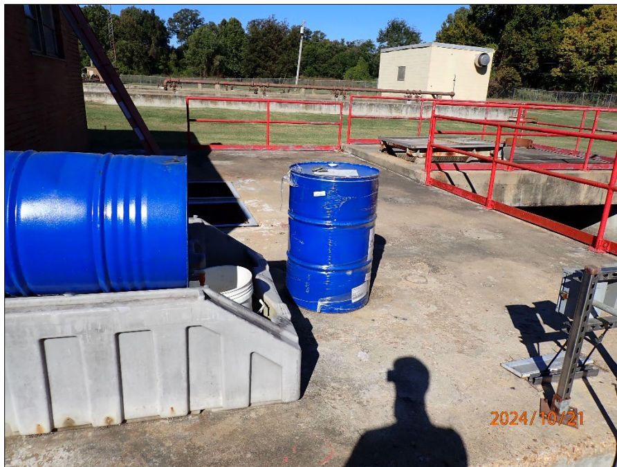
Photograph 4. 55-gallon drum of oil without secondary containment, located near the influent pump station and wet well.
