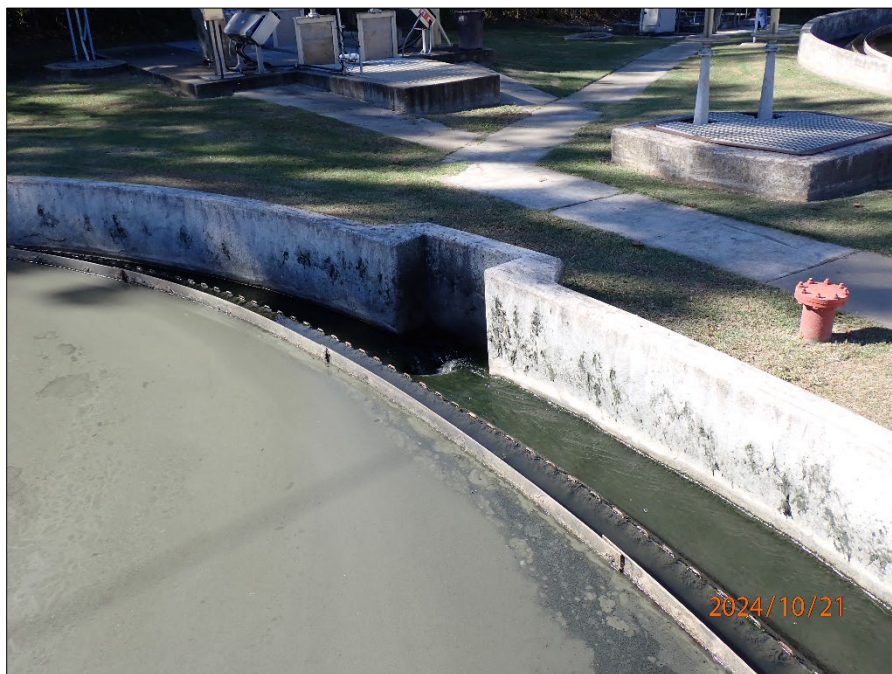
Photograph 26. East secondary clarifier weir.
