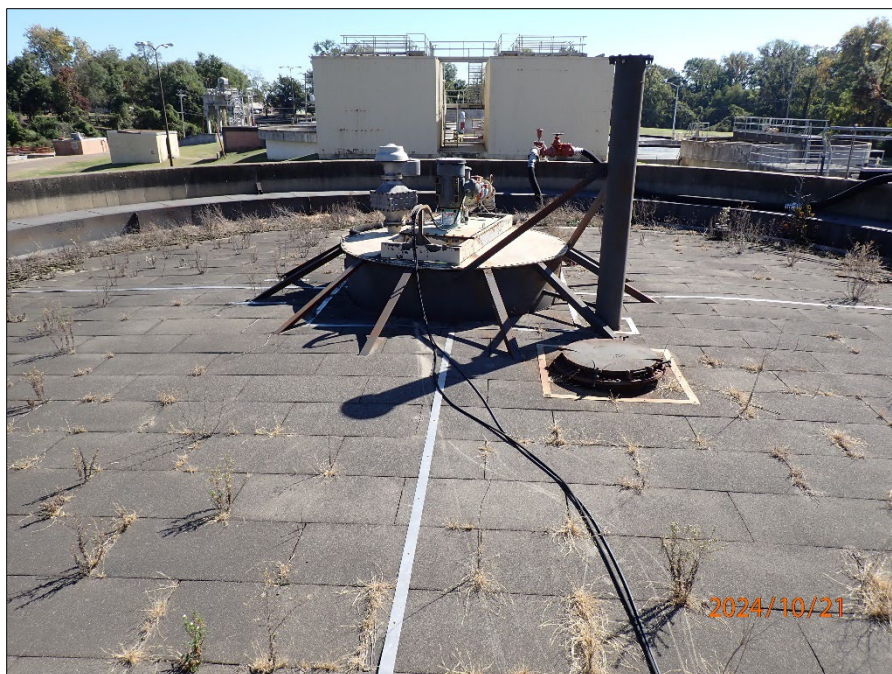
Photograph 45. Top of the north anaerobic digester.
