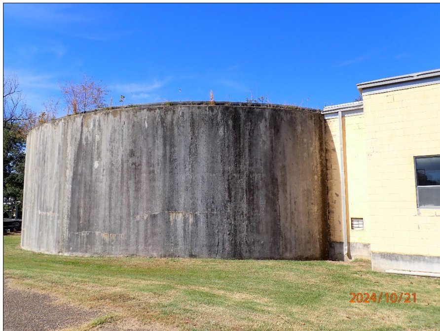
Photograph 44. South anaerobic digester. Note this digester was out of service at the time of the inspection due to sludge buildup and compaction within the digester.
