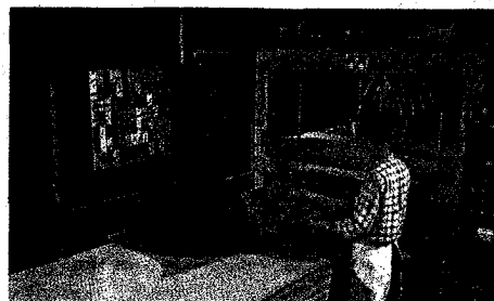
The Formica sheet is given a satin or "furniture" finish in Evendale, Ohio, plant.
