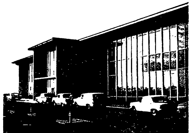
Modern Kellogg Division plant at Oxnard, California houses Division manufacturing, administrative and engineering functions.
