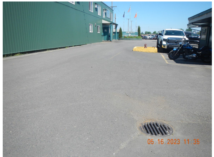
Photo #:12 (DSCN3267) Description: Facing north, photo of storm drain catch basin west of the metal/fabrication shop.
