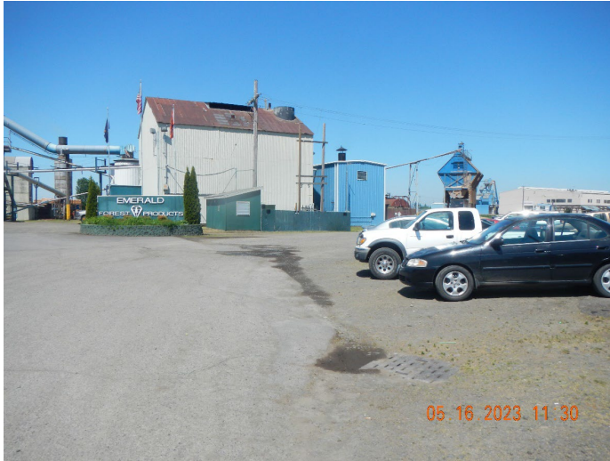
Photo #:09 (DSCN3264) Description: Facing west, photo of northern catch basin within Basin 5.
