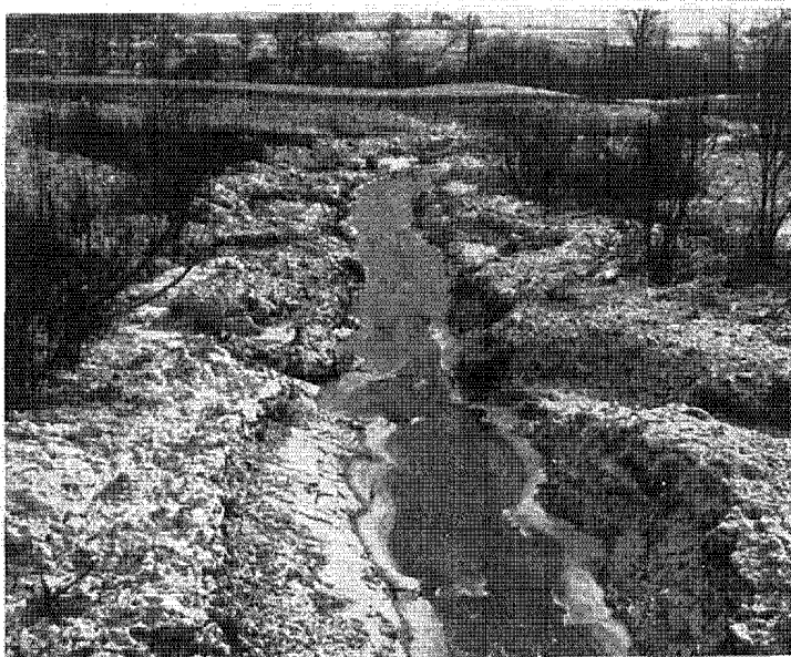
Before and after du Pont ditching dynamite had taken a hand at stream-correction work. The hatched line in the top picture shows the location of holes
