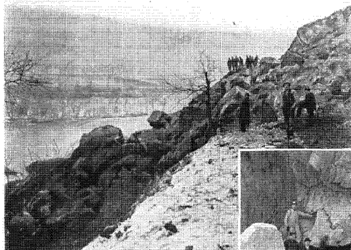
Above—After the shot. Right—Entrance to the coyote tunnel, from a picture taken during loading operations. Above, right—A long-distance view of the same spot. The projecting cliff you see here had to be brought down—and it was
