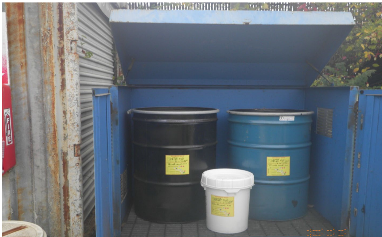
7. Hazardous Waste Accumulation Area – WMATA Bladensburg – 10/25/22
