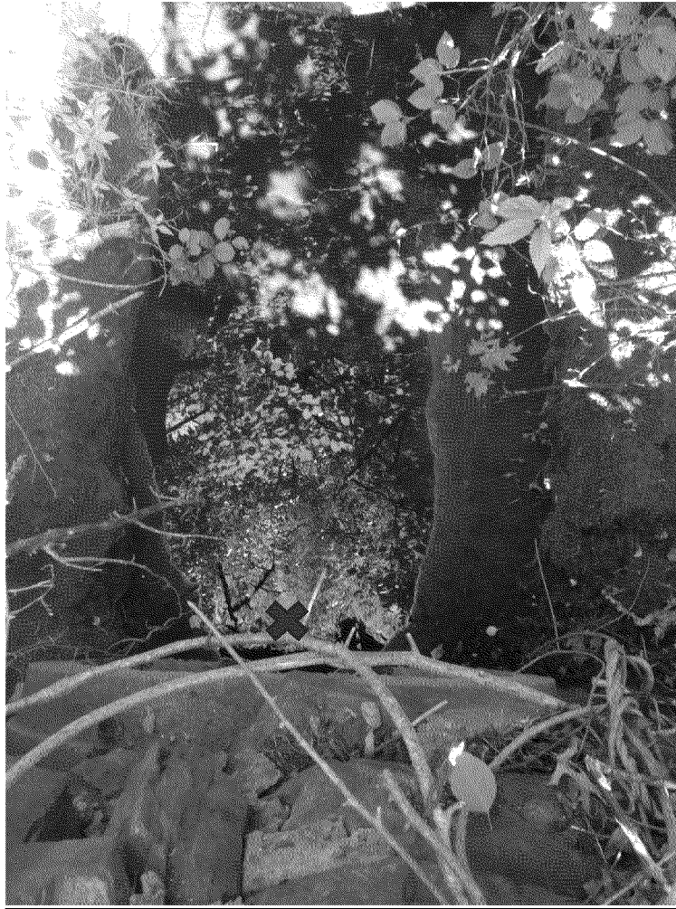
Photo 3: D2328 (photo taken 07/02/2024 at approx. 10:00) Outfall located near 650 Amherst St, discharging into the Pennichuck Pond. Sample points are indicated by a red X.
