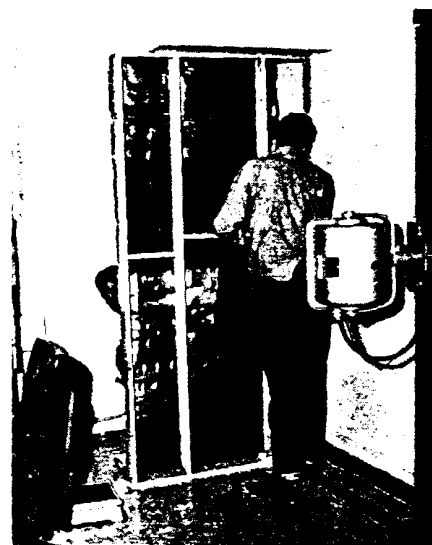
In the office where the X-ray screen was erected (left) the beams were directed towards a doorway. The lead was fastened only at the edges (right) to prevent any penetration which could result in leaks.
