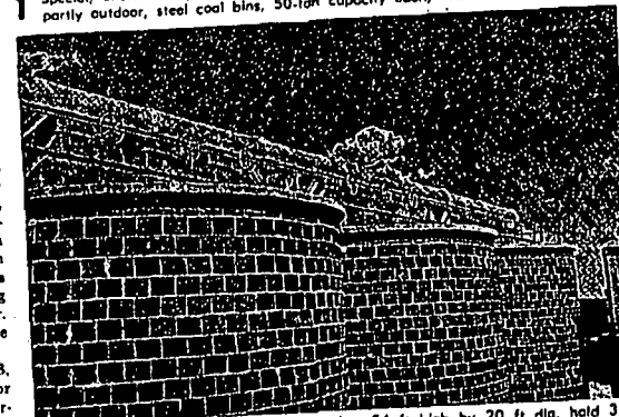
2 Reinforced, vitrified-tile coal-storage silos, 54 ft high by 20 ft dia, hold 330 tons each; are located so as to be in middle of any future plant expansion
