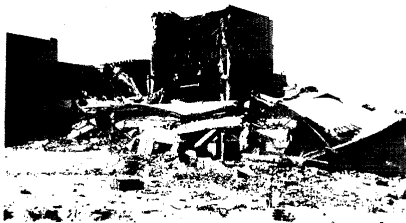
What was left of one building in Helena, Montana, after the earthquake. Modern structures and those built on rock suffered comparatively little damage.
