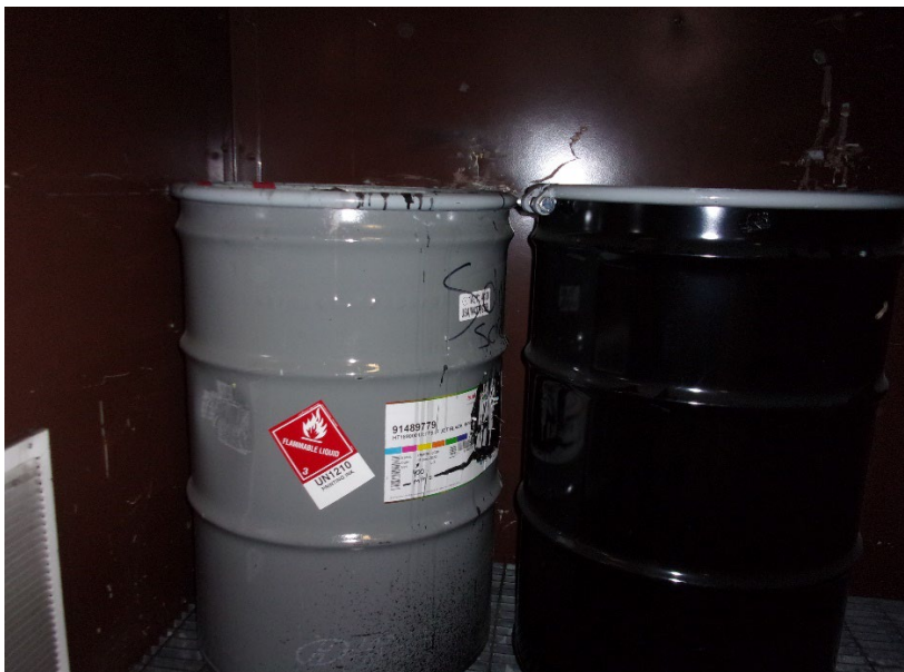
Photo -2 Inside Chemical Containment Locker - 1 55-gallon, Spent Ink Line Flush; 1-55-gallon Empty Drum
