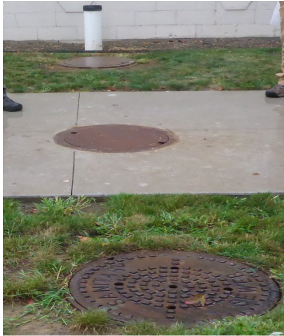
Photograph 7: Three-stage interceptor in front of the main building at JTM.
