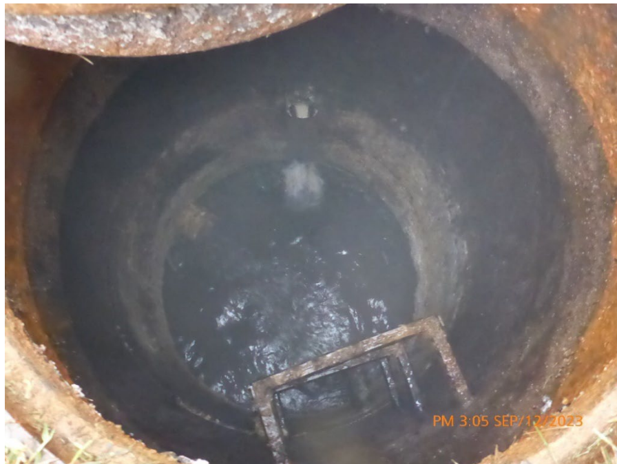
Photograph 6: Sampling manhole in front of the building at JTM.
