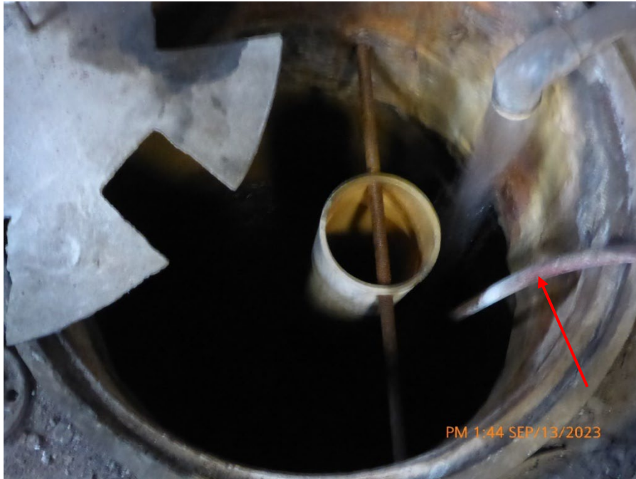
Photograph 9: Sample point at American Tinning, showing steam condensate hose (indicated by arrow) combining with regulated wastewater.
