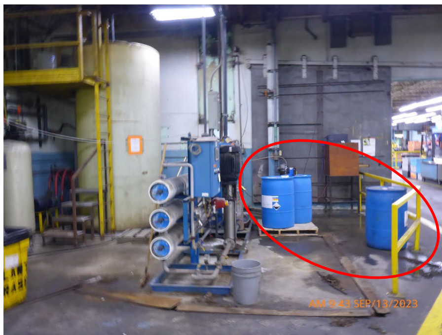
Photograph 4: Blue 55-gallon containers lacking secondary containment identified during walk-through of PHB.
