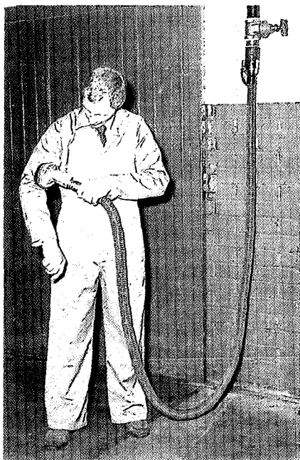
Before leaving the asbestos work area contamination on clothing should be vacuumed off
