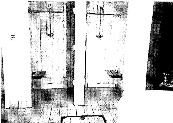
An example of good washing facilities
