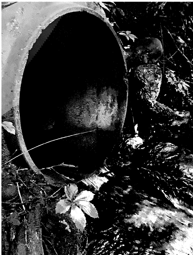
PFB15: Outfall located on the north side of 326 Clark Street discharging into Poor Farm Brook. Sample collection point indicated by a red arrow.
