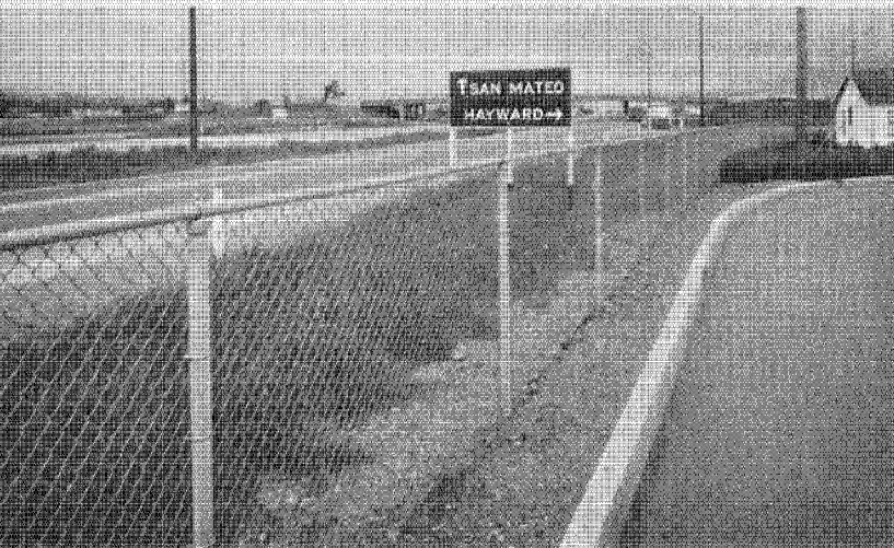
Note how "Telvar" has kept the curb area free of vegetation. Such treatment reduces maintenance, improves drainage and visibility.
