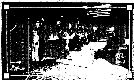
Some of our varnish fires. Skilled varnish-makers combine the melted gums and linseed oil at high temperature
