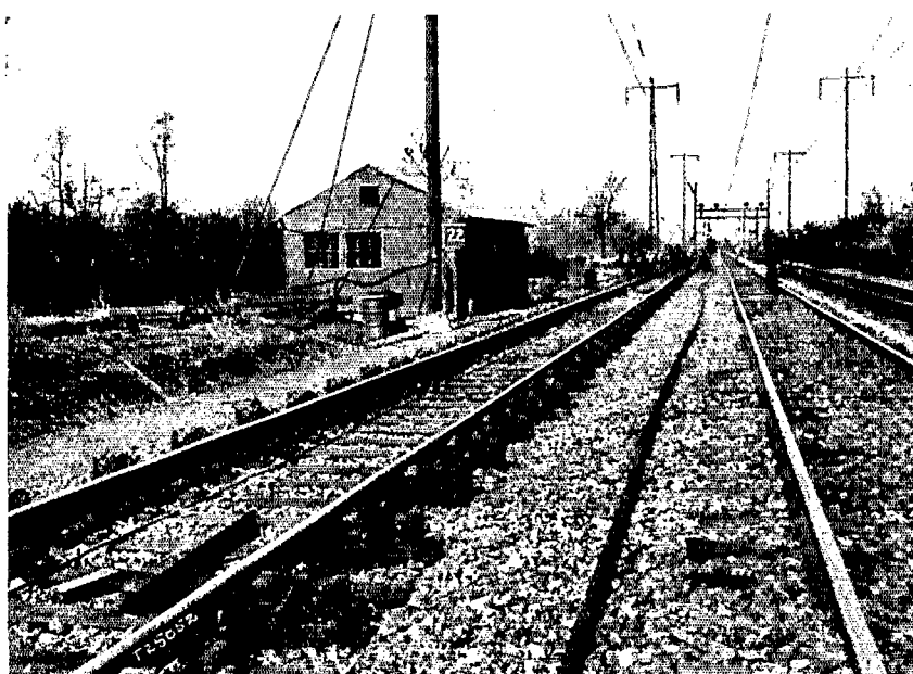
Test track at Claymont, Delaware, in normal or smooth condition, showing pressure recording devices at the ends of every alternate tie. The ties, both with and without recording apparatus, are of steel.
