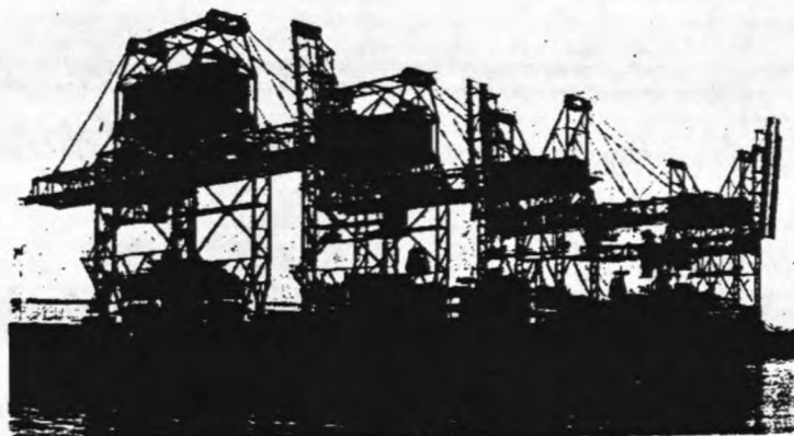
The Dravo Elliott-driven unloader is shown at left in the photograph reproduced below. Conveyor belts carry the ore from the hoppers of all four unloaders to the waiting weigh house and gondola cars for immediate movement to the nation's steel mills.
