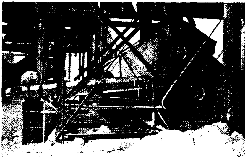
FIGURE 2. Fiber recovery process using willower and vibrating screens.
