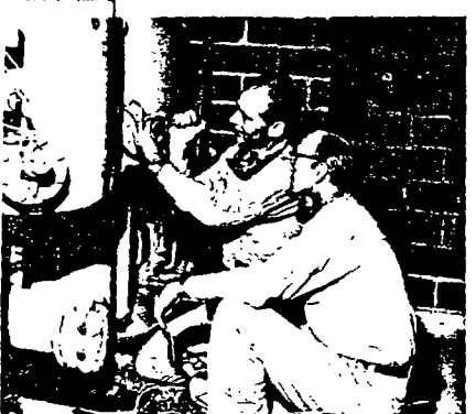
Ivan Lee, (left) Cecil Long rewired rectifier tanks in the rectifier substation.
