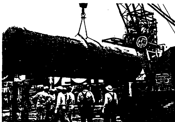
Construction work is progressing rapidly on the new methyl chloride unit. This photograph, taken May 1, shows one of the large tanks being lowered to the concrete foundation. Workers stand by to see that the tank is in correct position for the attachment of pipes and fittings. Construction is expected to be completed on the new unit this summer.
