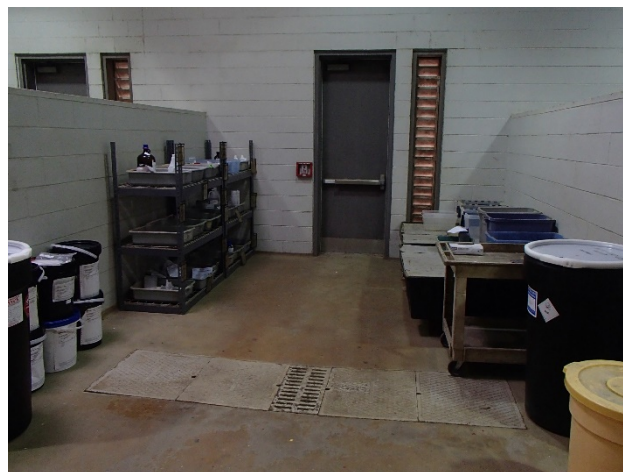
Photo 4: Cell 214-O Organic waste storage.
