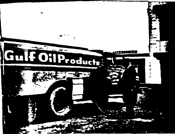
A 14-unit tank truck fleet brings gasoline from Putnam Brothers bulk plants to the company's 70 service stations.
