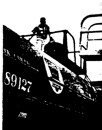
Two "firsts" at new vinyl chloride plant: Top, an operator opens valve to start production. Above, initial tank car of liquid chemical is "buttoned up" for shipment.
