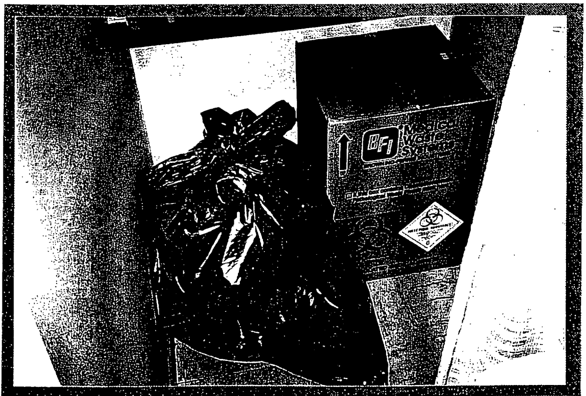
Medical waste storage area on 15th floor.
