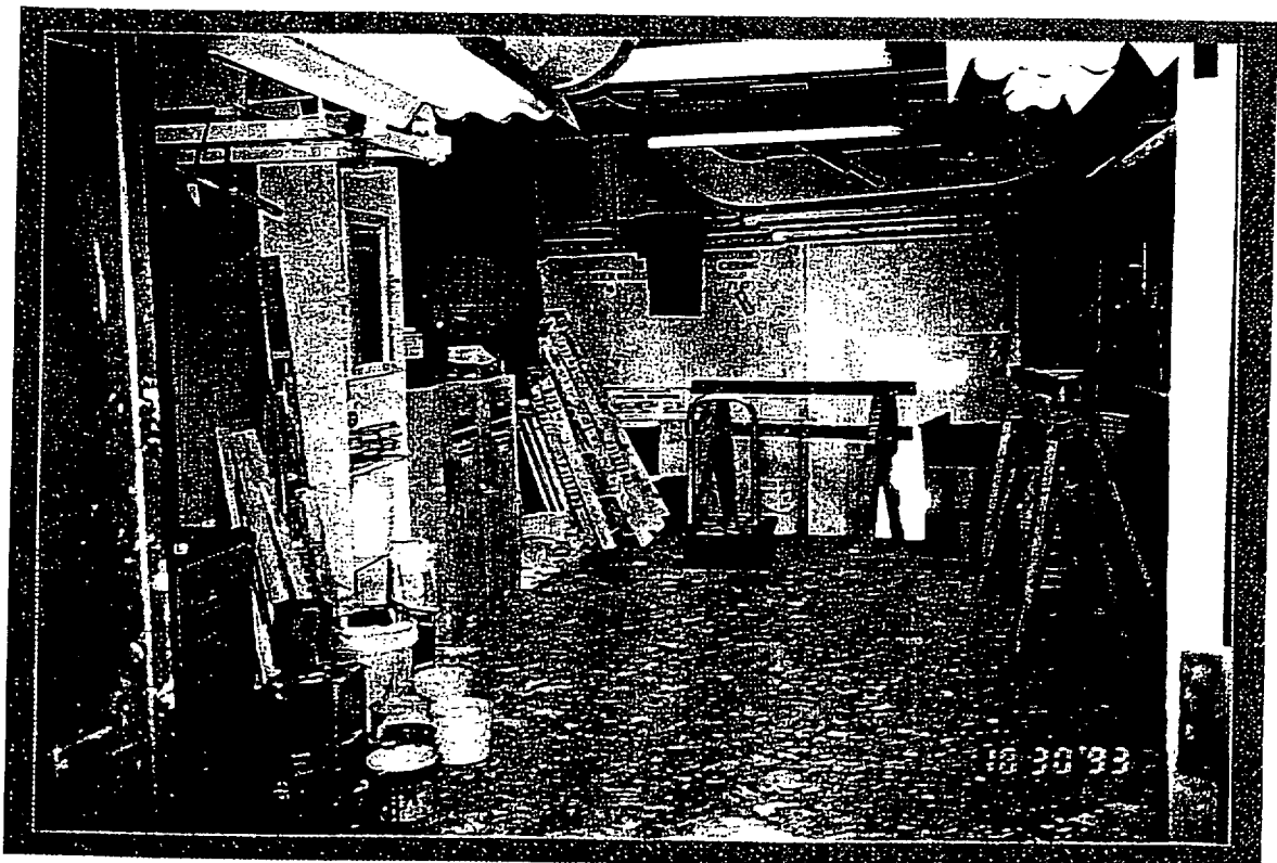
Paint spray shop in basement, room B-28A.
