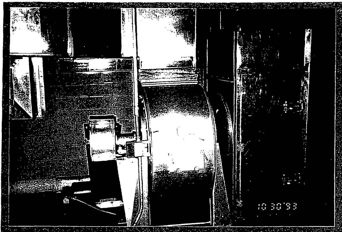
Exhaust system for medical floor air.
