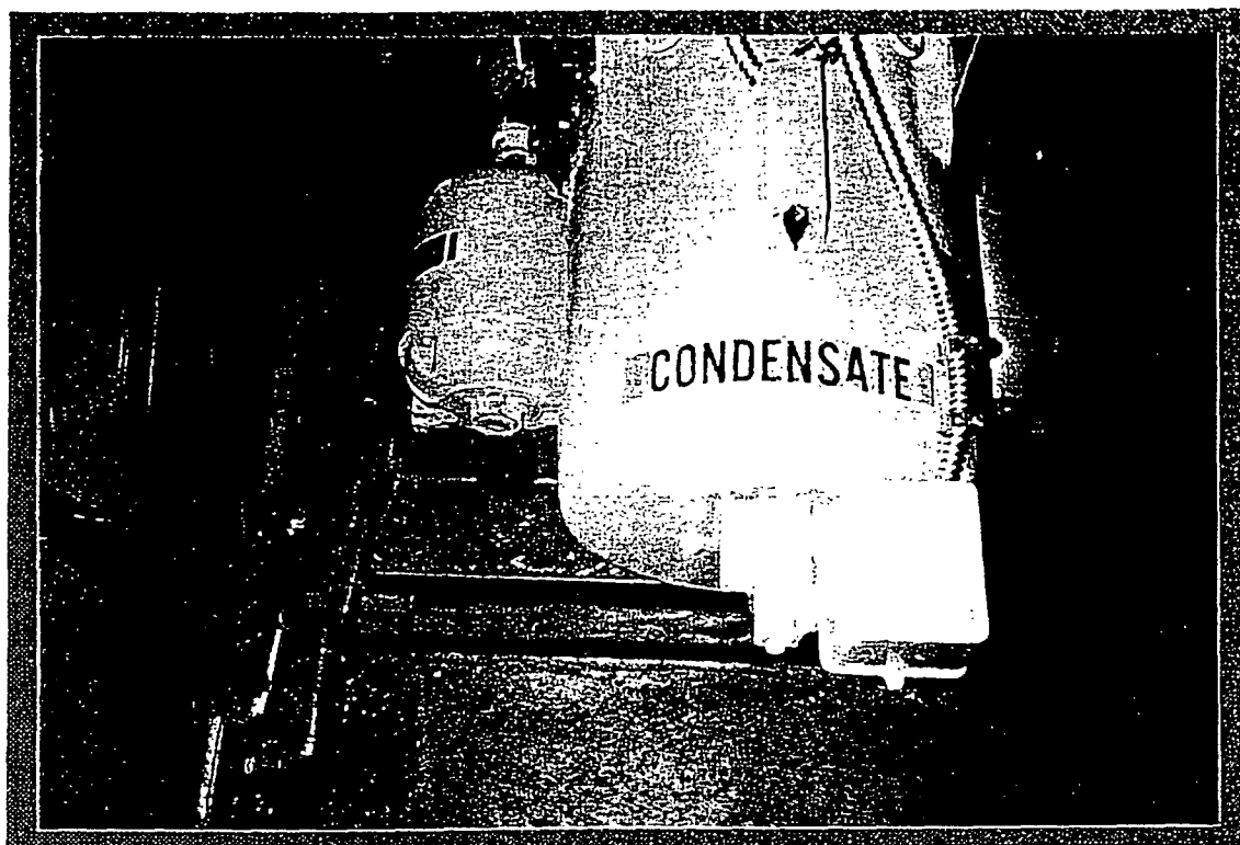
Condensate pump located in sump in floor of subbasement engine room.
