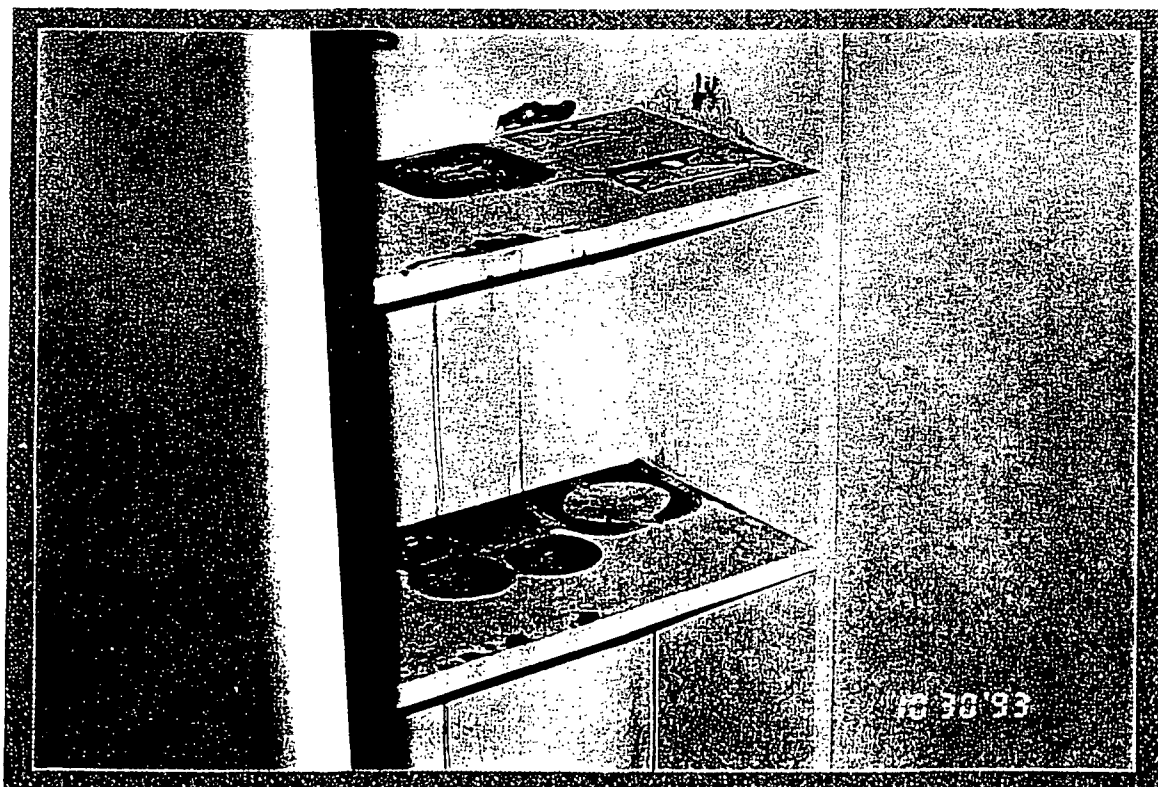
Stained shelves in former basement darkroom, room B-51.
