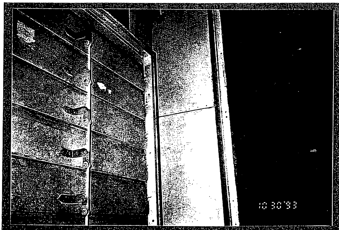
Intake chamber for outside makeup air in 14th floor primary air handling crossovers (outermost chamber).
