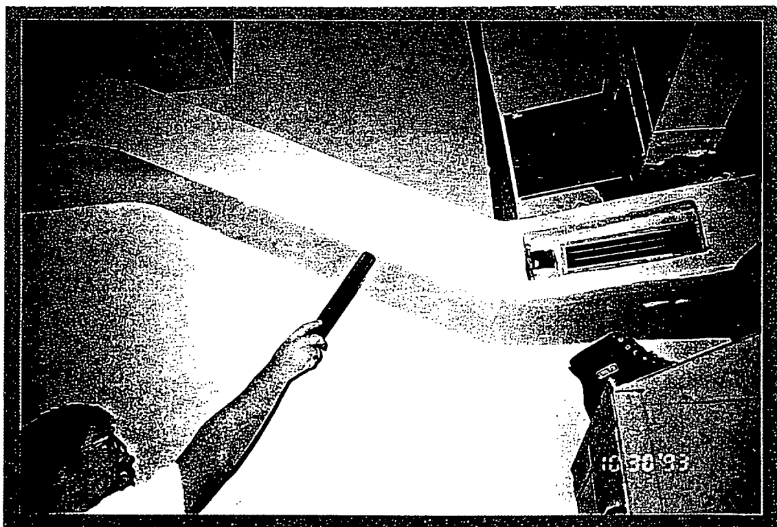
Breaching over ductwork insulation in subbasement locker room.
