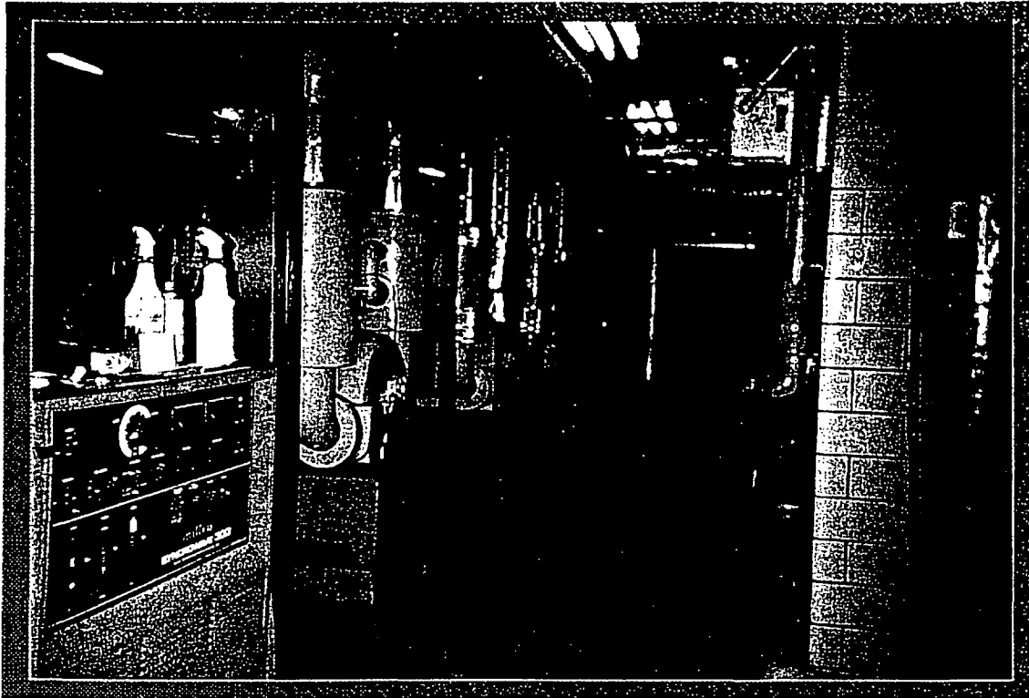
Hot water pump area in subbasement engine room.
