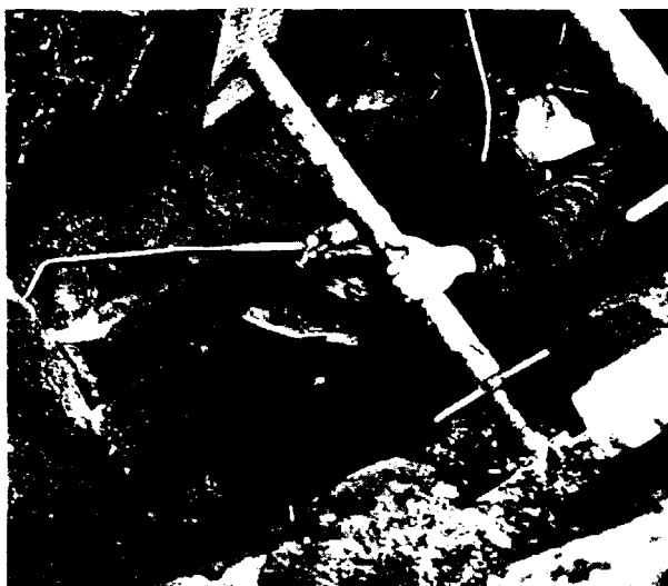
The use of a torch facilitates the removal of calking lead from joints. The lead may then be reused with perfect results, as in Springfield, Ill.
