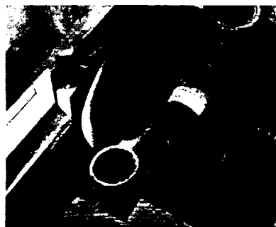
Lead water closet and vent connection in the Madison Park Housing Project at Seattle, Wash.
