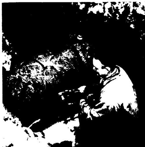
Tapping the water main at Stamford, Conn., and the Seal of Approval lead service which was insisted upon by the owner
