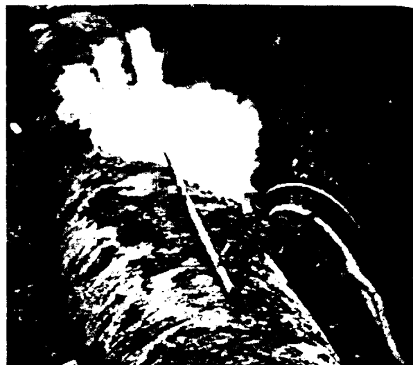
The use of a torch facilitates the removal of calking lead from joints. The lead may then be reused with perfect results, as in Springfield, Ill.
