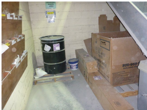
Photo 19: Universal waste accumulation and storage area in the Holcim Maintenance Area.
