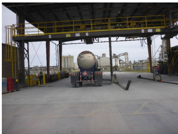
Photo 5: Tanker truck unloading bays in Area 6100.
