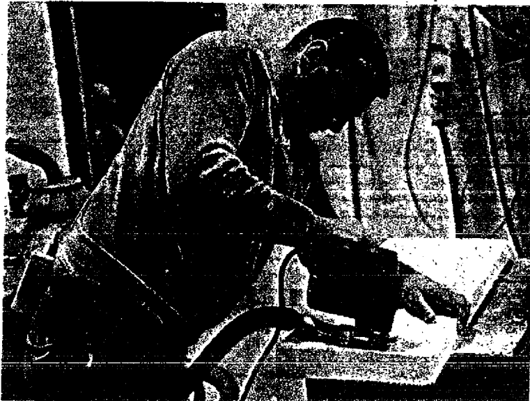
Charles Collins, President of Local 30 of the Asbestos Workers Union, cutting calcium silicate block during the powered hand-saw trials at the Hoffman Air Systems plant in Syracuse, New York.
