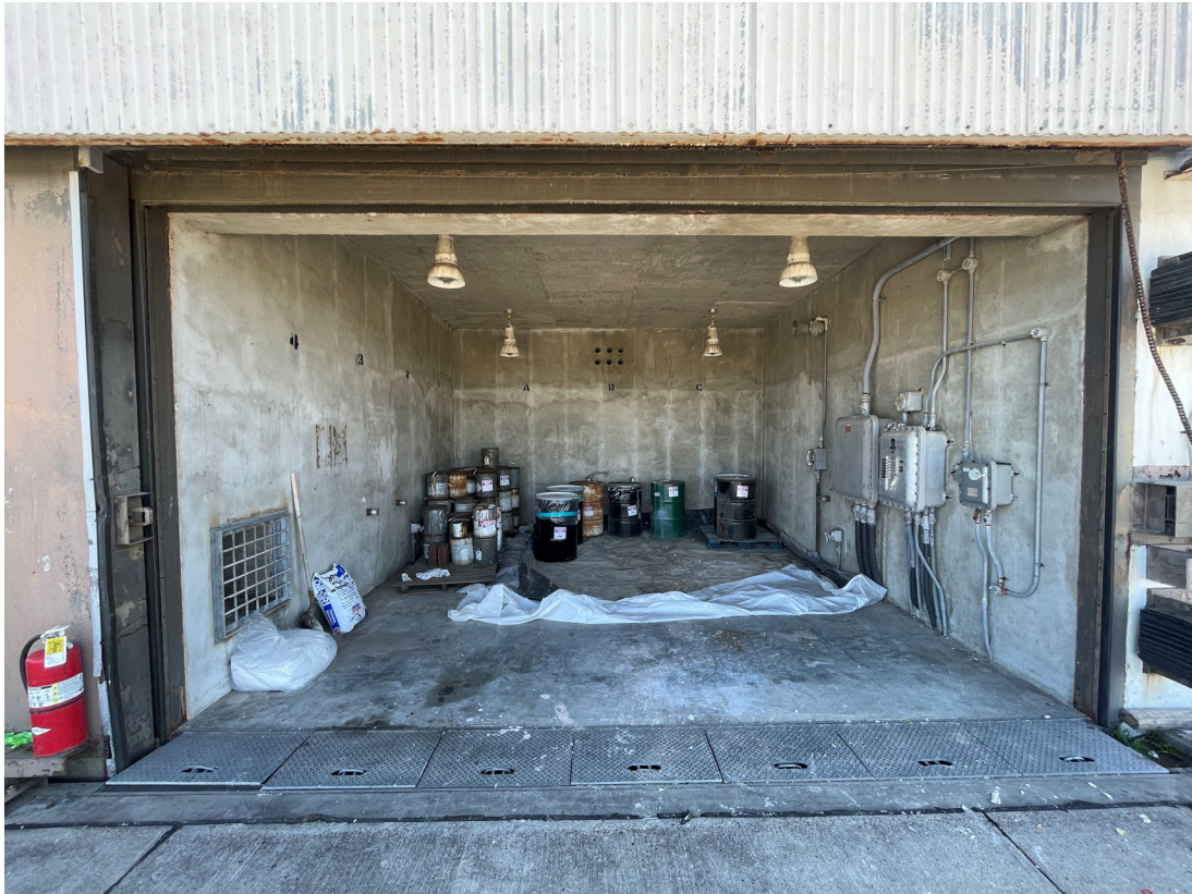
Figure 2: Universal waste paint & paint related waste storage area.
