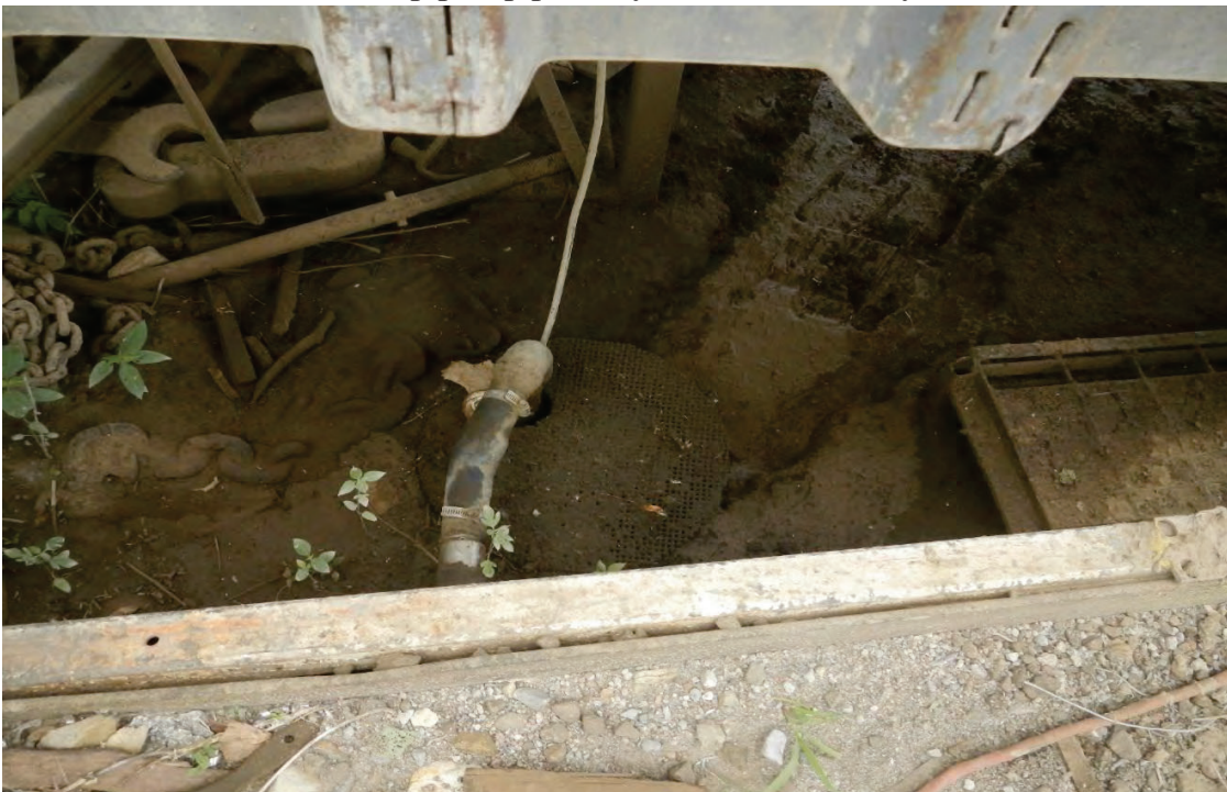
Photo 21, Sump pump possibly leadn the sanitary sewers
