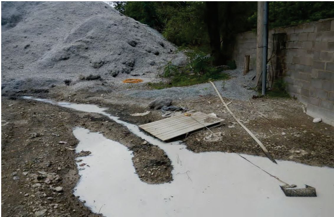
Photo 6 Murky water caused by stormwater runoff off the aluminum pile
