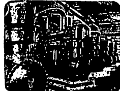
Six of the Nine Big Frick 4-Cyl. Ammonia Compressors
