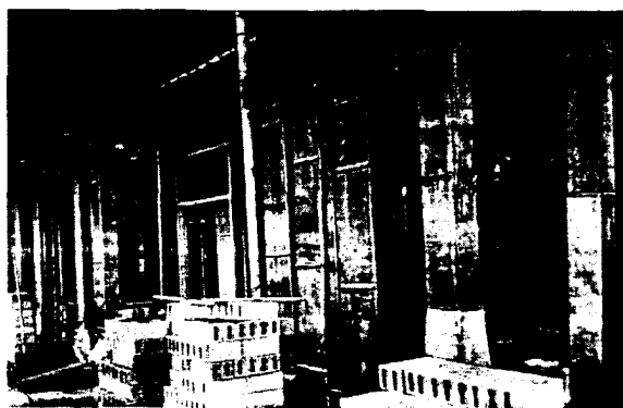
Some of the lead risers in the chemical laboratory ventilating system, giving an idea of the vast extent of the installation.
