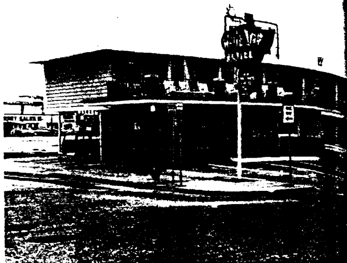
Lead-cured rubber solved the roofing problem at Wildwood.
