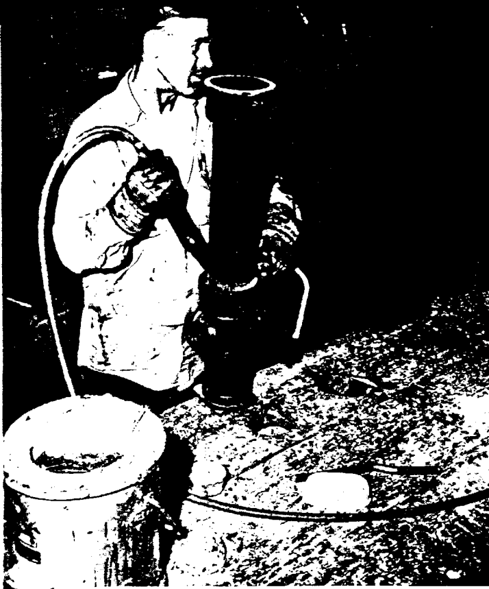
Advantages of shop prefabrication show up as this plumber uses a pneumatic tool to calk oakum into a cast iron pipe joint.
